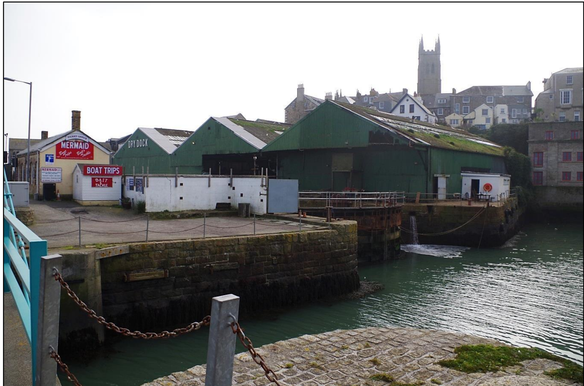
Fig 17 The former Holmans Dry Dock (Sites 23 and 25) (now owned by Penzance Dry Dock Ltd) from Ross Bridge (Site 20).
