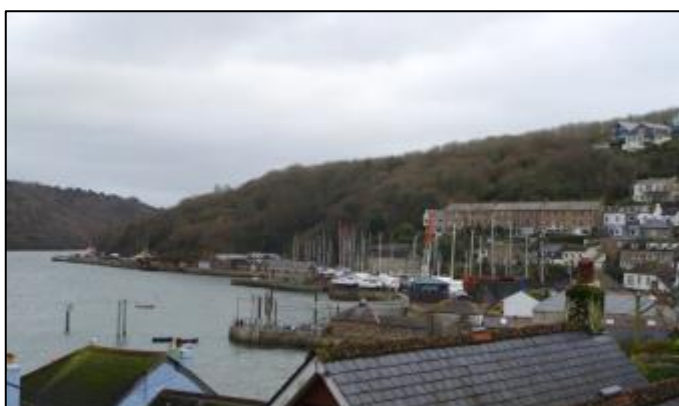
Fig 11 Late 19 th and early 20 th century shipyards extend along the shoreline to the north of Polruan, infilling between earlier quays and fish cellars.
