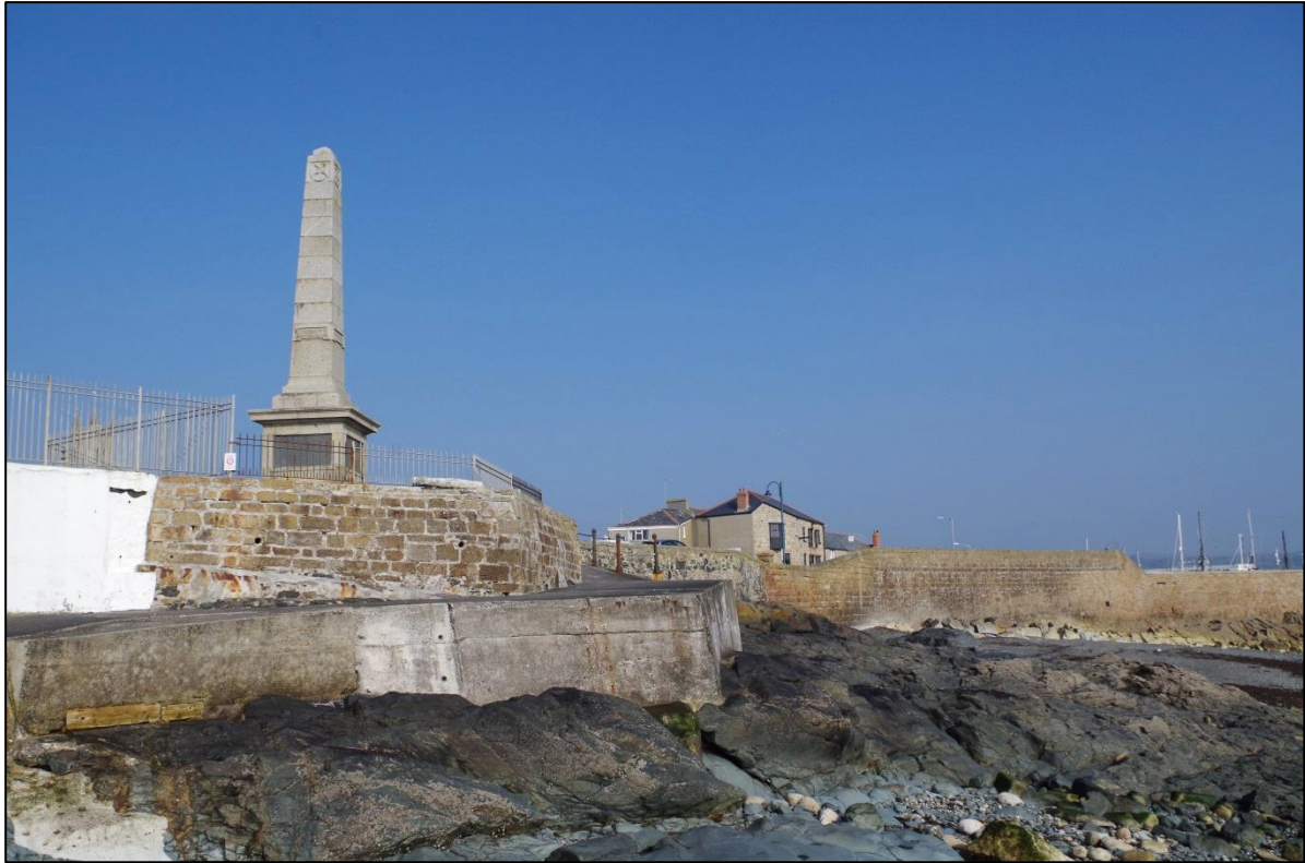
Fig 21 the base of the 18 th century battery (Site 6) from Battery Rocks, now the site of a WWI war memorial (Site 7).
