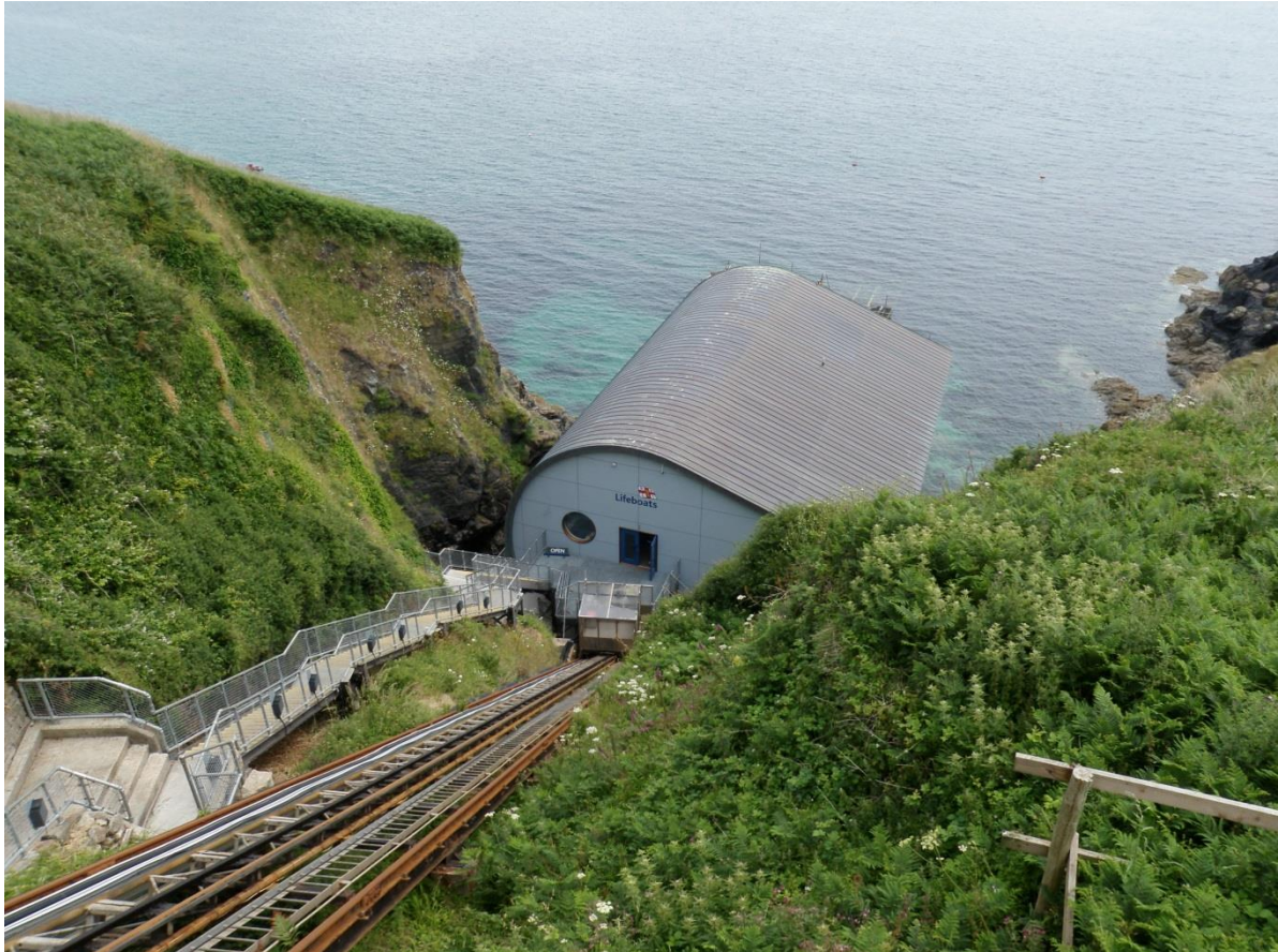
Fig 28 The modern build of the lifeboat station at Kilcobben Cove with its curved roofline presents an iconic modern building in its own right (Photograph: CAU).
