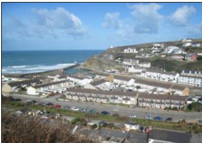
Fig 10 The former coal yards and industrial quaysides at Portreath are now wholly redeveloped for modern housing.
