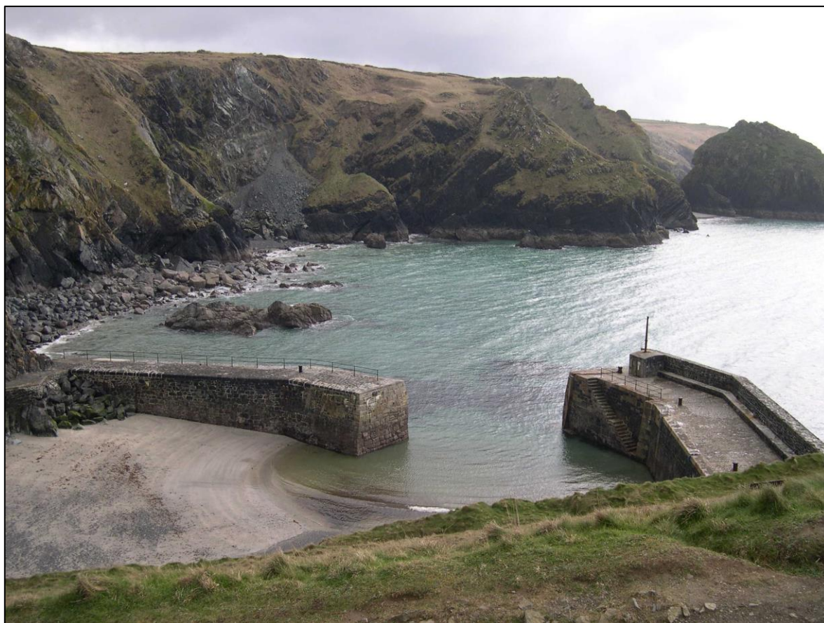
Fig 25 Mullion Harbour in June 2015 (Photograph: CAU).
