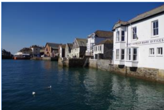
Fig 7 The historic quays extending north from Town Quay in Fowey illustrate the growth of the harbour during the medieval and post-medieval periods. The granite jetties and steps reflect different phases of construction and still survive in excellent condition.
