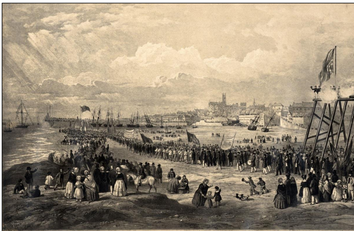
Fig 3 Setting the foundation stone for the New Pier (Albert Pier). A photograph of an engraving of July 7 th 1845. Delineator - FC Stockdale. Lithographer - Thomas Picken. (Penlee House Gallery and Museum PEZPH: 1989.554).
