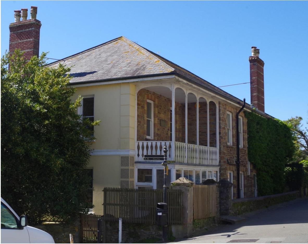
Fig 11 'Q's house in Fowey (Photograph: CAU).
