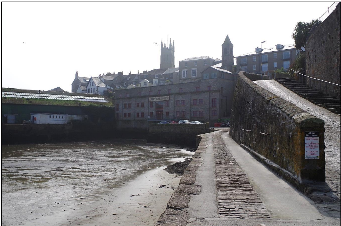
Fig 16 Looking west across Abbey Basin (Site 55) towards Abbey Warehouse (Site 37). The sloping path on the right is probably one of the post medieval slips (Site 39) onto the former foreshore.
