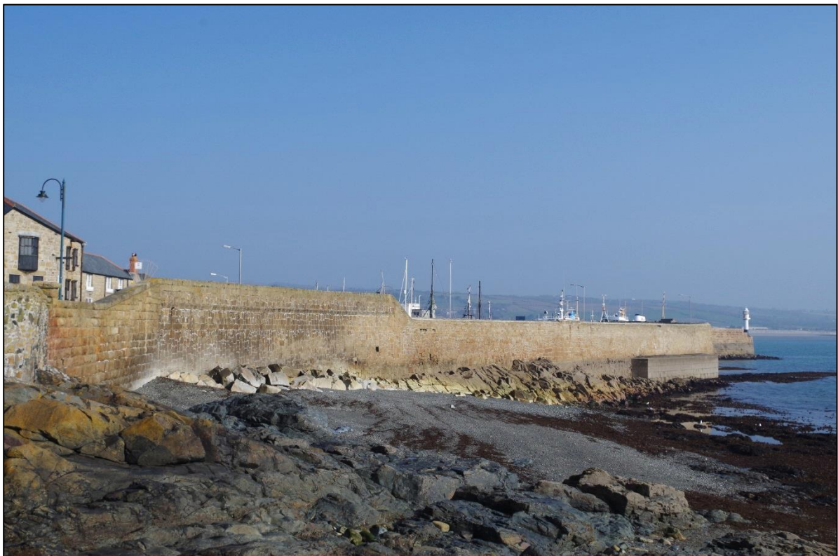
Fig 20 The defensive sea wall on the south side of South Pier (Sites 8 and 9); the construction clearly shows several phases of rebuilding and repair.
