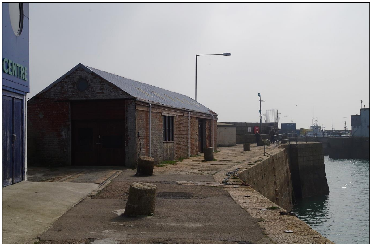
Fig 18 The south end of Albert Pier (Site 45); a former railway shed (site 46) survives along with a section of railway line (Site 51). Granite mooring posts (Site 50) line the quay and some of the historic quay surface and walling can also be seen.
