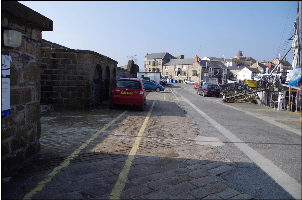
Fig 13 Looking west along South Pier (Site 10) towards the Dolphin Tavern (Site 33). The earliest medieval quay structure may be preserved within later rebuilds, some of which are 18th century in date.
