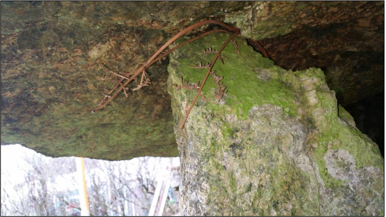
Figure 8: Point of contact between the supporting stone and the underside of the covering slab.
