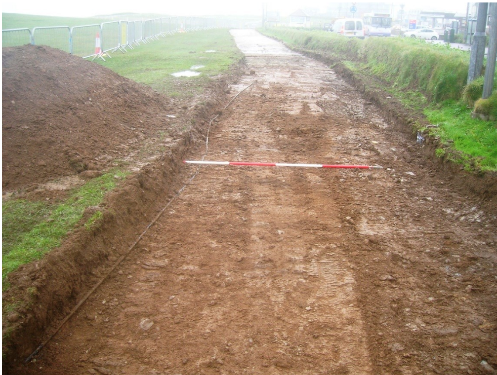
Figure 16. Disused BT cable exposed at southwestern end of cycle track at SW 81928 62075.
