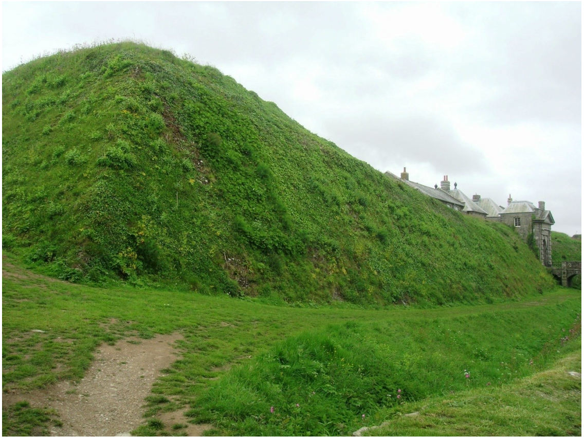
Figure 7. External face of Smithwick's Bastion showing the nature of the slope.
