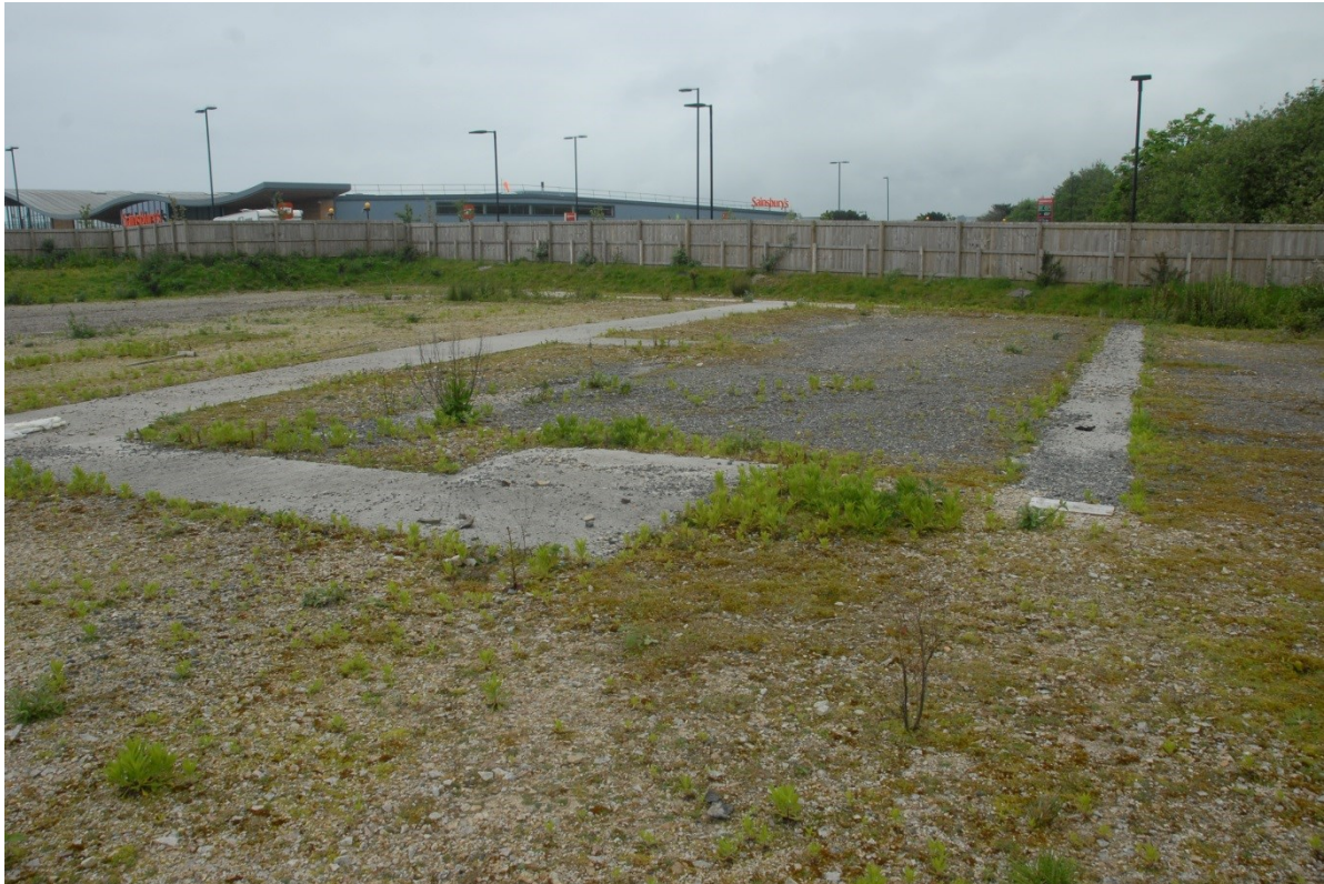
Fig 19. The concrete strip foundations at the western end of the project area.
