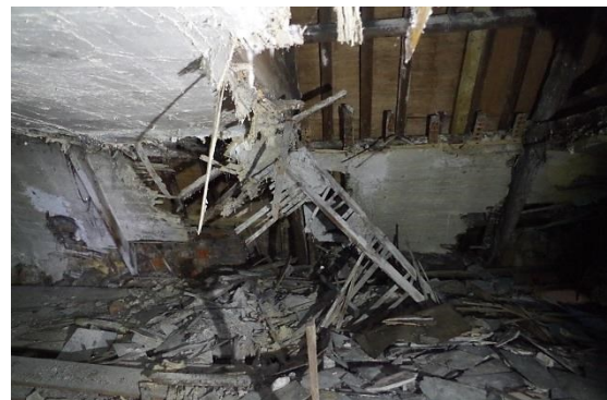
Fig 53 Room 27 collapsed lath and plaster ceiling looking north-west.
