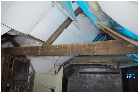
Fig 49 Room 25 sawn off truss looking north-east.
