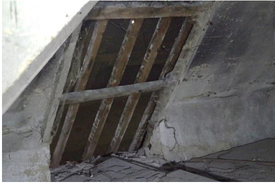
Fig 55 Room 27 blocked dormer window in rear, south-west wall.
