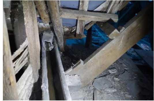
Fig 51 Room 26 Lead launder taking rain water from the diamond valley in the roof out to the rear wall at eaves level.
