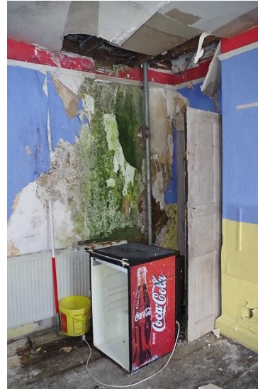
Fig 32 Room 14 water damage in south-west corner.
