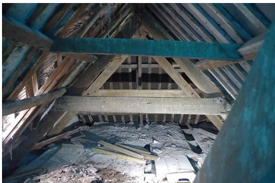
Fig 50 Room 26 pegged collar trusses looking south-west.
