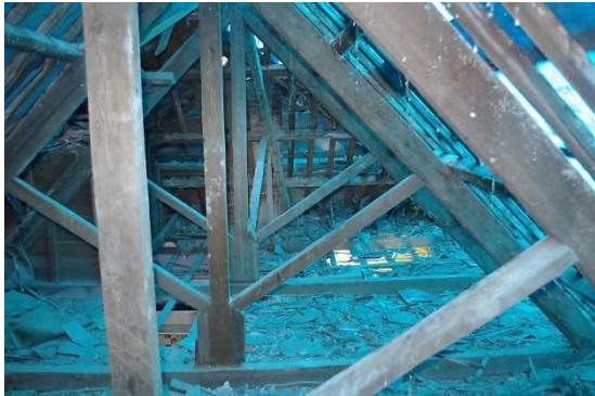
Fig 56 Room 28 kingpost trusses looking north-west showing former hip structure at north-west end of house.
