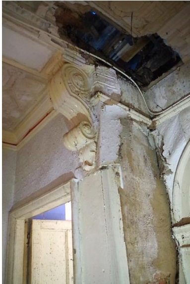
Fig 35 Room 16 detail of 18 th century corbel and damaged cornice.
