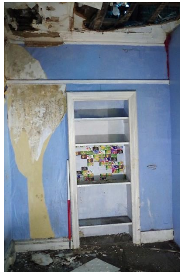
Fig 39 Room 20 showing 18 th century recessed cupboard in north-west wall.
