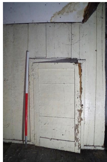
Fig 46 Room 25 cupboard in north-east wall. Door has HL hinges.
