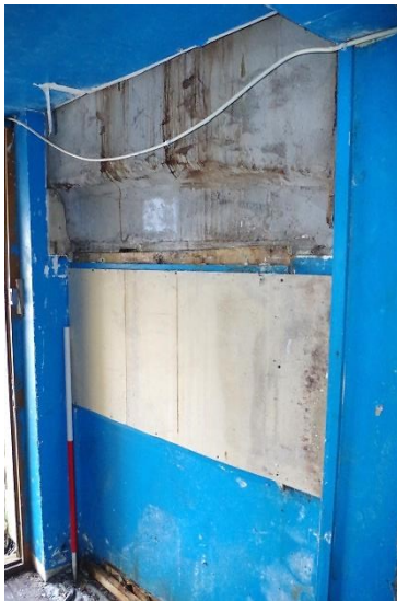
Fig 25 Room 11 looking north showing blocked window in rear wall of house.
