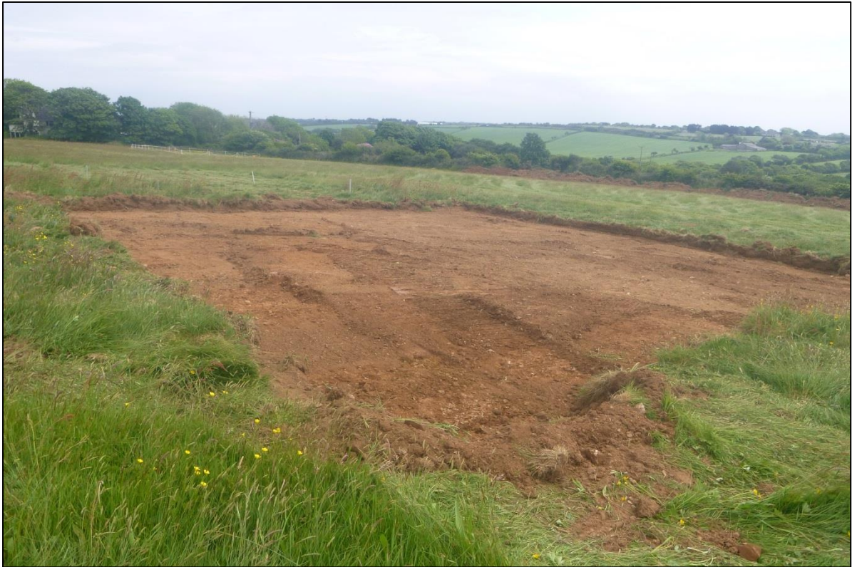
Figure 5: Post excavation view of crane pad/laydown area looking south east.
