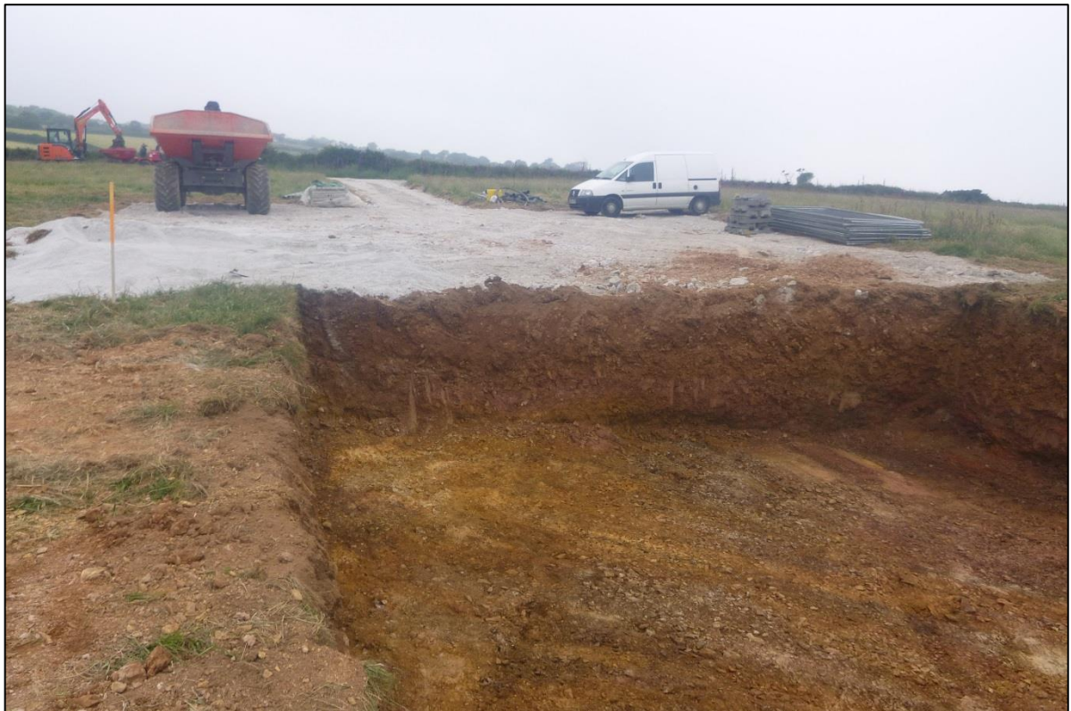
Figure 6: Post excavation view of turbine foundation pit looking west.
