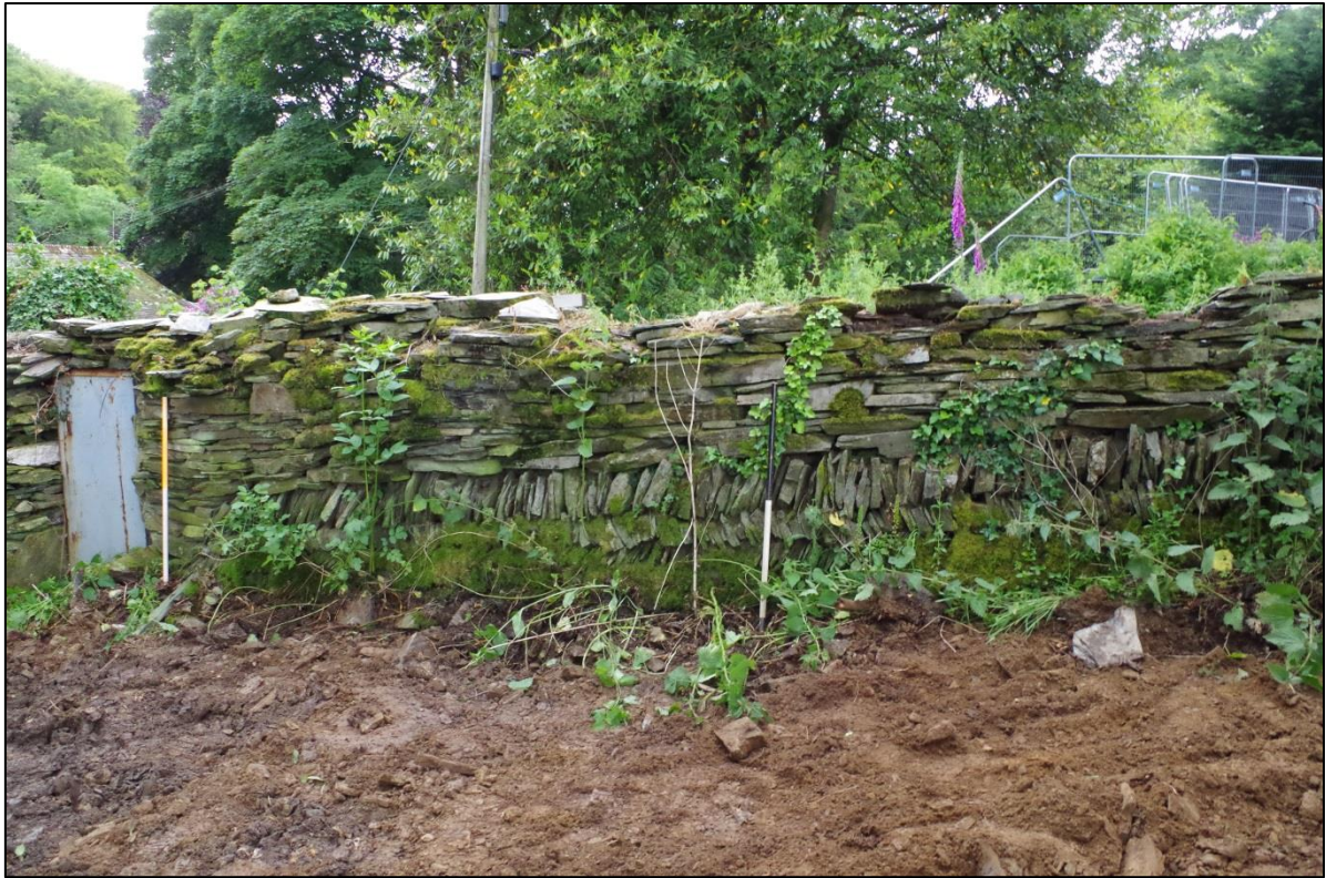
Figure 5: View of field wall looking west, 1m scale.
