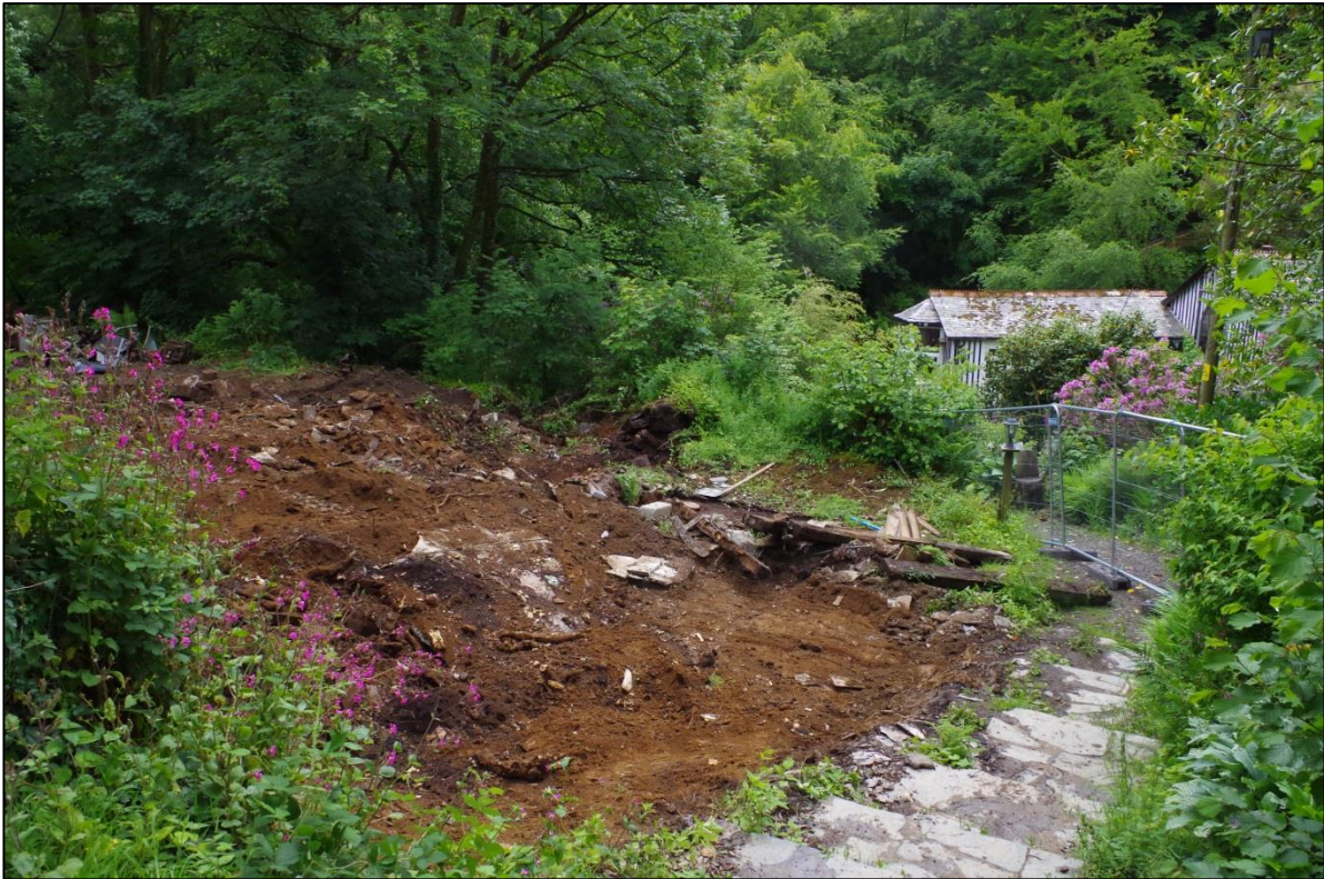
Figure 8: View of Area B post clearance.
