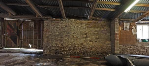
Fig 71: Northern shed NW wall doorway and window
