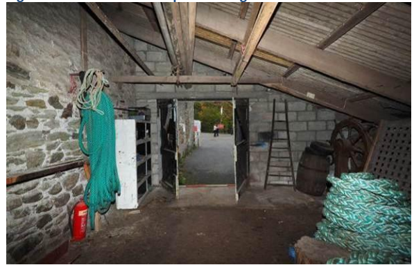
Fig 48: Southern shed NE end
