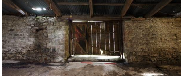
Fig 70: Northern shed NW wall altered doorway
