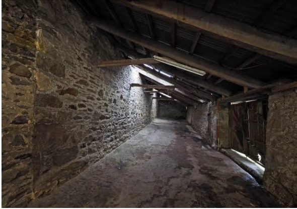
Fig 51: Northern shed from NE
