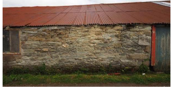
Fig 22: NW wall of northern shed left of centre
