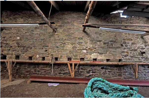
Fig 47: Southern shed NW spine wall towards right
