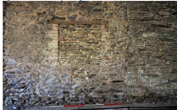
Fig 54: Northern shed SE wall: inserted then blocked window
