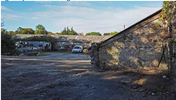
Fig 31: Later wall within northern shed, now the end wall
