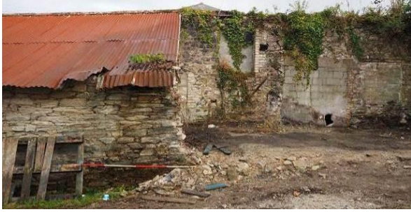
Fig 27: Truncated NW wall of northern shed + spine wall, right
