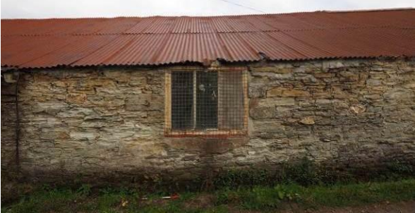
Fig 21: NW wall of northern shed towards the left
