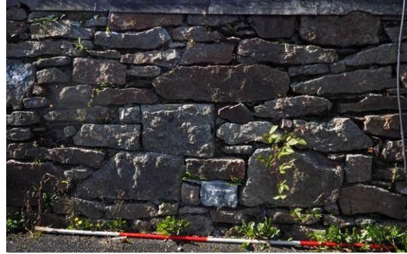
Fig 18: Detail of SE wall of southern shed
