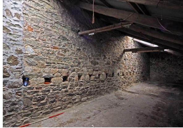
Fig 52: Northern shed pressing-beam sockets from north
