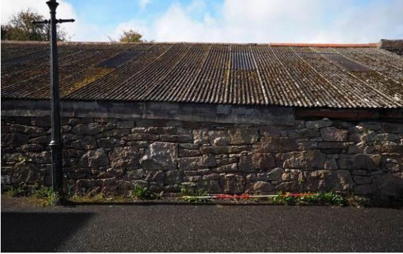
Fig 17: Representative length of SE wall of southern shed
