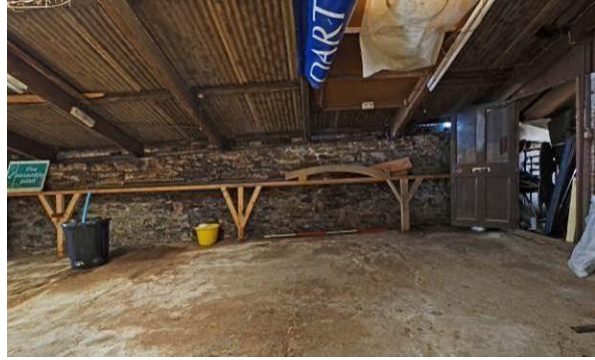
Fig 36: Southern shed SE wall centre
