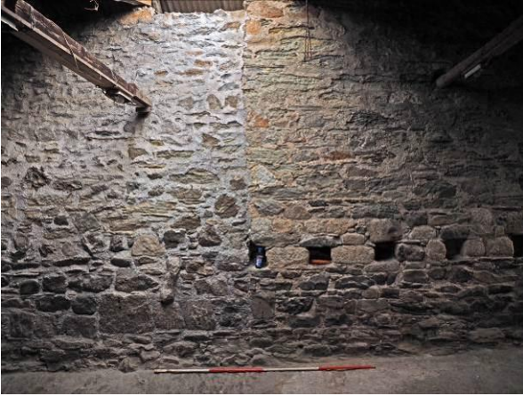
Fig 59: Northern shed SE wall junction with beam sockets
