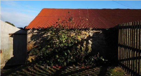
Fig 19: NE end of NW wall northern shed from NW
