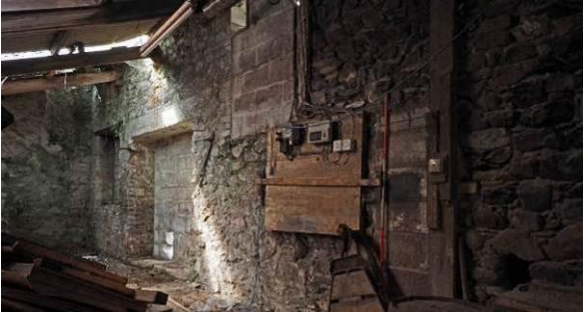
Fig 43: Southern shed NW spine wall left-hand end from east
