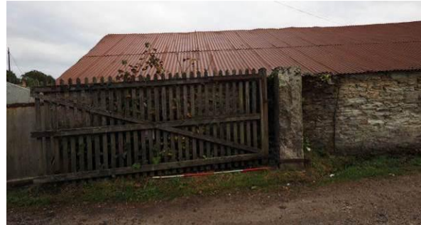
Fig 20: NE end of NW wall of northern shed
