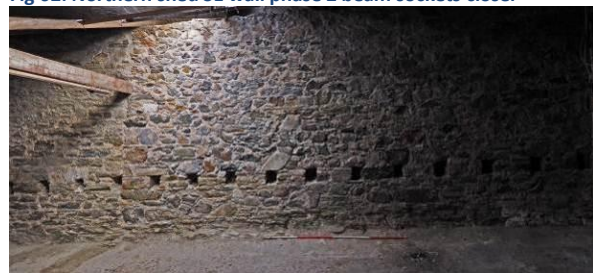
Fig 64: Northern shed SE wall phase 1 beam sockets
