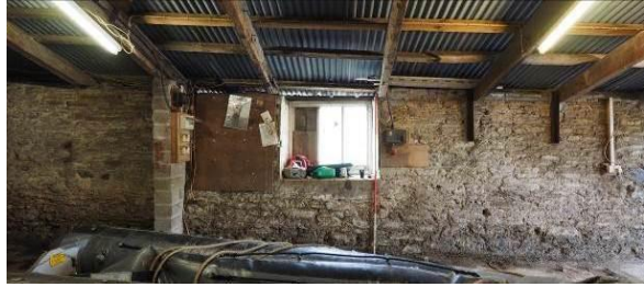
Fig 72: Northern shed NW wall centred on window
