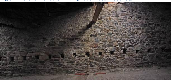
Fig 63: Northern shed SE wall phases 2 and 1 beam sockets
