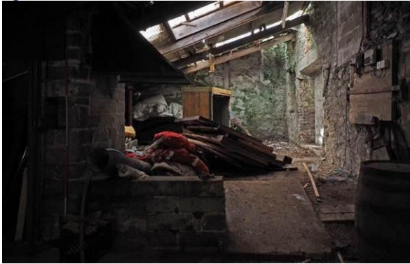
Fig 37: Southern shed SW end; early-mid C20 forge on left
