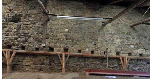
Fig 46: Southern shed NW spine wall right of centre
