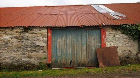
Fig 23: NW wall of northern shed: widened doorway left of centre
