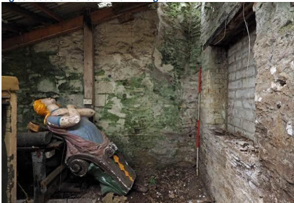
Fig 41 Southern shed SW wall, right
