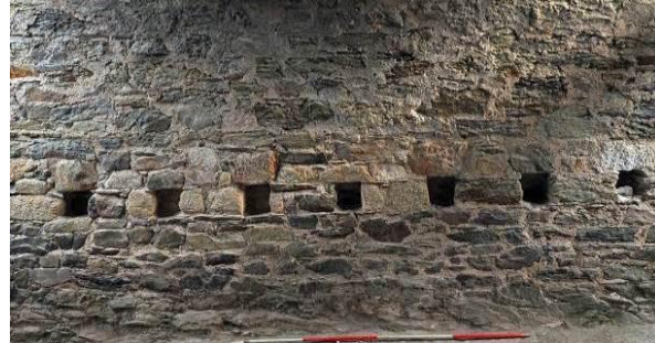
Fig 62: Northern shed SE wall phase 2 beam sockets closer
