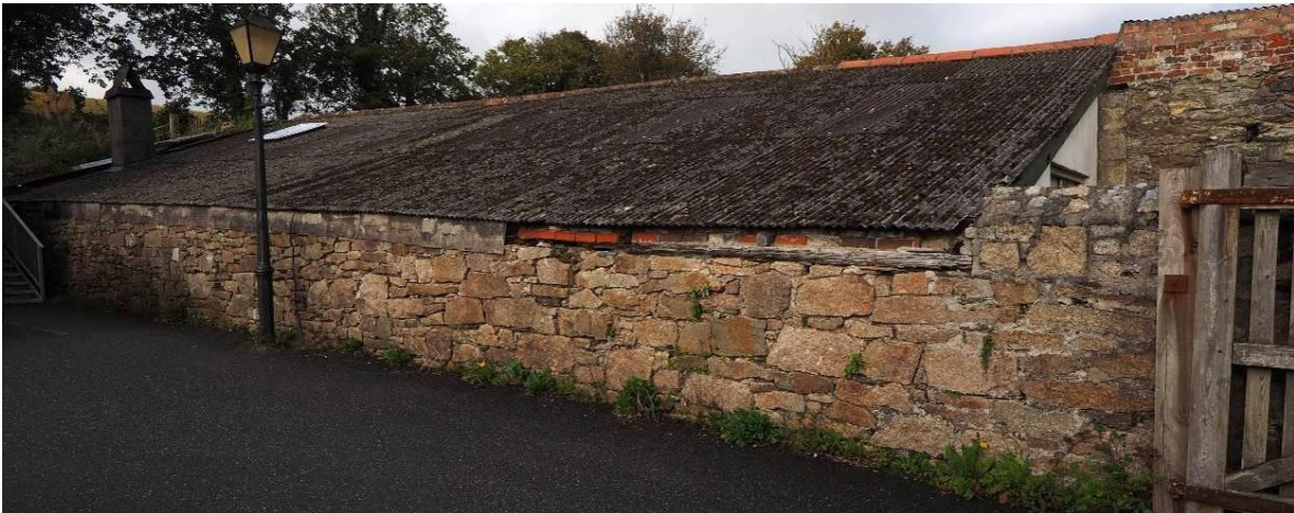
Fig 8: SE wall from east
