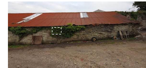
Fig 25: : NW wall of northern shed, right with approximate location of hidden blocked window opening within dashed line
