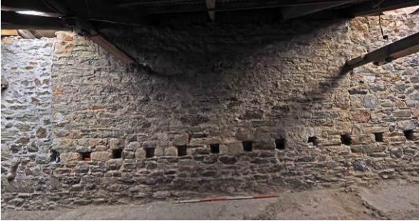
Fig 61: Northern shed SE wall phase 2 beam sockets
