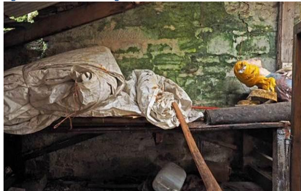
Fig 40: : Southern shed SW wall, left
