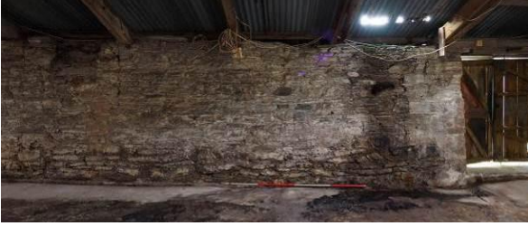
Fig 69: Northern shed NW wall left of centre
