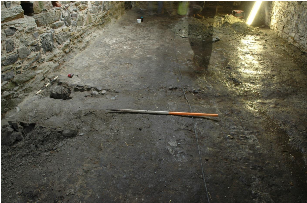
Fig 10 Shed 1: surface drainage gully (301) looking south-west
