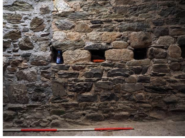
Fig 60: Northern shed SE wall junction with beam sockets
