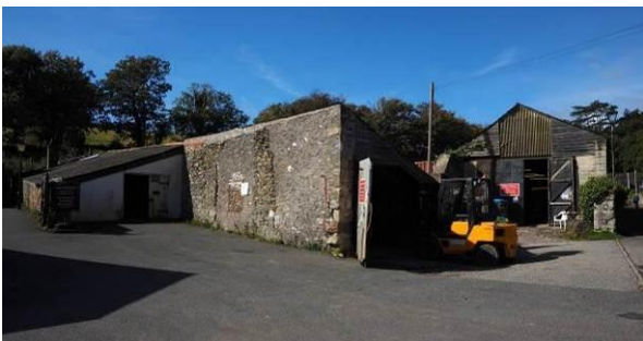
Fig 13: Sheds and context from east
