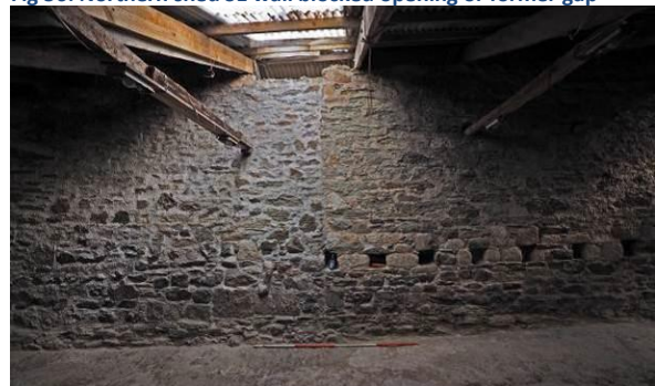
Fig 58: Northern shed SE wall junction with beam sockets
