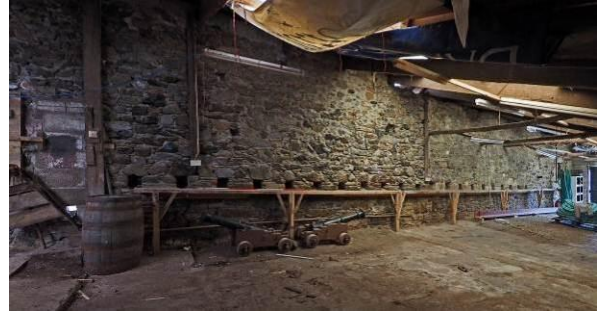
Fig 44: Southern shed pressing-beam sockets from south
