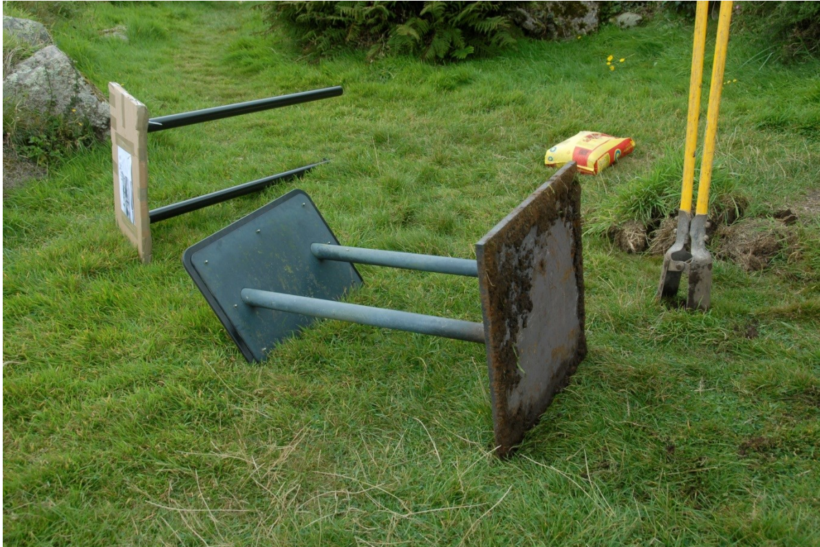
Fig 24. The original Interpretation Panel 2 at Carn Euny following its removal, showing the heavy steel plate which had anchored it into the ground.
