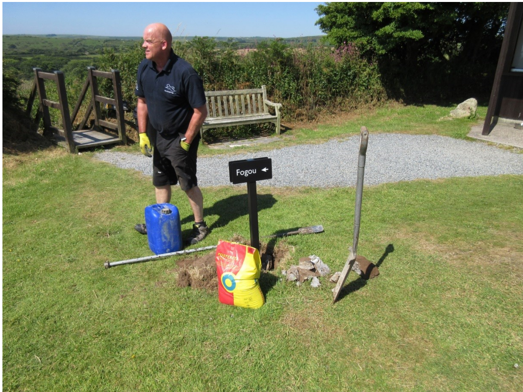
Fig 12. The replacement Operational Sign installed adjacent to the Chysauster ticket hut.
