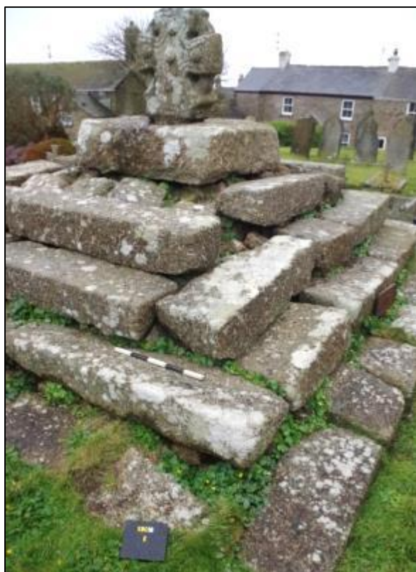
Fig 13 North east corner (JG).
