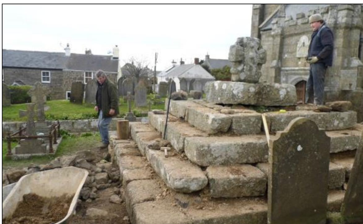
Fig 31 Conservation work in progress: the use of rab (local orangey-brown granitic subsoil) to level the stones can be seen in this picture (in the stonework joints and in the wheelbarrow) (AGL).
