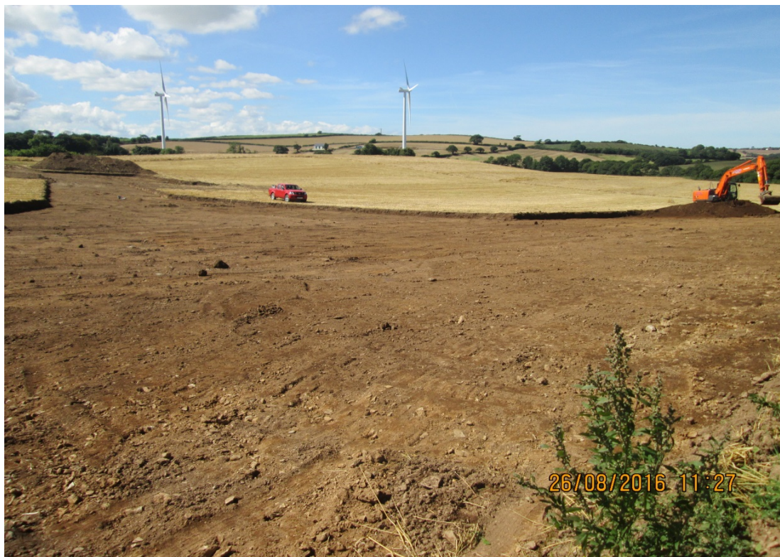
Figure 4: The eastern corner of the stripped area looking west. ©CAU
