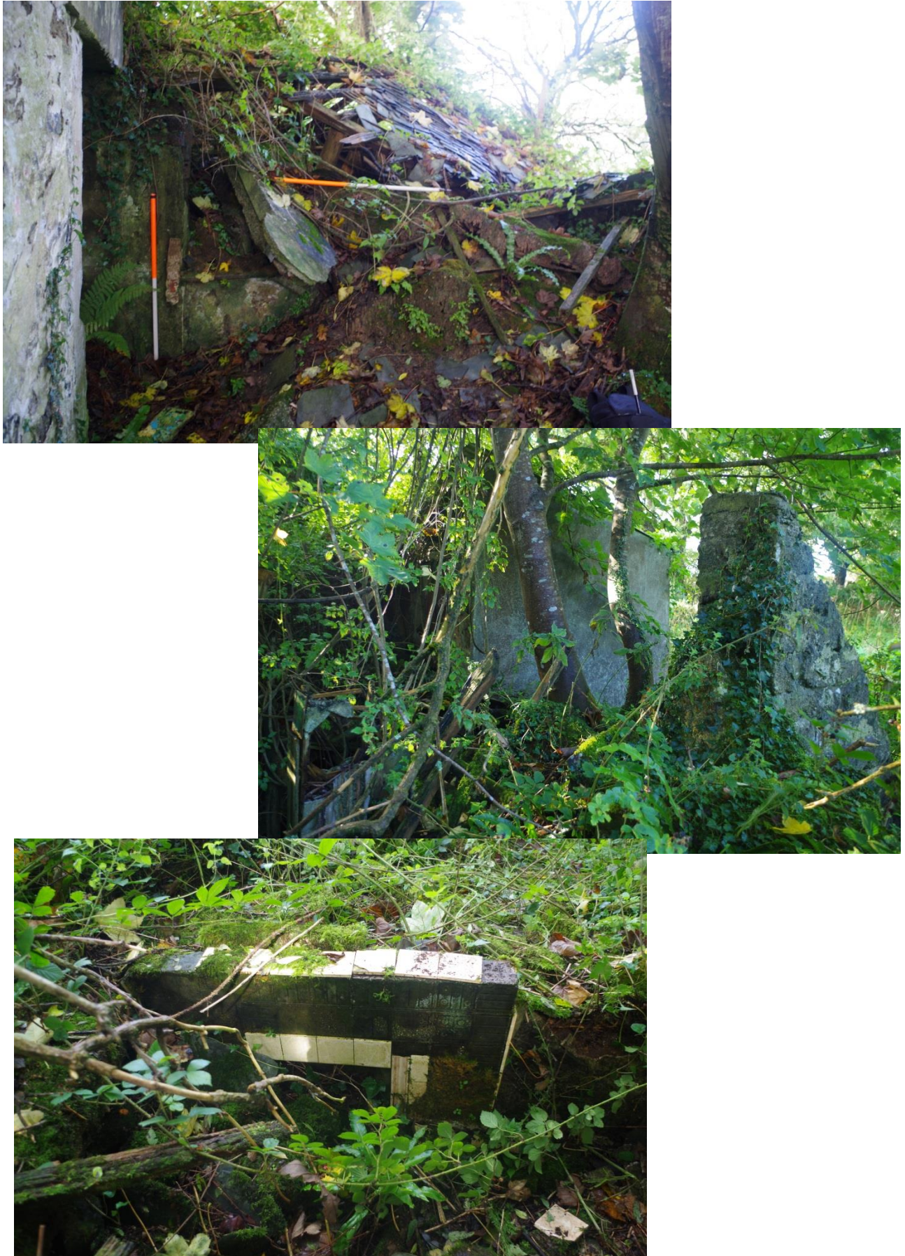
Fig 8 Higher Bochym, top – looking west at north-western corner of building A; middle - looking south along external western wall of building a showing buttress?; bottom – looking north at internal northern gable end of building A showing remnant fire place with ceramic cream tiles and fallen chimney stack beyond.
