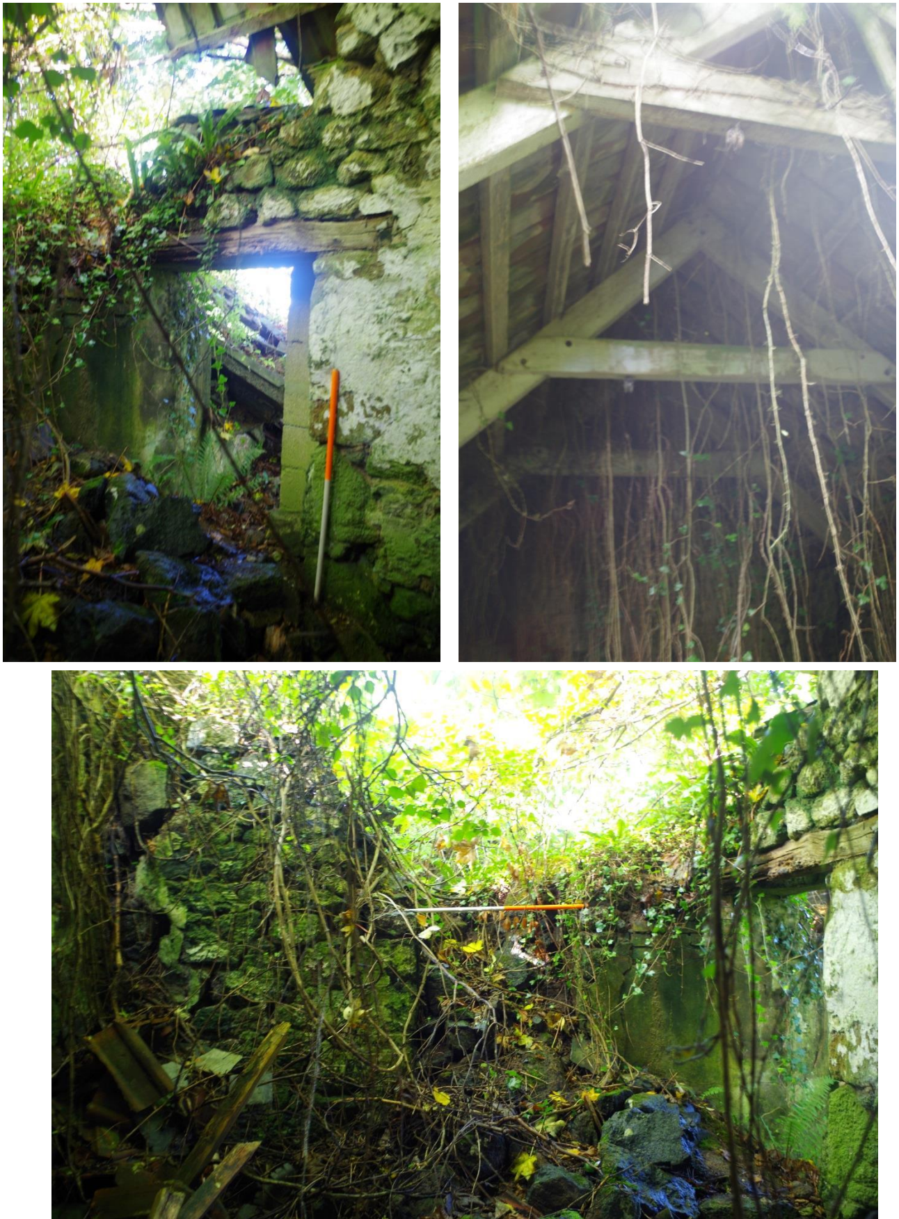
Fig 6 Higher Bochym, top left – internal north-west corner of building B showing doorway and building A outside; top right – remnant roofing with two surviving rope pulleys; bottom – looking west inside building B showing doorway blocked with collapsed building A.
