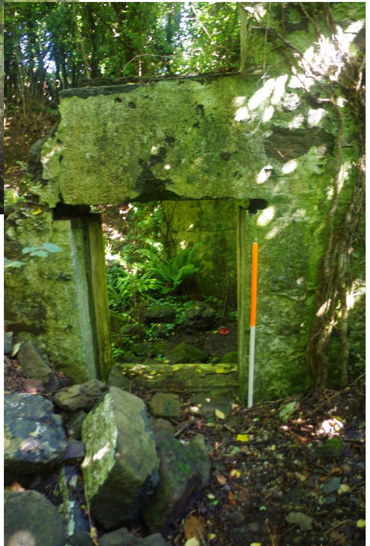
Fig 12 Carn Kennack, top – looking in to the internal south-eastern corner showing a low doorway and a large upper floor window; right – looking north-east in to the building. Note the rotted out timber lintel, upper window and heap of external wall tumble.
