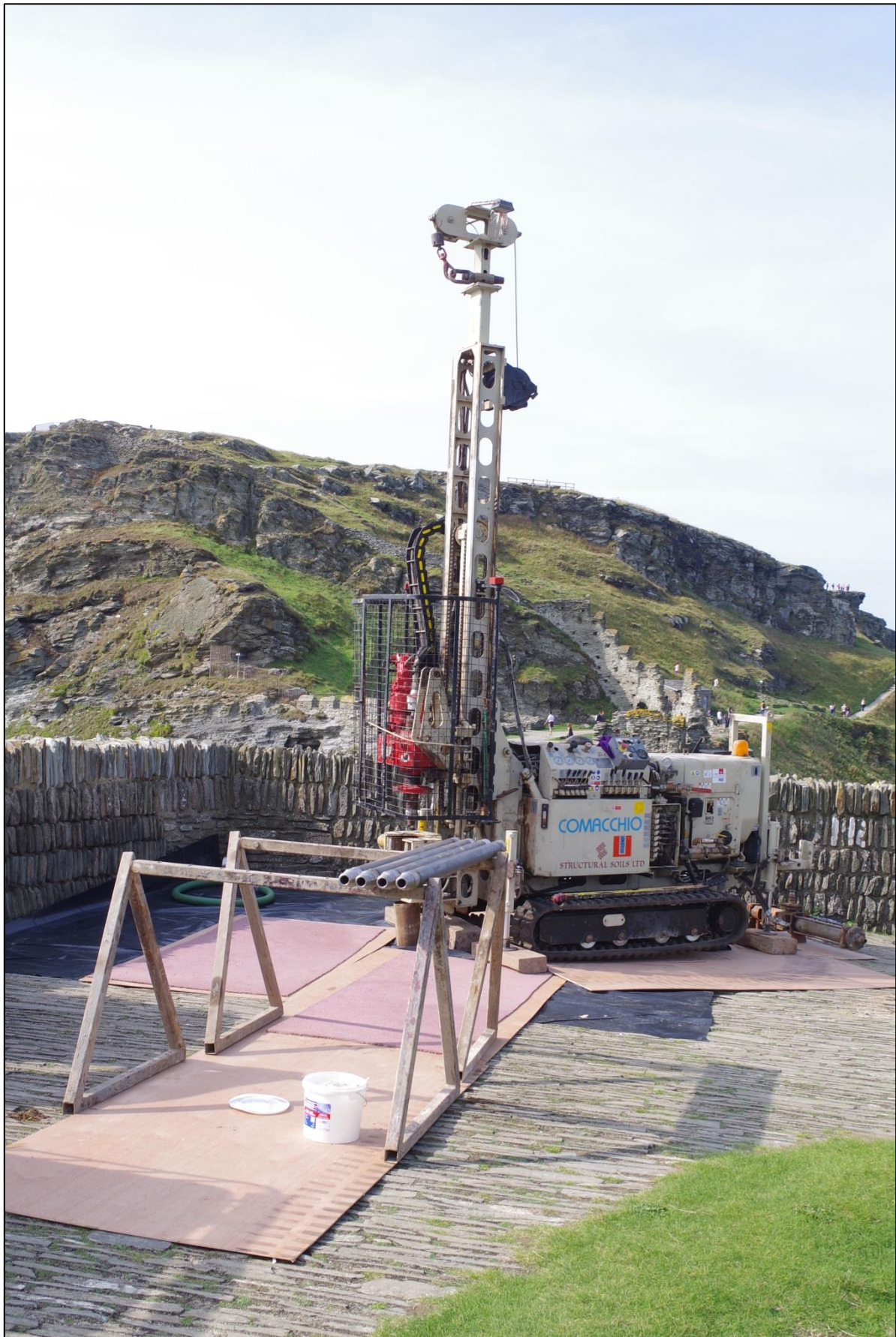
Figure 5: Drilling rig in situ borehole 1.
