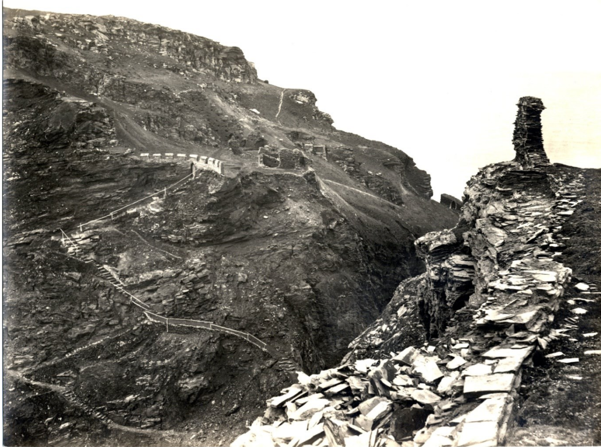
Fig 10. In this slightly later image, the lower section of the path can be seen to have been abandoned, and a new route had been cut down to and across the top of the neck.
