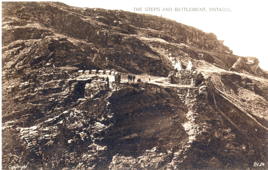
Fig 18. A relatively early (probably early C20 th ) view of the Inner Ward, showing the substantial erosion scar below and to the right of Kinsman's new walling, the right hand end of which had already collapsed.
