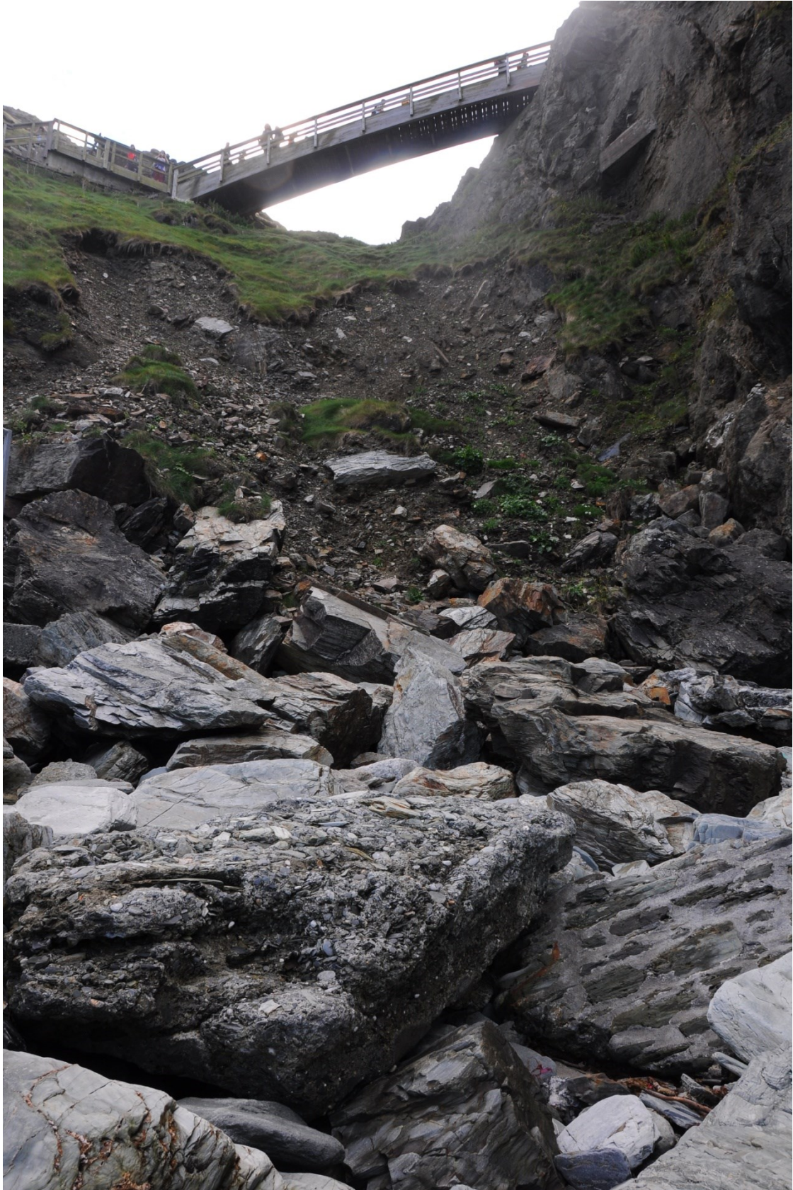
Fig 26. Looking up to the neck from the Haven, the instability of the land bridge is immediately evident, as is the absence of exposed solid rock within it on this side.
