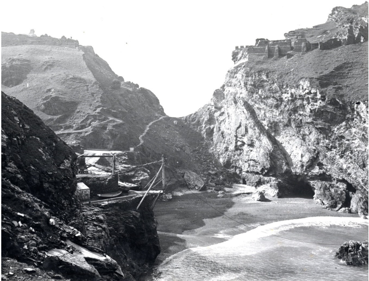
Fig 16. A good late 19 th century view looking from the Haven showing the access track leading up the neck. Note the clear evidence for major landslips on the slope below the Lower Ward.
