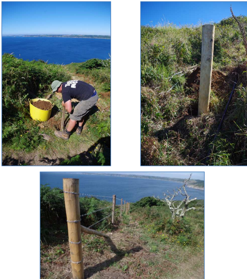
Figure 26 Digging postholes for the new line of fencing on the west side of Dodman Point
