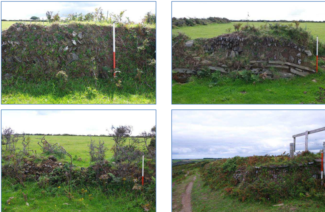
Figure 42 Boundary 14 showing different styles of stonework and evidence for repair. The west end of boundary 14 curves round to meet boundary 3
