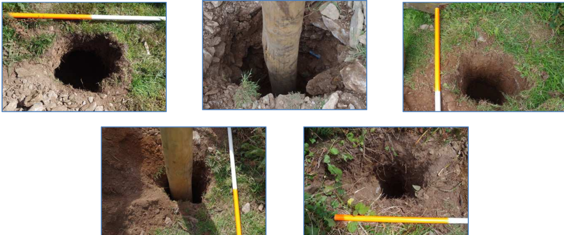
Figure 27 Postholes 1 to 5, dug to erect gateposts for two new gates and one existing gate leading on to the field lanes crossing the inner rampart
