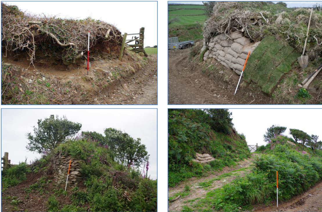
Figure 23 Clockwise, Erosion Area (E1) before, during and following repair in March, April and August 2016. The Cornish hedge adjacent to the gateway on the west side was also repaired
