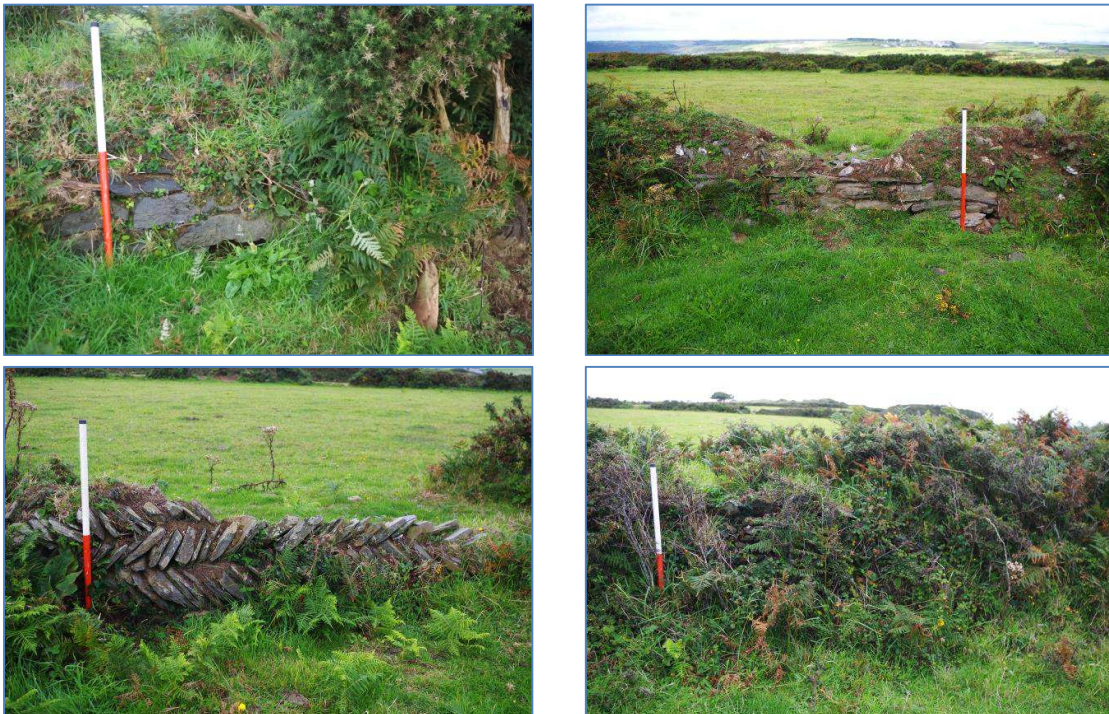
Figure 43 Boundary 15 showing different stonework styles and evidence of repair. A worked stone at the eastern end (top left) may have served as a drain
