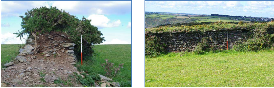
Figure 41 An eroded section across boundary 13 and a section of the south face showing coarse 'Jack and Jill' style stonework, capstones and one of the lateral piers
