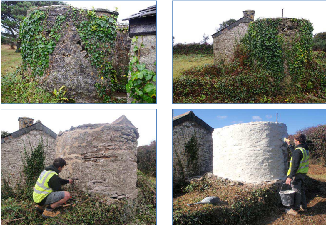
Figure 28 The watch house lookout platform before and during repair
