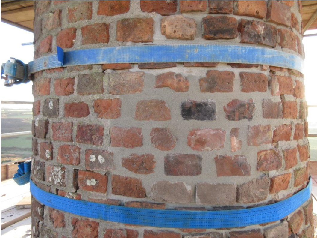
Fig 7. The sample pointing on the brickwork.
