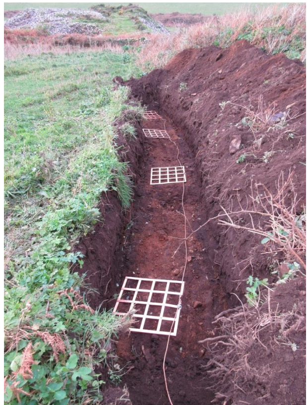
Fig 21. The earth mats installed in the trench.
