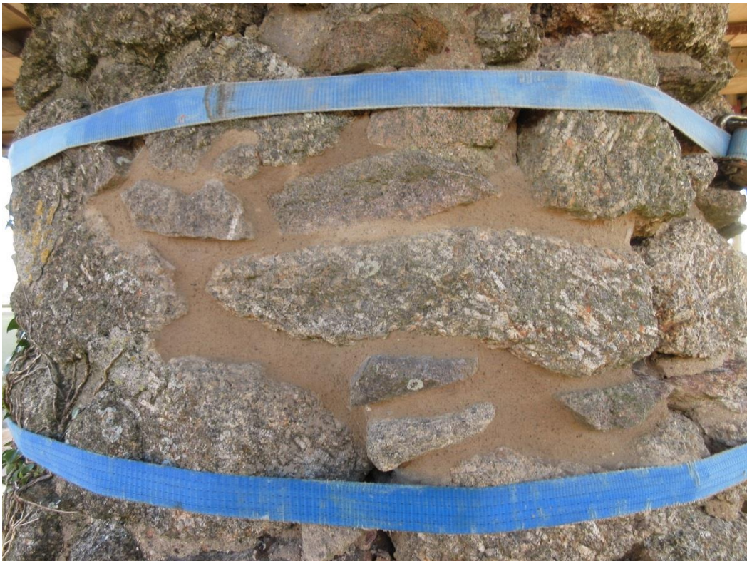
Fig 8. The sample pointing on the stone section of the chimney.
