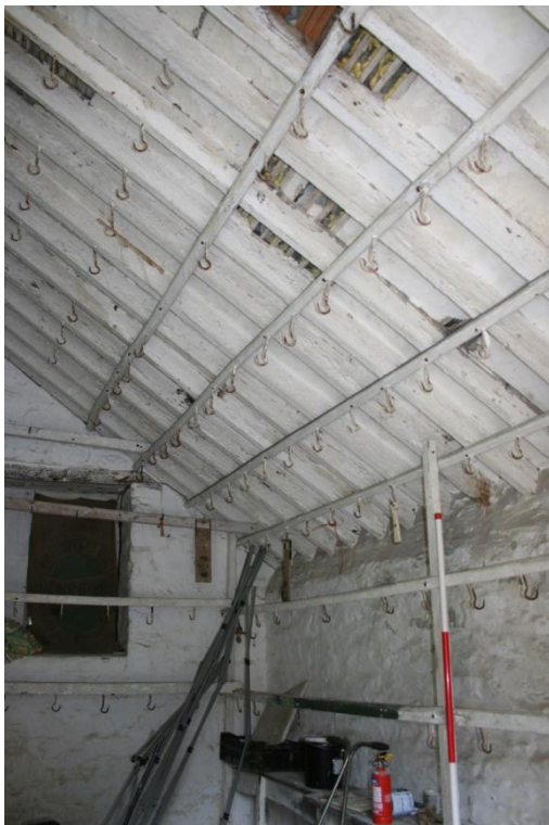
Figure 20 Stables Range – iron hooks within garage/game larder [7].
