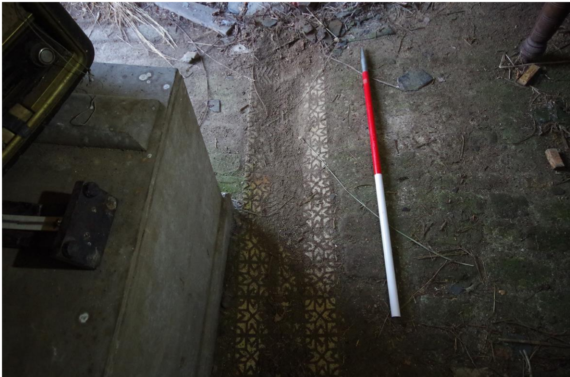
Figure 66 North-west Range - tiled drain within cow-house [21].
