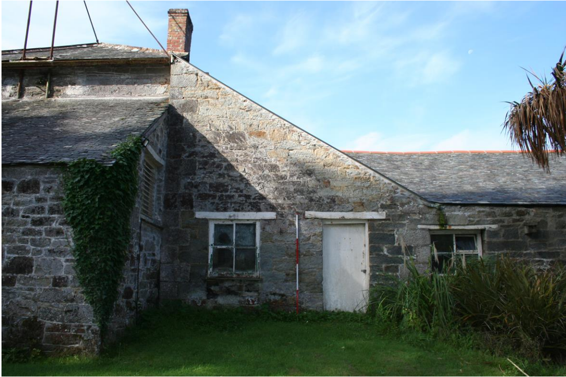
Figure 31 Corner between North-east (right), Stables (left) and Farmyard Ranges (centre) - exterior of the former working horse tack room and later farm office/crib room [12]. The left hand window is a converted doorway that once probably connected with an extension mapped here on the 1841 and 1880 maps.
