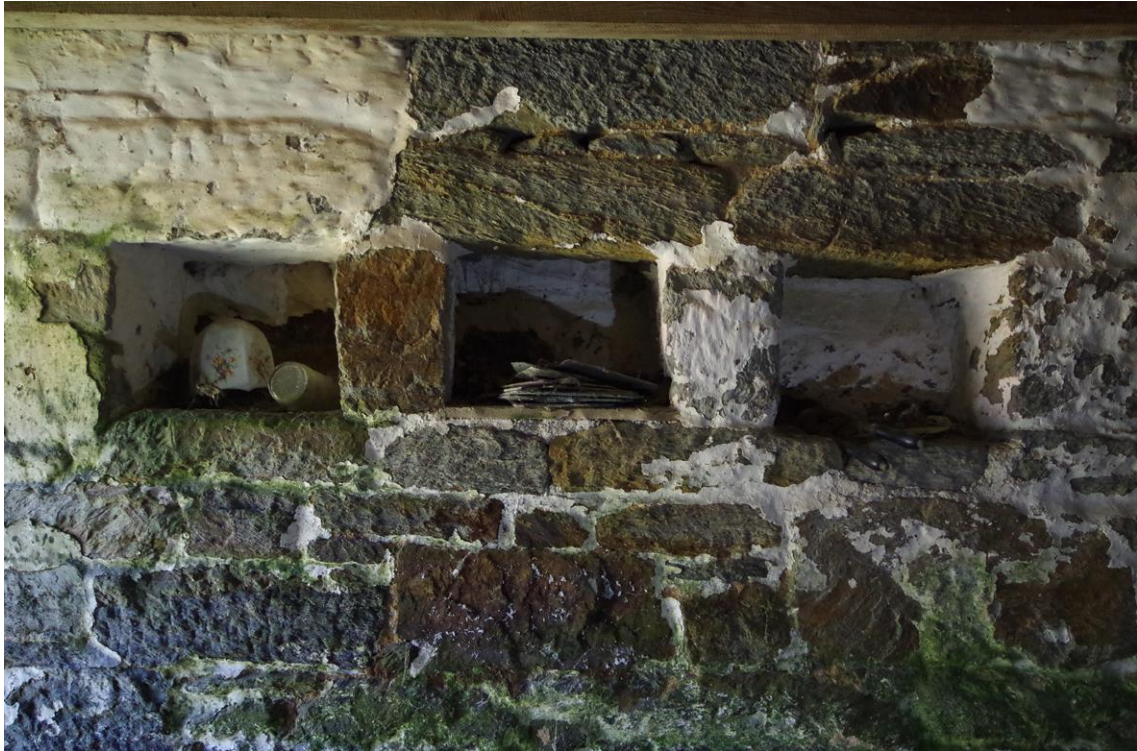
Figure 67 North-west Range - lintelled recesses or 'keeping places' within the central block.
