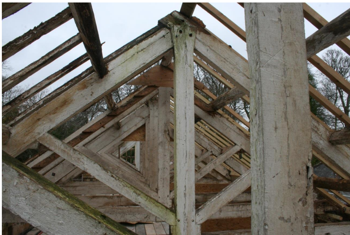
Figure 49 South-west Range - carpenter's marks on roof trusses.
