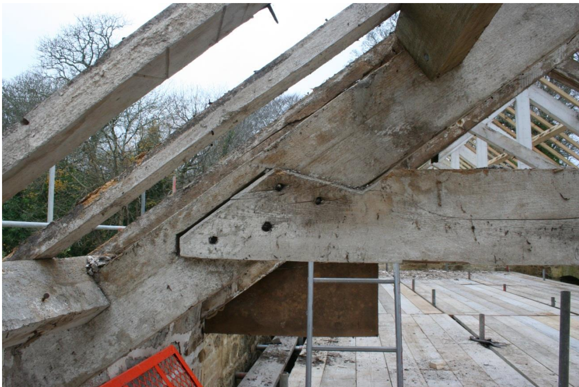
Figure 48 South-west Range - detail of roof collar joint.
