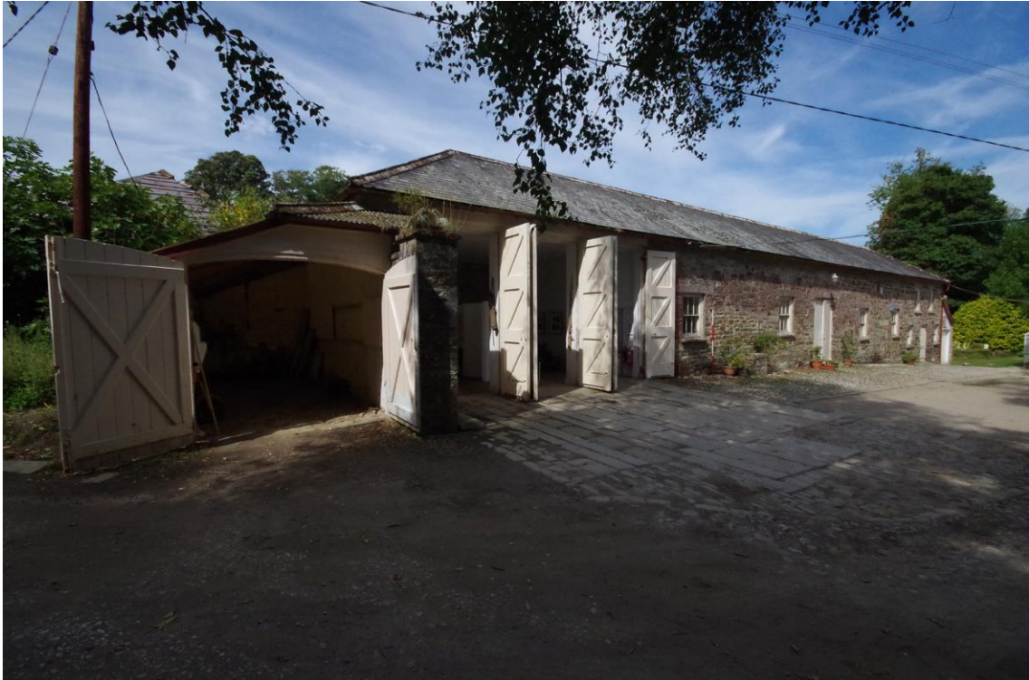
Figure 9 Stables Range - looking north along south-east elevation.
