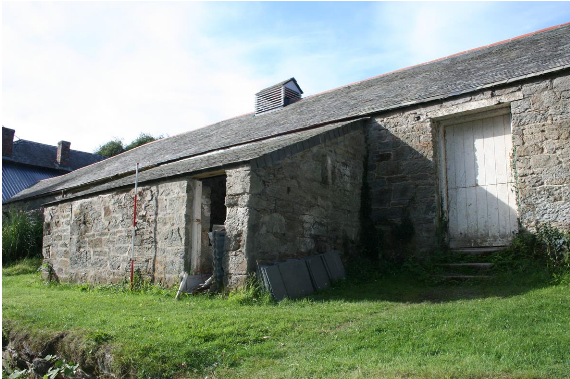
Figure 59 North-east Range - pair of later lean-to buildings (rooms [17] and 18]) added to the rear elevation.
