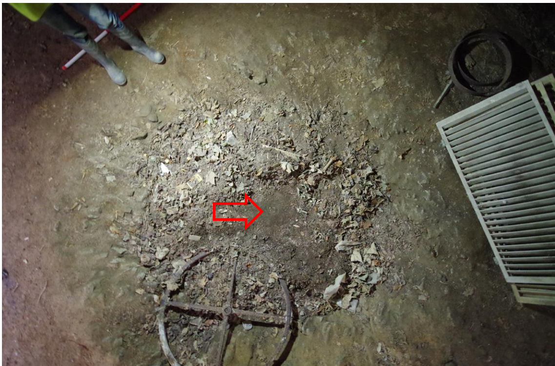
Figure 52 South-west Range - horse engine house [32]: looking down from first floor towards in situ lower bearing (arrowed).
