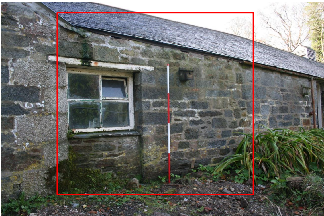
Figure 58 North-east Range - exterior view showing location of original farmyard gateway.
