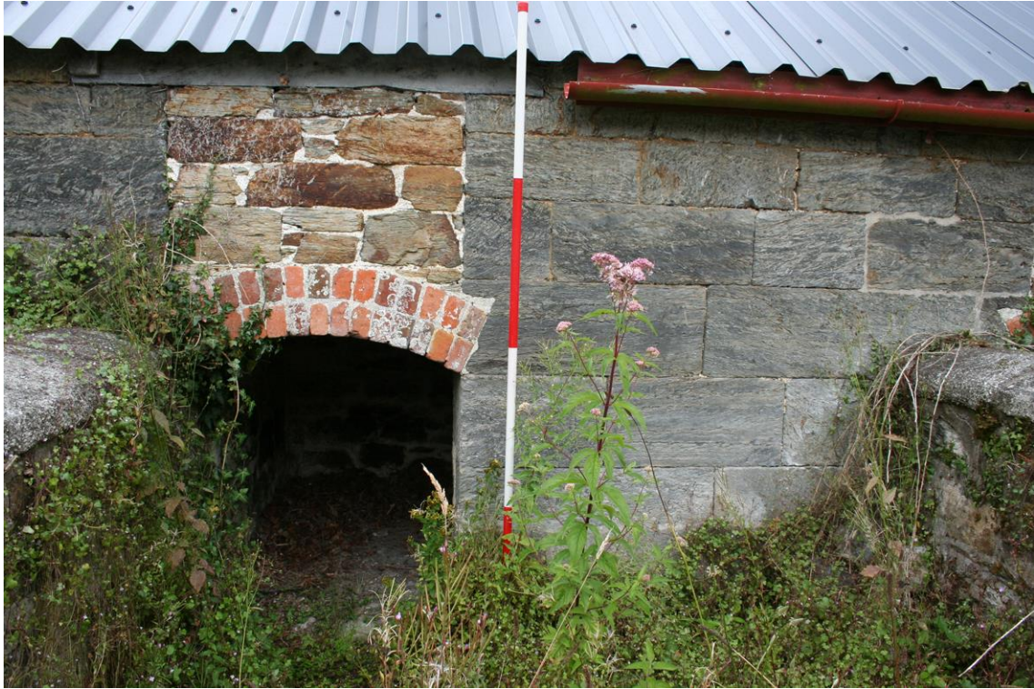
Figure 69 North-west Range - pigsty doorway and run.
