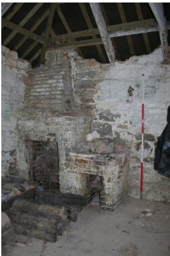
Figure 62 North-east Range - swill boilers in room [16].
