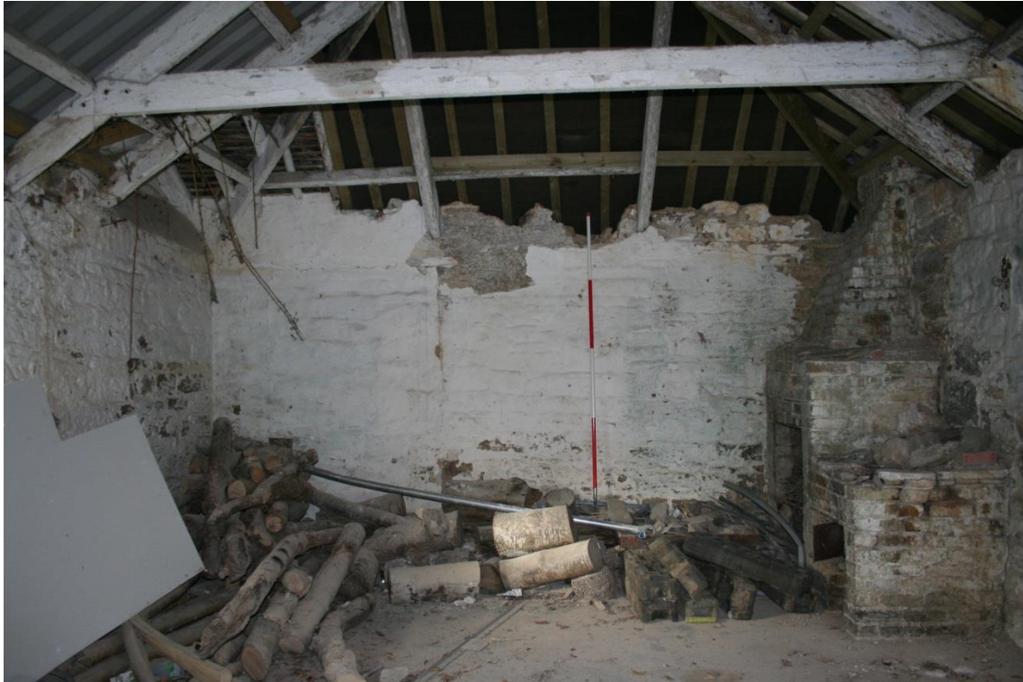
Figure 61 North-east Range - interior of room [16].
