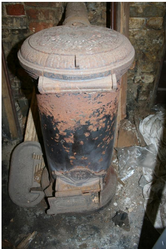
Figure 28 Stables Range – stove within former tack room [8].
