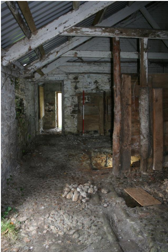
Figure 32 Farmyard Range – interior of working horse stable [11] showing cobbling, stalls (right) and doorway to former working horse tack room.
