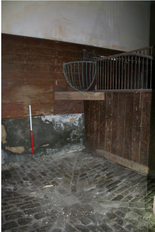
Figure 25 Stables Range – stables [5], showing interior stall detail, drain and hay rack.
