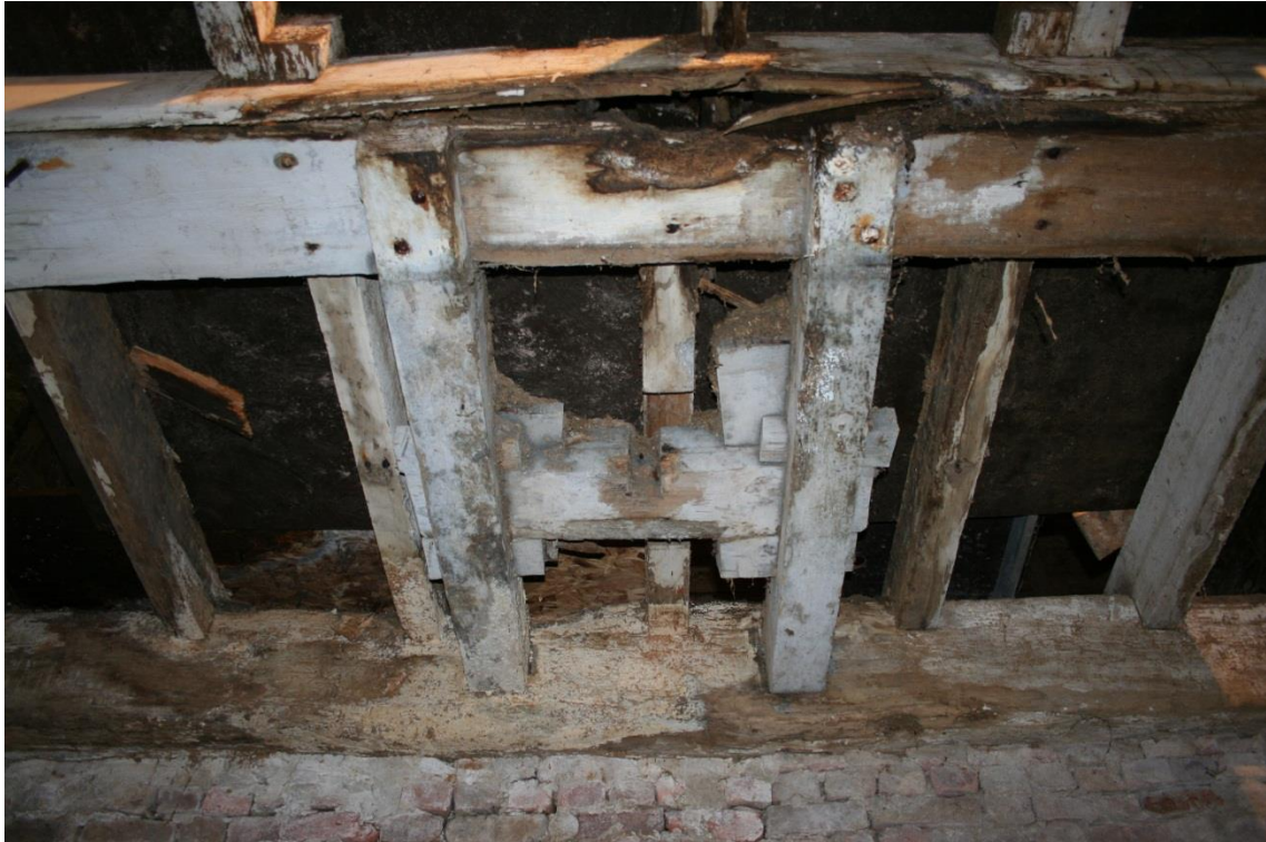
Figure 43 South-west Range - bearing support for vertical axle within ceiling of room [25].
