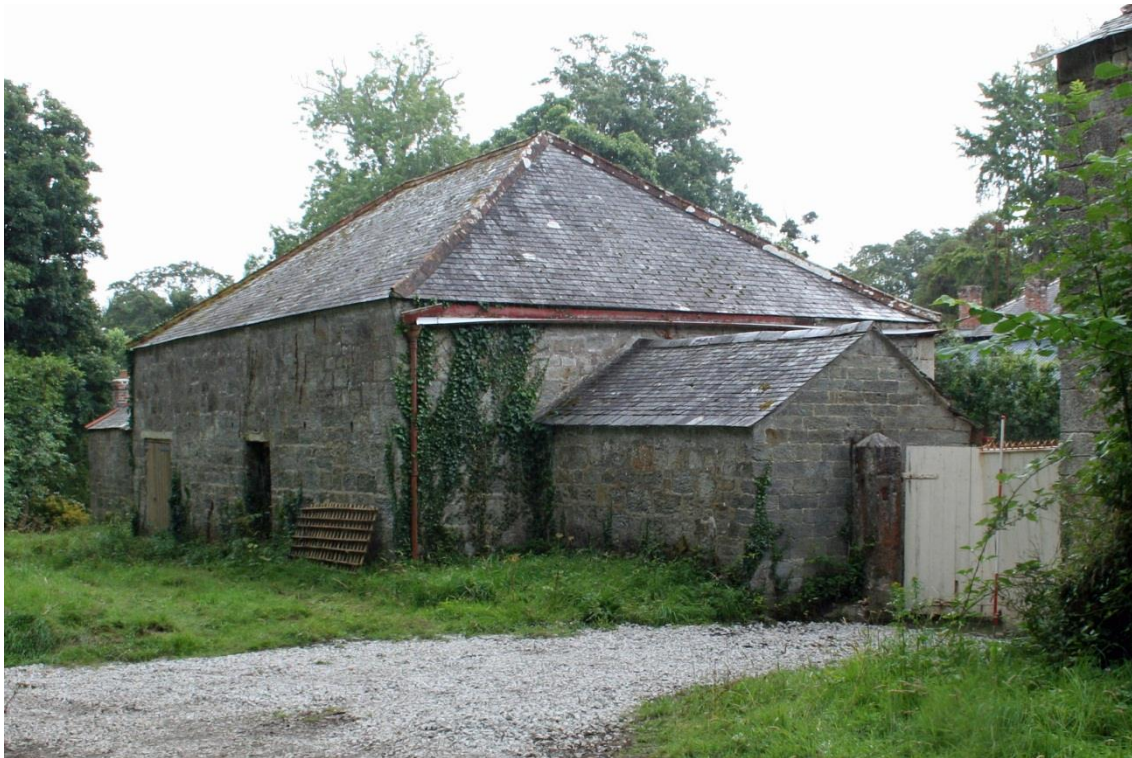
Figure 63 North-west Range – rear view, showing the inserted farmyard gateway and rebuilt gable of the adjoining pigsties.
