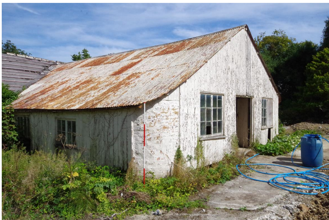
Figure 50 South-west Range – looking east to the exterior of the horse engine house, showing first floor addition [33].
