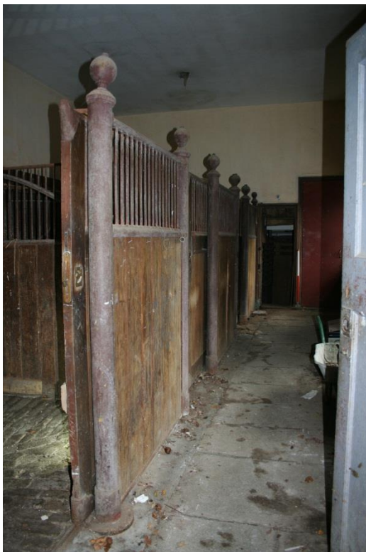
Figure 24 Stables Range – stables [5], showing stall and corridor detail.
