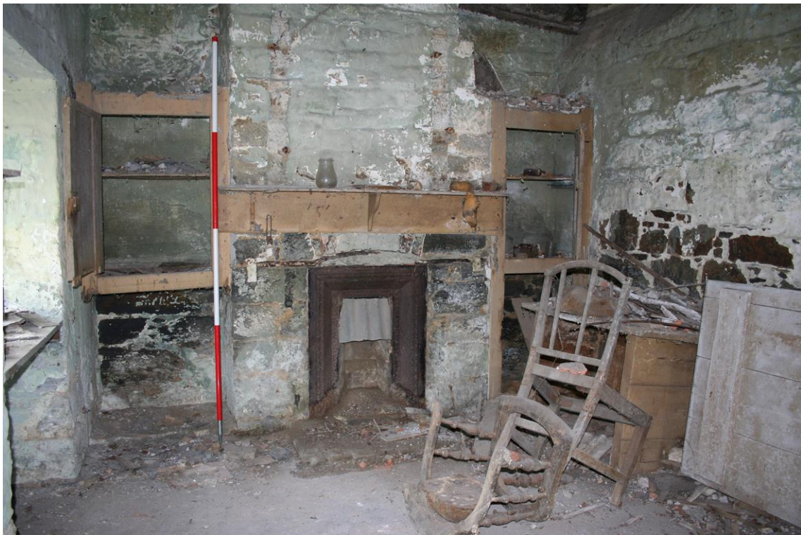
Figure 30 Farmyard Range – former working horse tack room (and later farm office or crib room [12])
