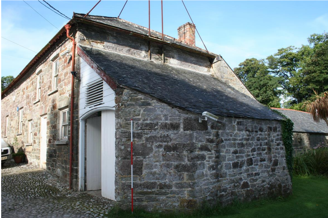
Figure 19 Stables Range – later garage/game larder [7] lean-to added to range by 1907.
