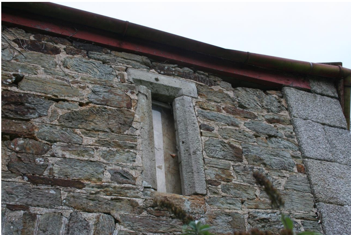
Figure 64 North-west Range - loft opening in central block, showing reused dressed masonry window parts.
