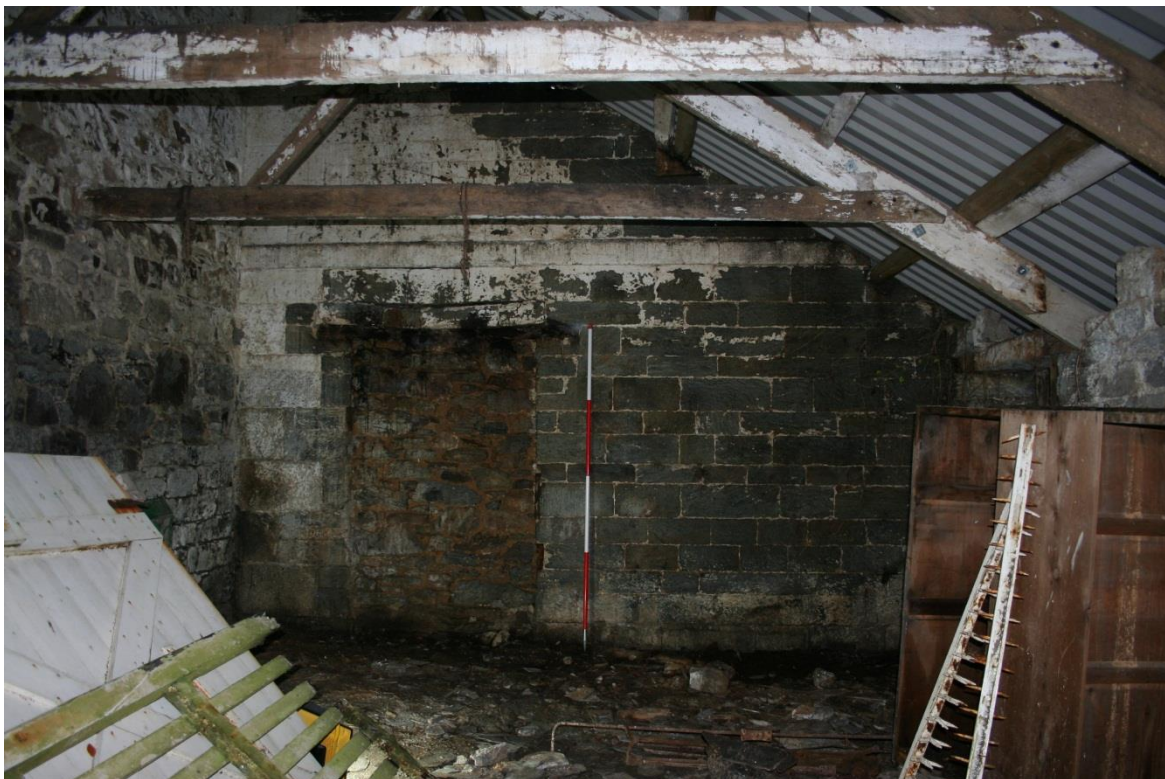
Figure 34 Farmyard Range – interior of former cow-house [9] with inserted (and later blocked) doorway to South-west Range to rear left.
