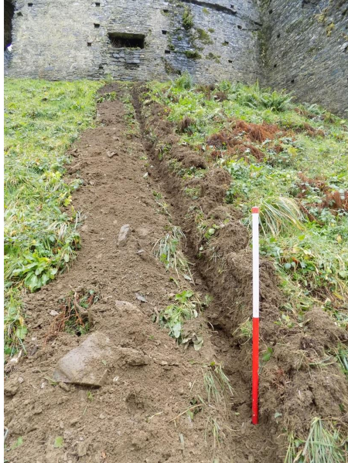
Figure 6. Detail of conductor tape trench looking south west.
