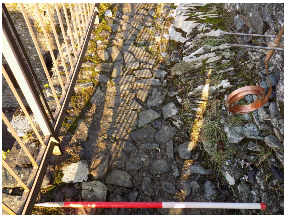
Figure 11. Slot 1. Detail of wall walk surface.
