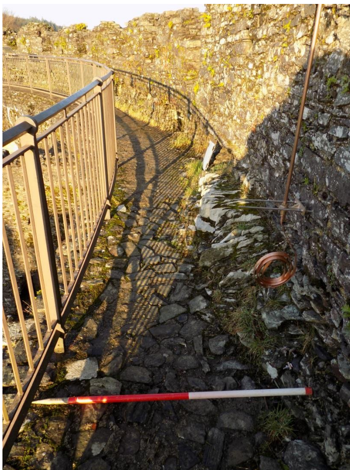
Figure 10. Slot 1. Location adjacent to lightning conductor.
