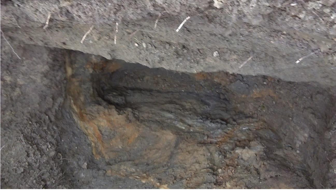
Figure 8. Mining mitigation work within openwork showing possible tunnel(Photograph courtesy of Alan Caddy).
