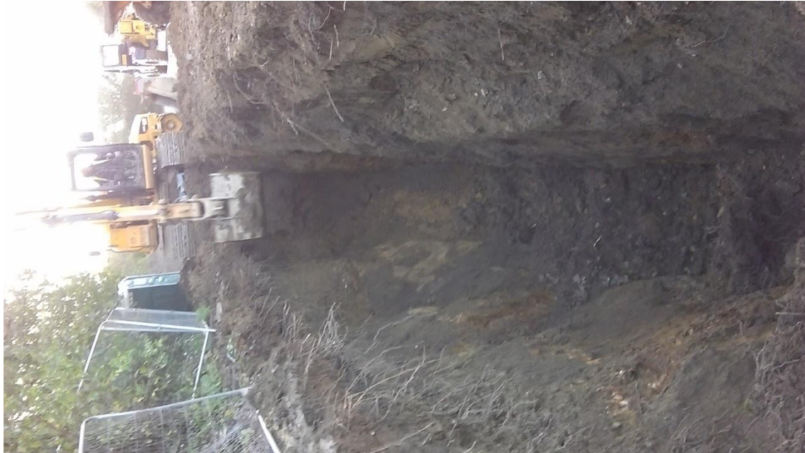
Figure 7. Mining mitigation work within openwork illustrating the depth of the feature (Photograph courtesy of Alan Caddy).
