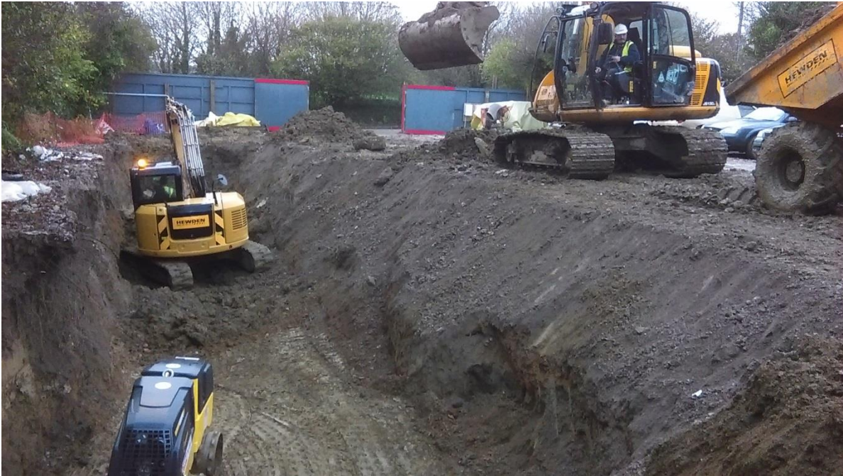
Figure 9. Mining mitigation work within openwork showing width of the feature (Photograph courtesy of Alan Caddy).
