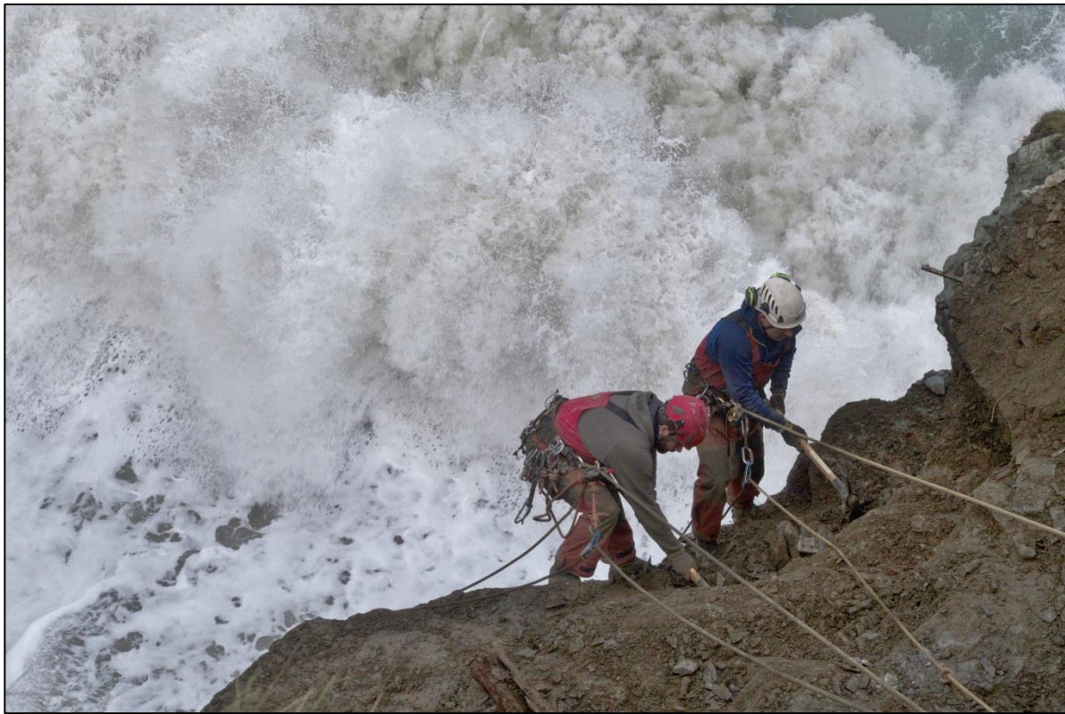
Fig 15. Vertical Technology staff clearing steps cut into the cliff face.
