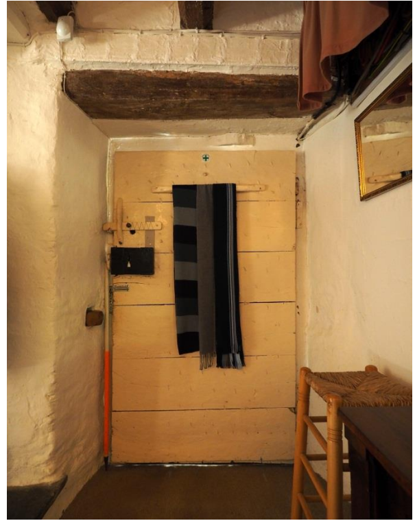
Fig 19. C17 front door and drawbar slot
