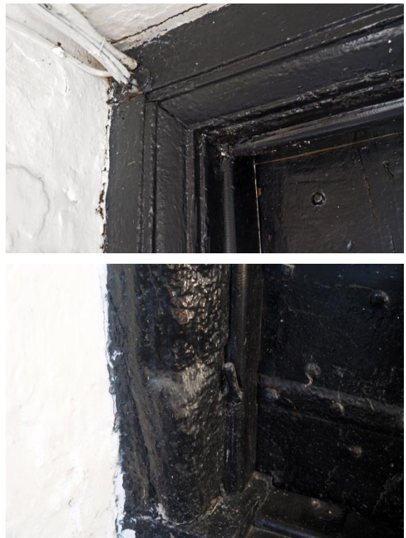
Fig 17. Doorframe mouldings and stop
