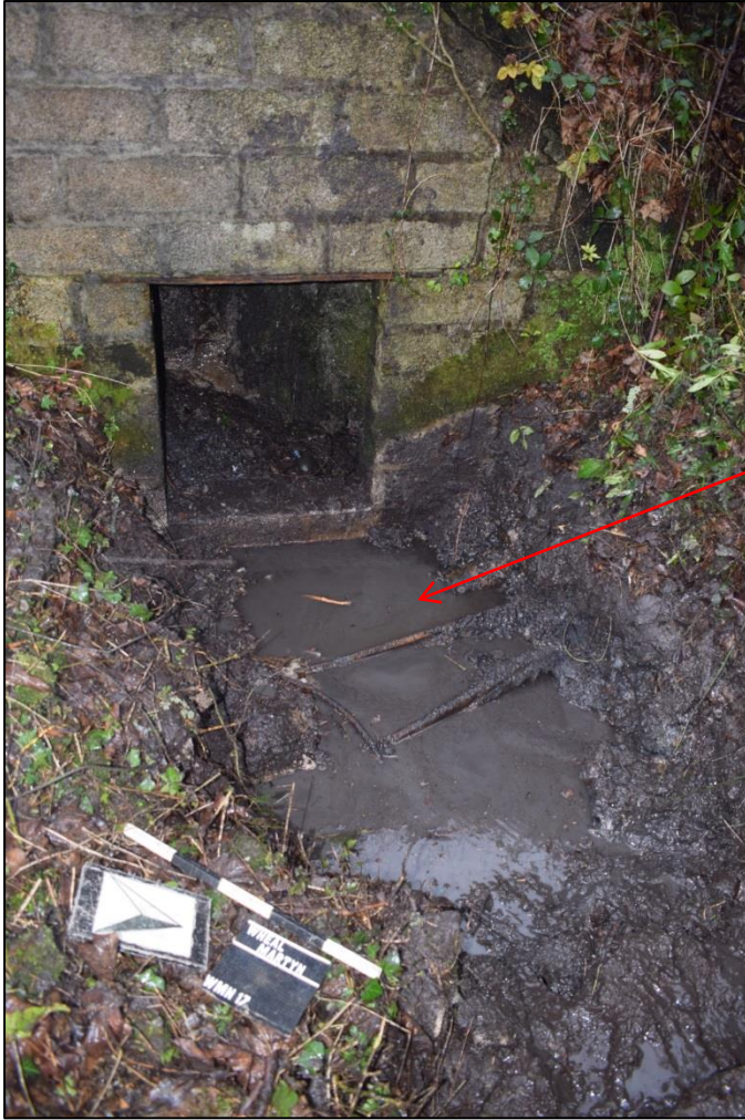
Figure 10: Trench 4 post excavation.
