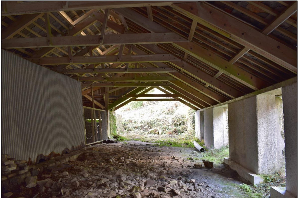
Figure 6: View through Mica Dry looking west-south-west, prior to excavation.
