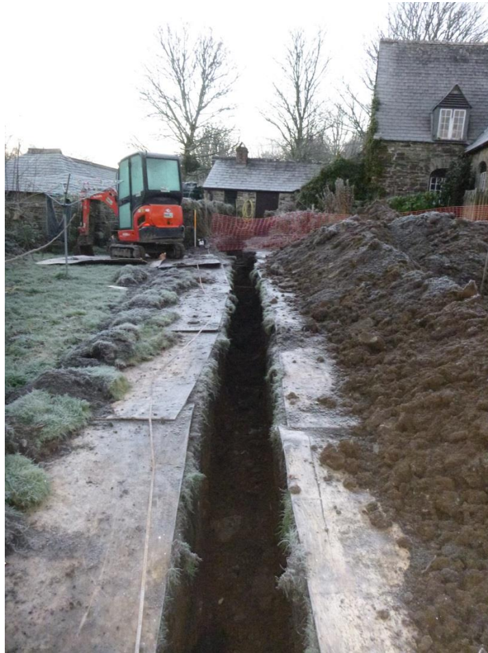
Figure 6. Trench 6 looking south west.
