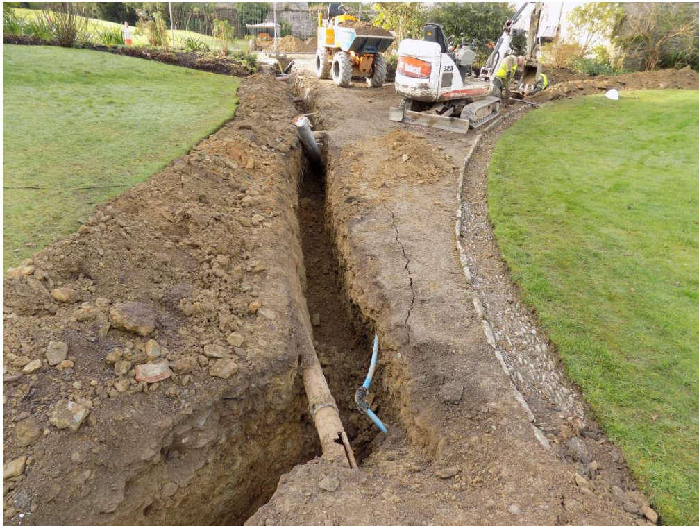
Figure 10. Trench 9. East end, looking westwards.
