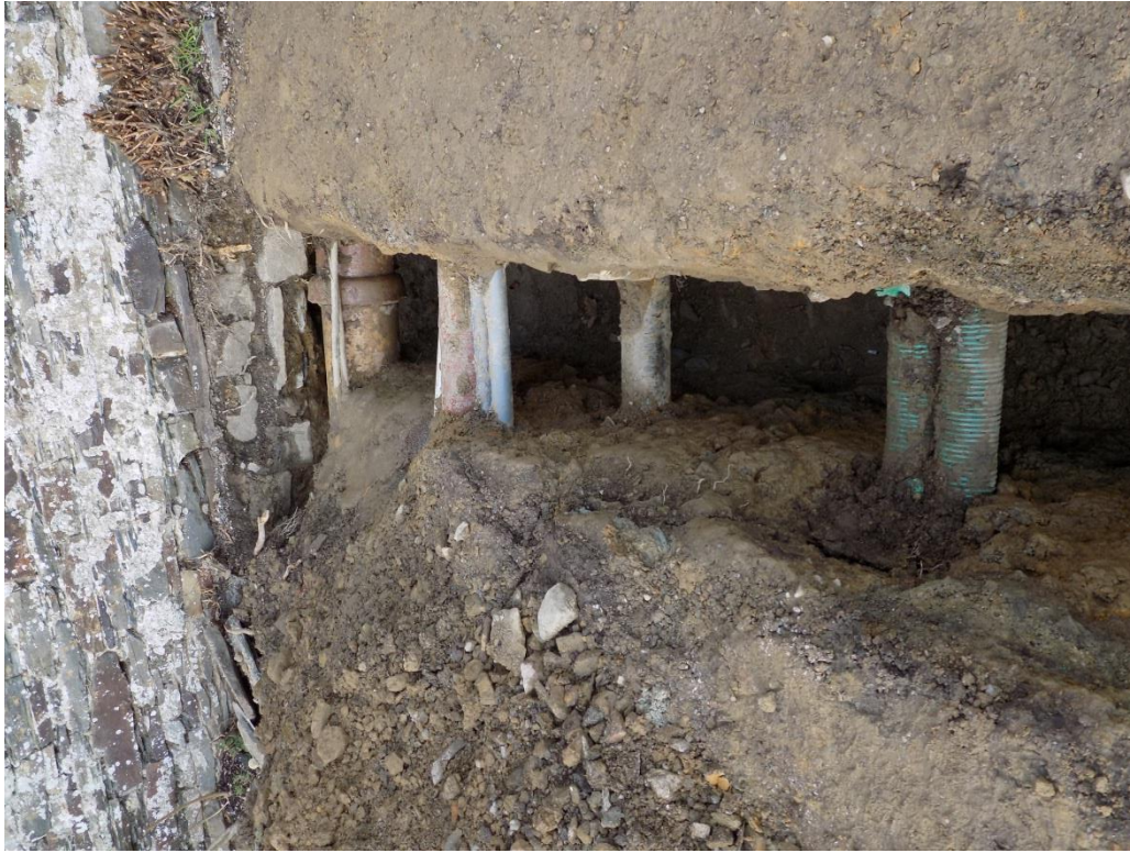
Figure 9. North end of Trench 8 showing the density of services encountered.
