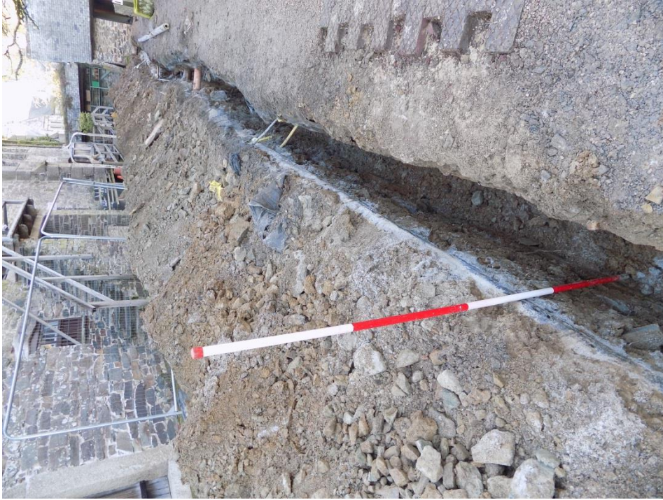
Figure 13. Trenches 12, 14 and 16 looking east.
