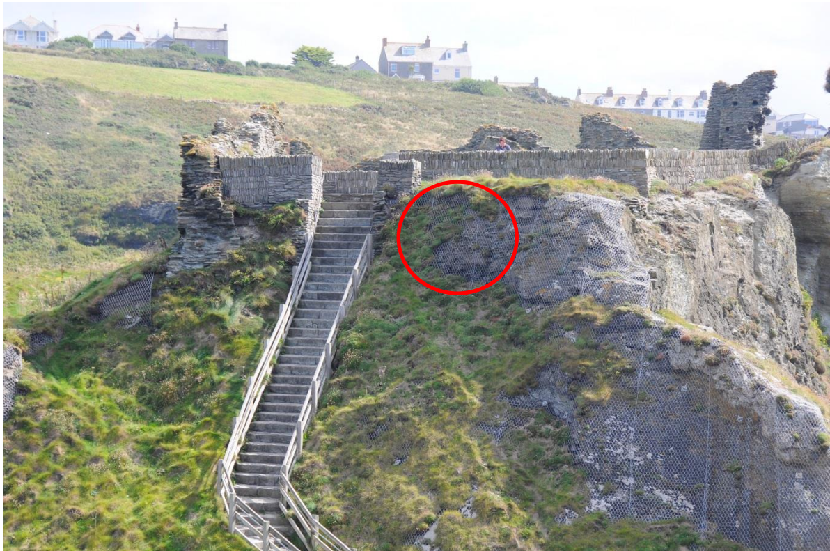
Fig 3. The northern end of the Lower Ward at Tintagel Castle. The location of the proposed bridge abutment is circled.
