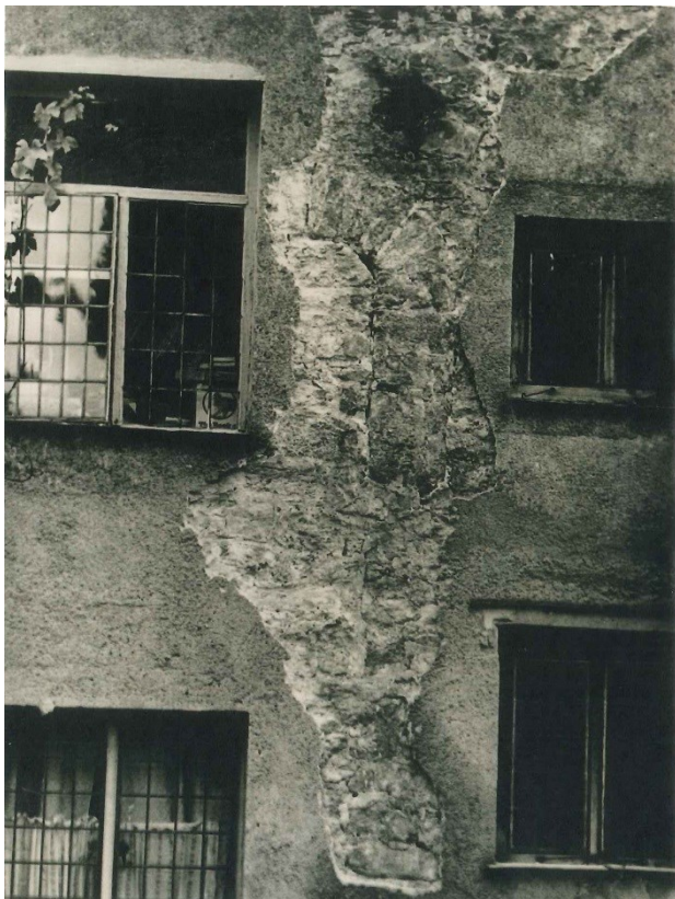
Fig 56 Blocked round arch probable door opening in first floor of south range (Bradley archive.).
