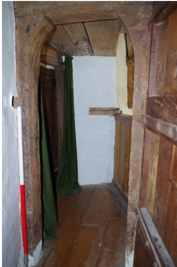
Fig 199 Room 24 door frame to chapel balcony looking north.
