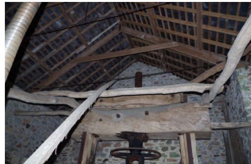
Fig 272 Pound House room 3 cider press and roof structure at north end.
