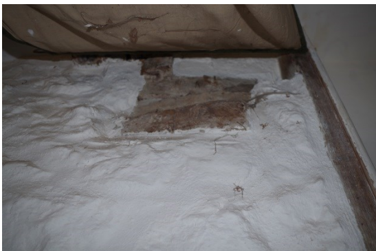
Fig 140 Room 8 sawn off timber at north end of west wall.
