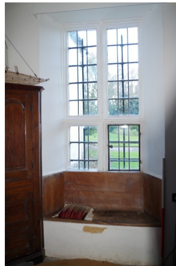
Fig 99 Room 4 transom window at north end.
