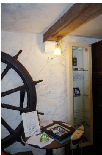
Fig 125 Room 6 scar of removed return wall in south wall.
