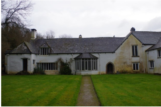
Fig 80 West elevation of East Range.
