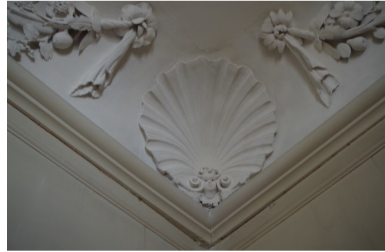
Fig 236 Room 31 detail of plasterwork.
