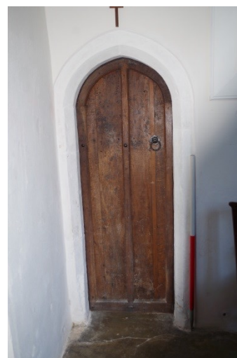
Fig 100 Room 4 door opening in north wall.
