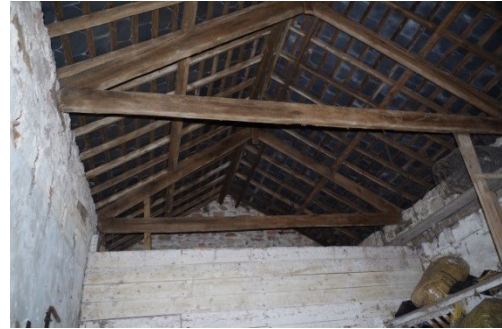
Fig 270 Stables roof structure at south end.
