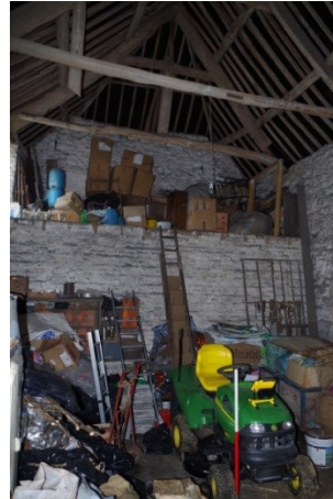
Fig 175 Room 18 looking south.
