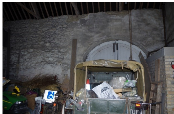
Fig 178 Room 18 looking west.
