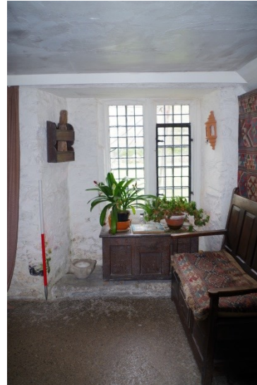
Fig 126 Room 6 window inserted in larger opening in west wall.
