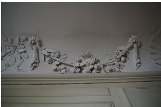
Fig 235 Room 31 detail of plasterwork.
