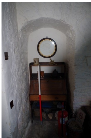
Fig 103 Room 4 blocked door opening at south end of west wall.
