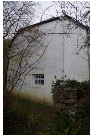
Fig 77 South elevation of Coach House.
