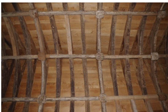
Fig 91 Room 3 roof structure.
