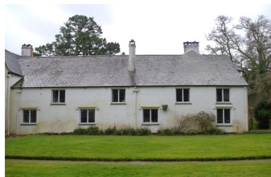
Fig 79 North elevation of South Range.
