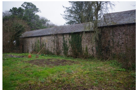
Fig 264 West elevation of stables and Pound House.
