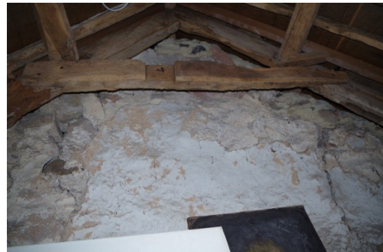
Fig 237 Attic above Room 30, rubble gable end wall to east.
