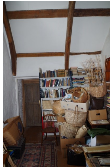
Fig 195 Room 24 looking south.
