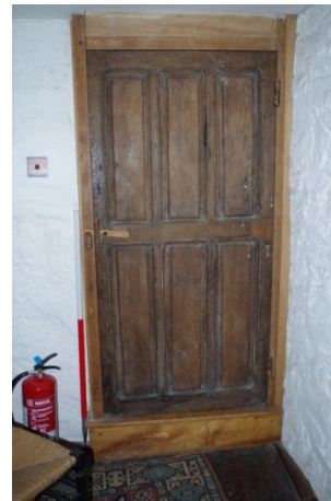
Fig 207 Room 25 inserted door opening in north wall.
