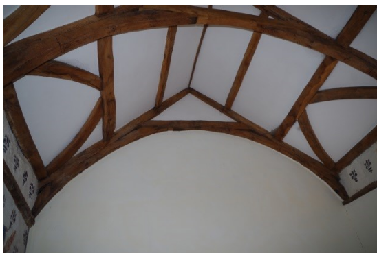
Fig 241 Room 32 roof looking west.
