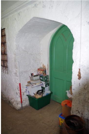
Fig 150 Room 9 door opening to room 13.
