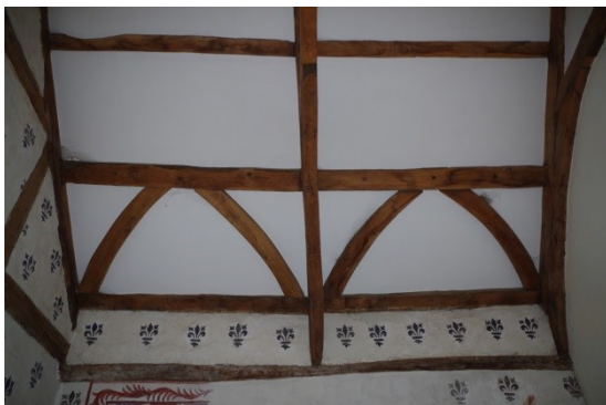
Fig 242 Room 32 roof looking south.
