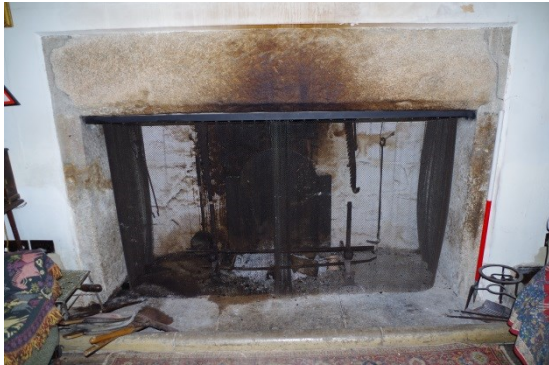
Fig 109 Room 5 fireplace in east wall.
