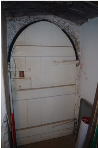
Fig 163 Room 11 door to room 9.
