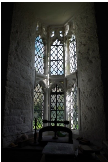
Fig 205 Room 25 oriel window in east wall.
