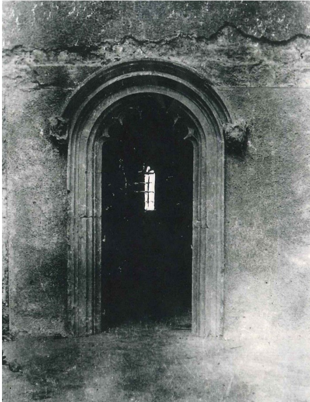
Fig 55 Doorway constructed from reused window masonry (since removed) in the south elevation of the South range. Formerly referred to as the 'Saxon Door' (Bradley archive.).
