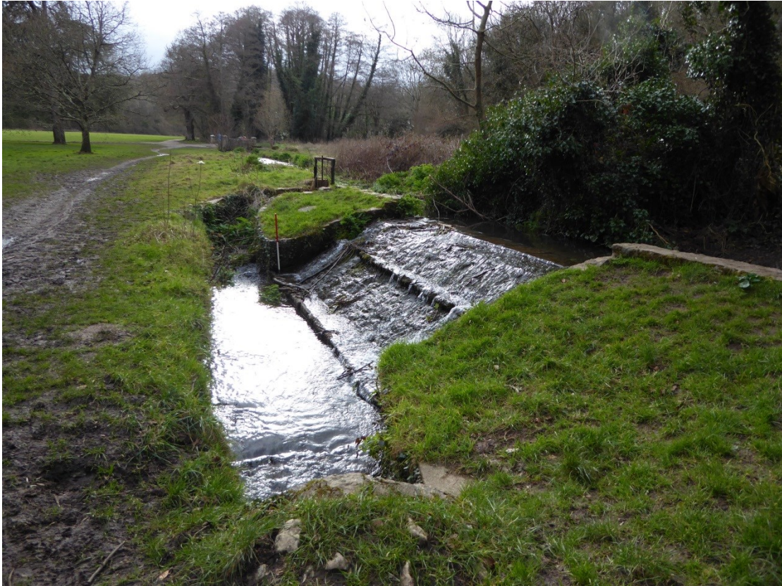
Fig 67 The cascade, spillway and sluice (NT 160070) on the leat below Bradley, looking west towards the leat bridge. This view can be compared with numerous images from a similar viewpoint which were produced in the late 19 th and early 20 th centuries.
