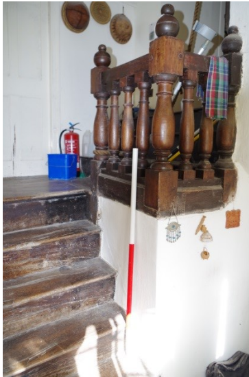
Fig 185 Room 20 staircase looking north-east.
