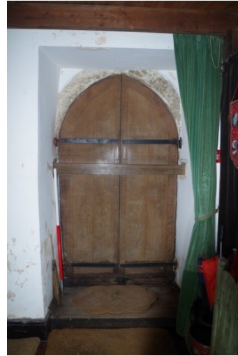
Fig 118 Room 5 screens passage door in west wall.
