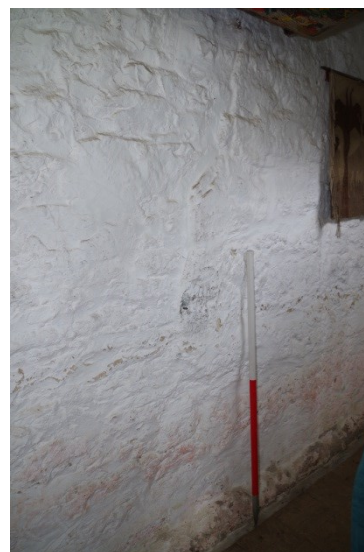
Fig 149 Room 9 masonry joint in south wall (former external wall).
