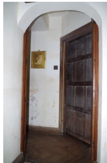
Fig 143 Room 9 east end of passage looking east.
