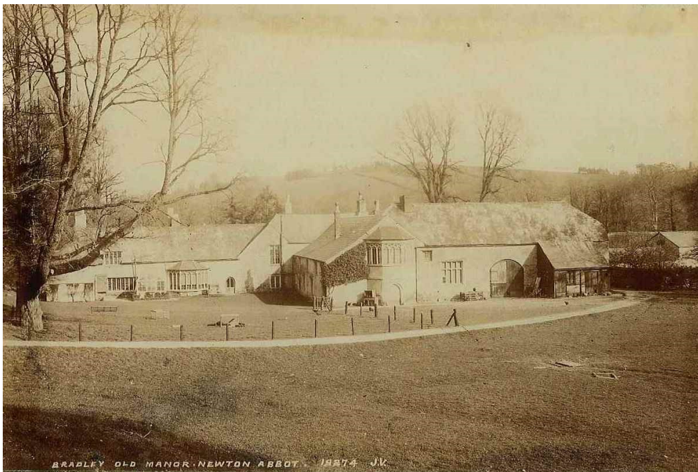
Fig 46 Undated, late 19 th or early 20 th century postcard view of the west side of the house, from The Lawn. The rear garden is separated from the Lawn only by a post and wire fence, a remnant of the former 'park' landscape. A track passing the south side of the Barn Range 'coachhouse' rises on a sloping embankment to join the carriage drive to the north. The slight earthwork feature turning a sharp angle in the right foreground is probably the route of the culvert which formerly fed the pond to the south of the house (cf Fig 13). (Bradley archive.)
