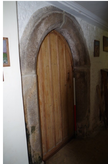
Fig 148 Room 9 door opening to room 11.
