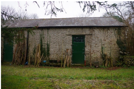
Fig 260 North end of east elevation of stables.
