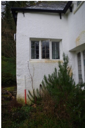
Fig 81 South elevation of north-west extension.
