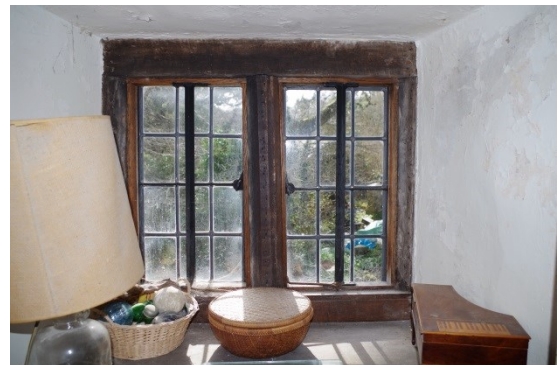
Fig 222 Room 28 window in south wall.
