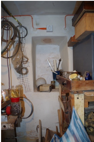
Fig 157 Room 11 blocked probable window opening in north wall.
