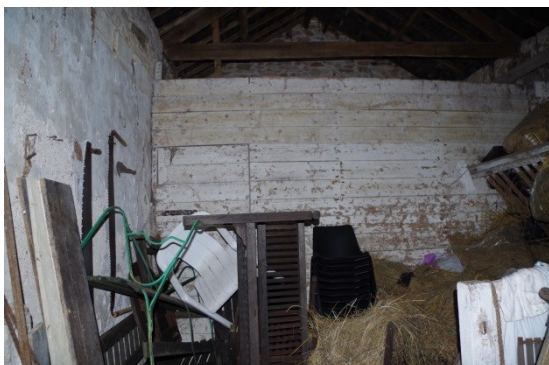
Fig 268 Stables Room 1 looking south to partition wall.
