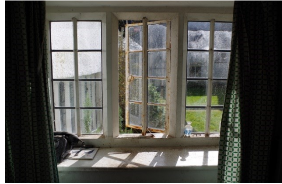
Fig 187 Room 20 inserted window in blocked door opening in south wall.
