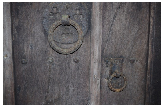
Fig 128 Room 7 (porch) looking west door furniture.
