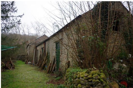
Fig 259 North and east elevation of stables and Pound House.
