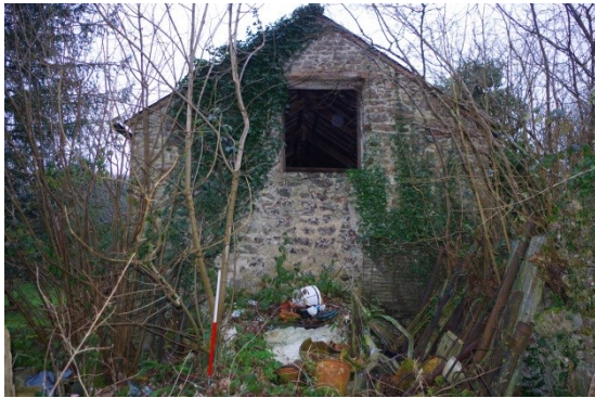
Fig 258 North elevation of stables.
