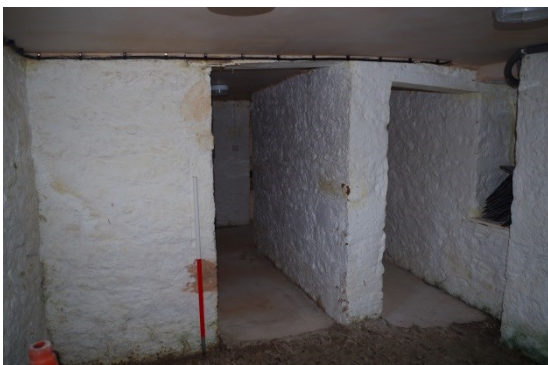
Fig 299 Lodge, room 9 looking south.
