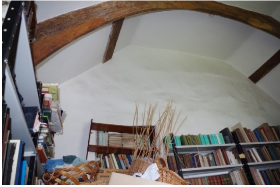
Fig 197 Room 24 looking west.
