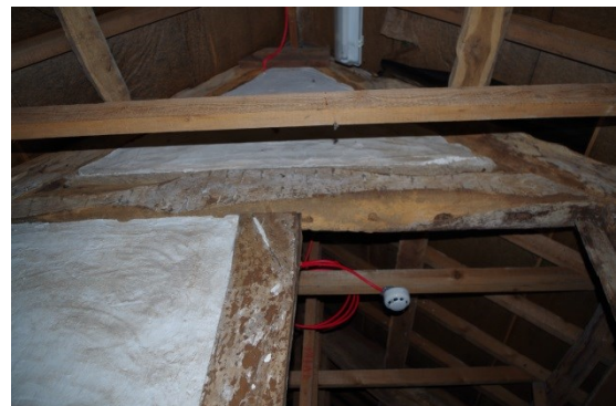
Fig 238 Attic above Room 30, timber framed wattle and daub wall to west.
