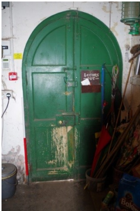
Fig 172 Room 14 external door in east wall.
