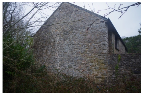
Fig 265 South elevation of Pound House.
