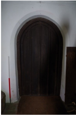
Fig 129 Room 7 (porch) looking south.
