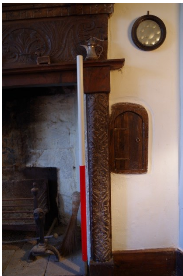
Fig 211 Room 26 fireplace and cupboard.
