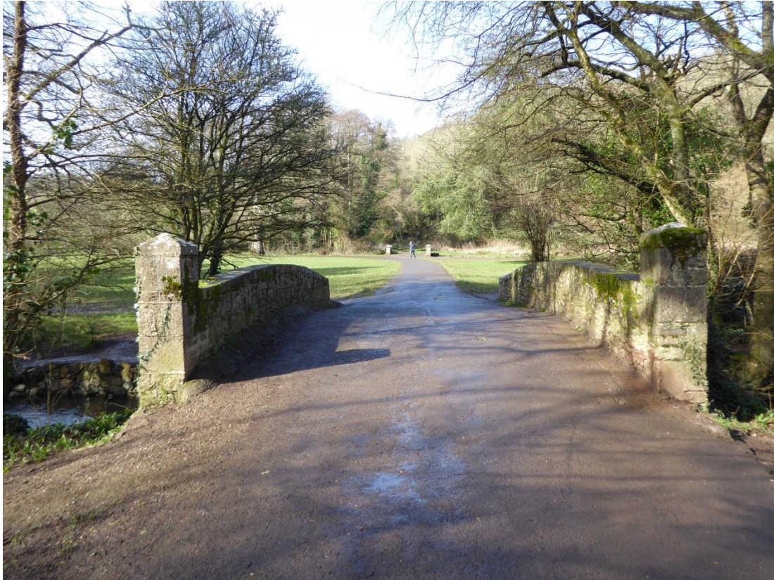
Fig 69 The approach to Bradley via the drive from the Totnes road crosses the 1826 bridge across the River Lemon and continues over the leat bridge seen in the middle distance.
