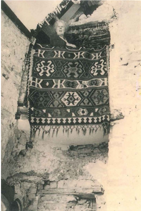
Fig 57 Removed spiral stair in Chapel showing blocked door opening at ground floor level (Bradley archive.).
