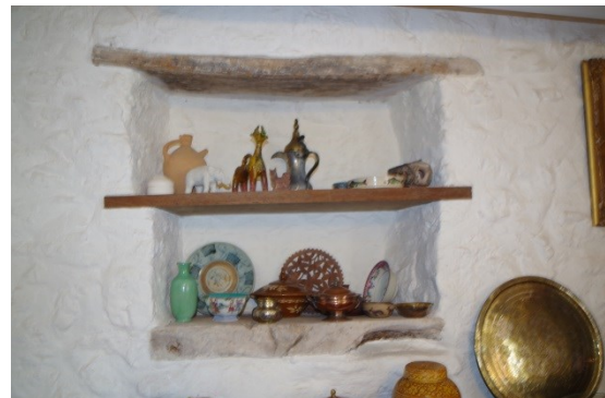
Fig 142 Room 8 blocked opening or recess in north wall.
