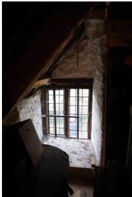
Fig 225 Window in south wall of Room 38 above Room 28.
