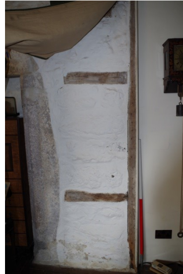
Fig 141 Room 8 timbers inserted at north end of west wall.
