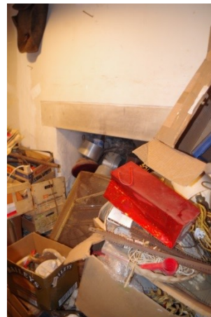
Fig 162 Room 11 fireplace in south wall.
