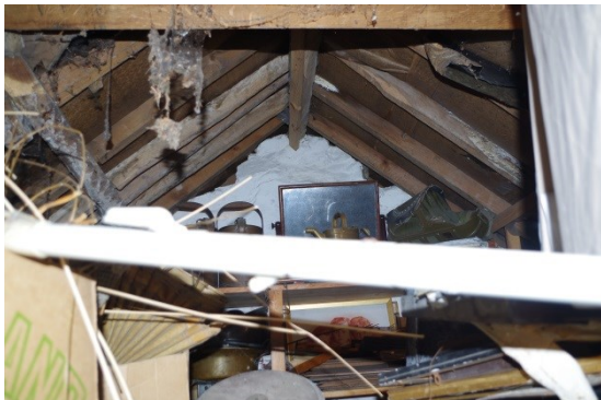
Fig 226 Room 38 above Room 28 looking west to phase 1 gable end wall.
