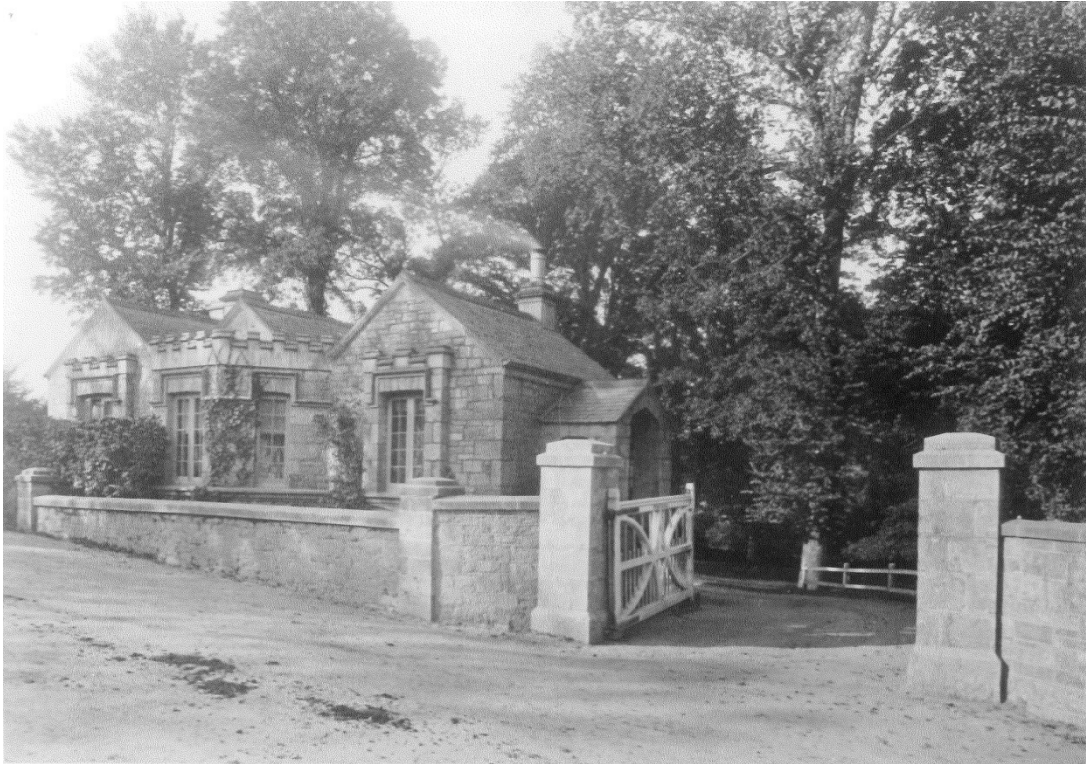
Fig 51 The Totnes Road lodge, probably built by the Reverend Wall in the mid 19 th century. This early 20 th century photograph (Bradley archive) shows a significantly different layout from that which exists at present. Much of the wall fronting the lodge has been lost to a rise in the level of the main road and the gate piers and gate have been moved and are now set back behind the porch and main door to the lodge.
