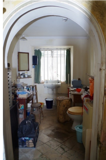
Fig 153 Room 10 looking south to blocked door opening with inserted window.
