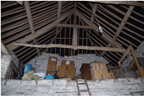
Fig 180 Room 18 looking south at roof.
