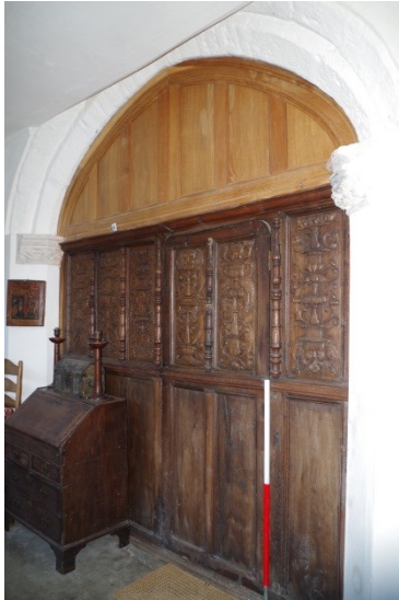
Fig 101 Room 4 arched opening with carved screen.
