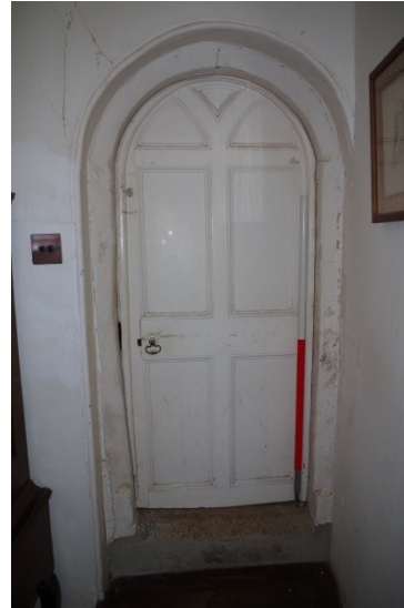
Fig 213 Room 26 door to room 25 in north wall.
