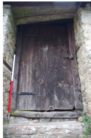
Fig 263 Loft door in east elevation of Pound House.
