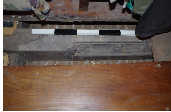
Fig 194 Room 23 carved probable door jamb reused as part of floor structure.
