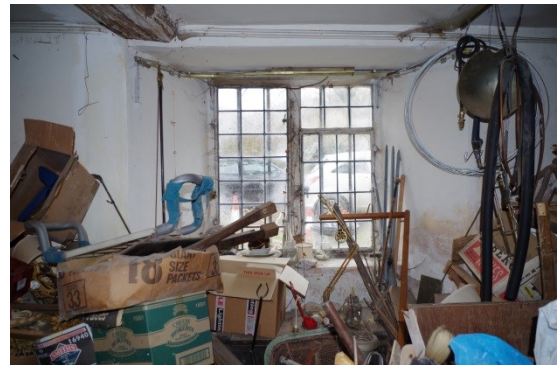
Fig 160 Room 11 window at east end of south wall.
