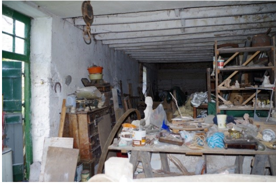
Fig 266 Stables Room 1 north end looking south.
