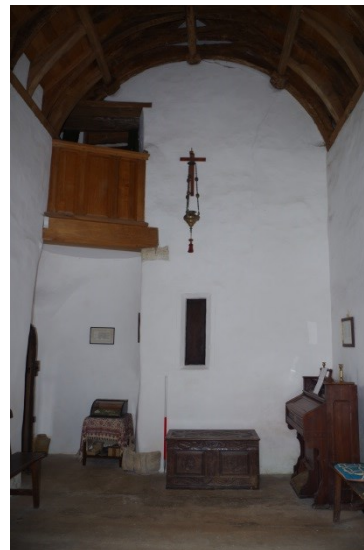
Fig 93 Room 3 looking west.
