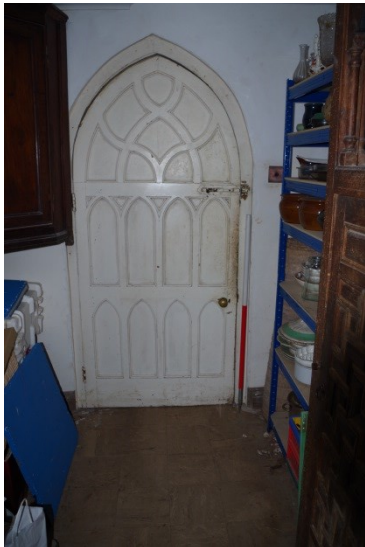
Fig 151 Room 9 door opening to room 12.
