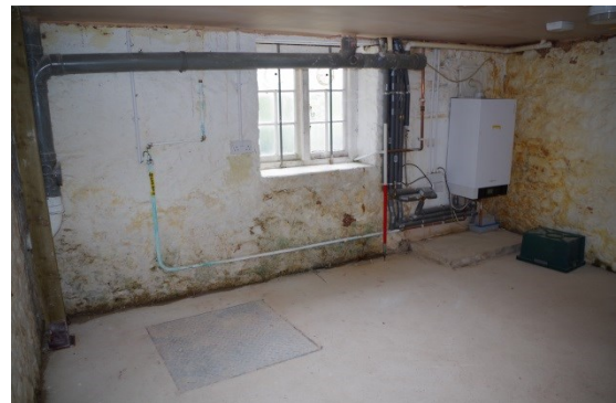
Fig 294 Lodge, room 11 looking south.
