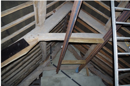
Fig 257 Roof structure above rooms 36 and 37 looking north.
