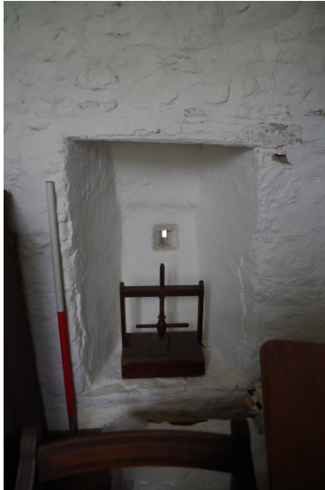
Fig 203 Room 25 squint in blocked window in west wall.
