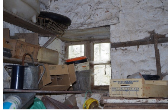
Fig 182 Room 19 window in west wall.
