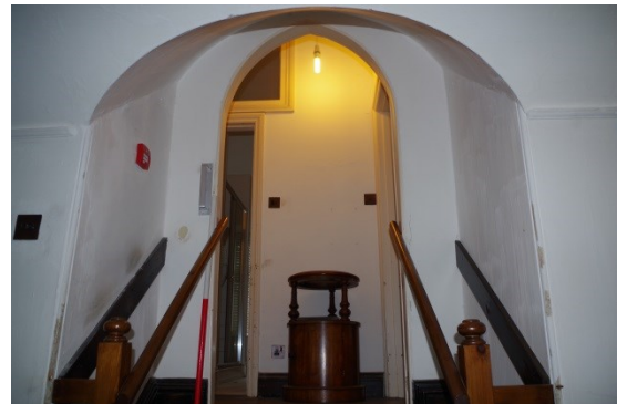
Fig 229 Room 29 arched opening cut through south wall to rooms 33 and 34.
