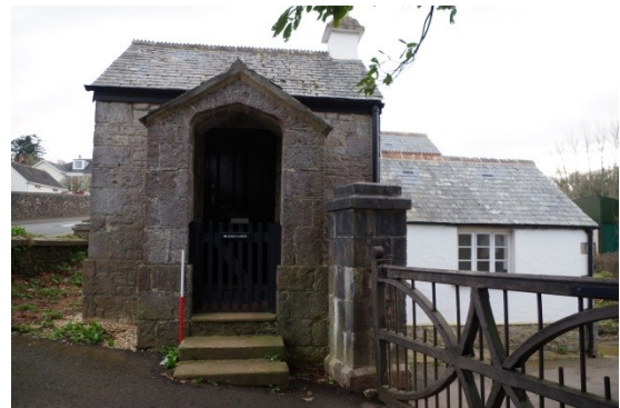
Fig 278 North elevation of Lodge porch.
