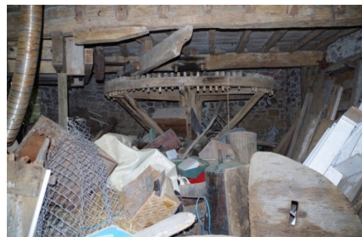
Fig 273 Pound House room 3 looking south to horse engine.
