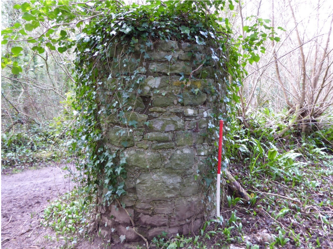
Fig 63 One of the two surviving gate piers (NT 1600095) to Culver Orchard.
