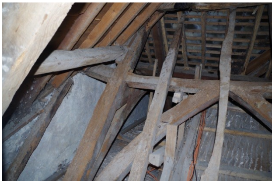
Fig 218 Exposed earlier roof over Room 27 looking north.
