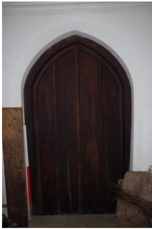
Fig 130 Room 7 (porch) looking north.
