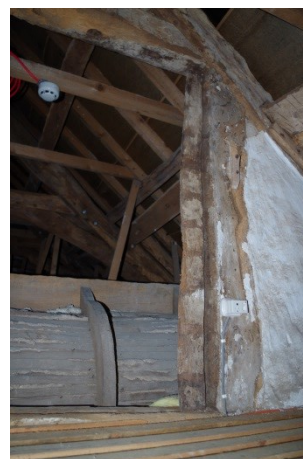
Fig 239 Attic above Room 30 timber framed wattle and daub wall to west.
