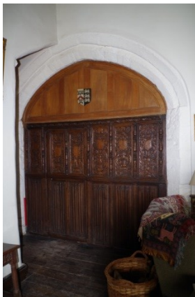
Fig 110 Room 5 arched door opening in east wall with carved screen.
