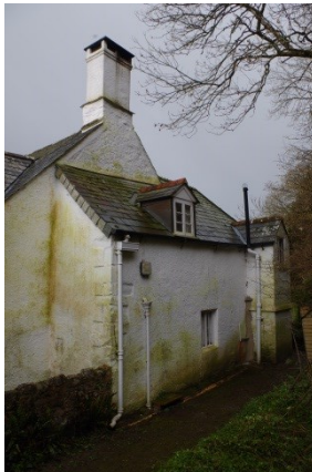
Fig 82 North elevation of East Range and extension.
