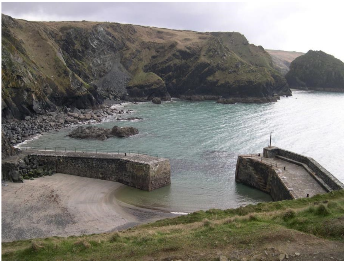
Fig 2.8 Mullion Harbour in June 2015 (Photograph: CAU).
