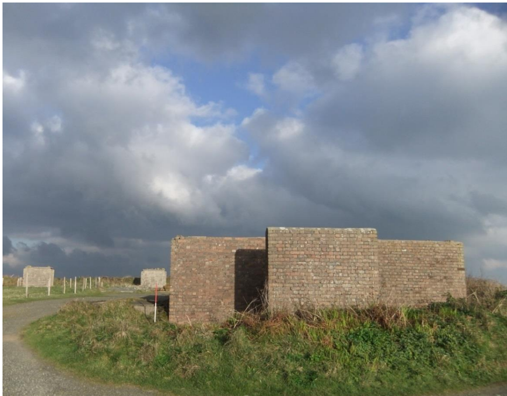
Fig 28 Post-war modification at RAF Pen Olver (Site 86), a radar station of 1941.
