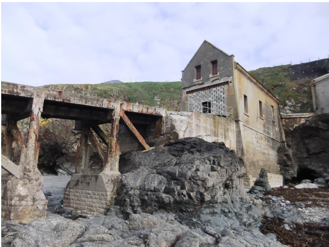
Fig 38 Lifeboat house of 1914 with dedicated slipway at Polpeor Cove (Sites P3 , P4 ).
