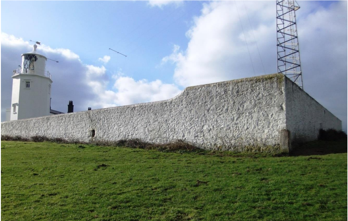
Fig 24 The north end of the east side of the Lizard Lighthouse enclosure, adjoining the NT property. The complex contains a lighthouse museum and itself shows growth, technical development and change over the centuries since its foundation c1752.
