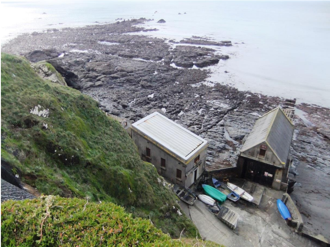
Fig 37 Successive lifeboat houses at Polpeor Cove, with the Phase 3 slipway, and the site of the turntable and earlier studio, used for small boats (Sites P3 , P4 , P6-P10 ). Note also the tidal rocks with the 'Vellan Drang' gully; and invasive purple dew plant.
