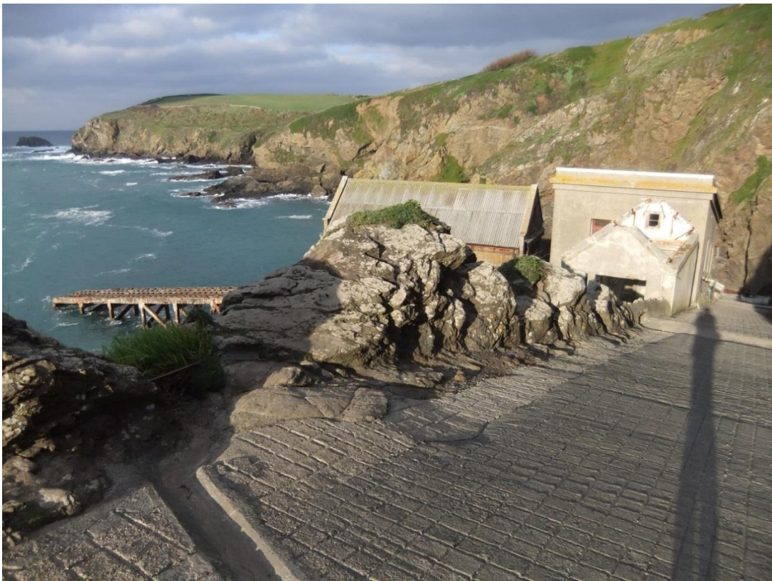
Fig 33 Rock-cut road to Polpeor Cove (Site 50), re-surfaced and partly re-cut to serve the lifeboat station from the mid-19 th century, but originating from a route of 1631.
