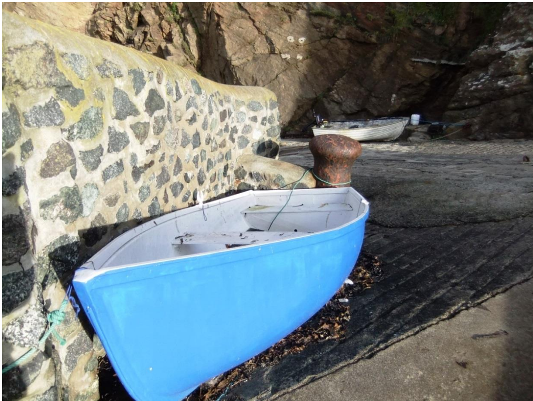
Fig 40 Sea walls, warping or mooring bollards, and expanded slipway with 'box slide' chain haulage system, features of the Polpeor Cove lifeboat station (Sites P6 , P7 ).
