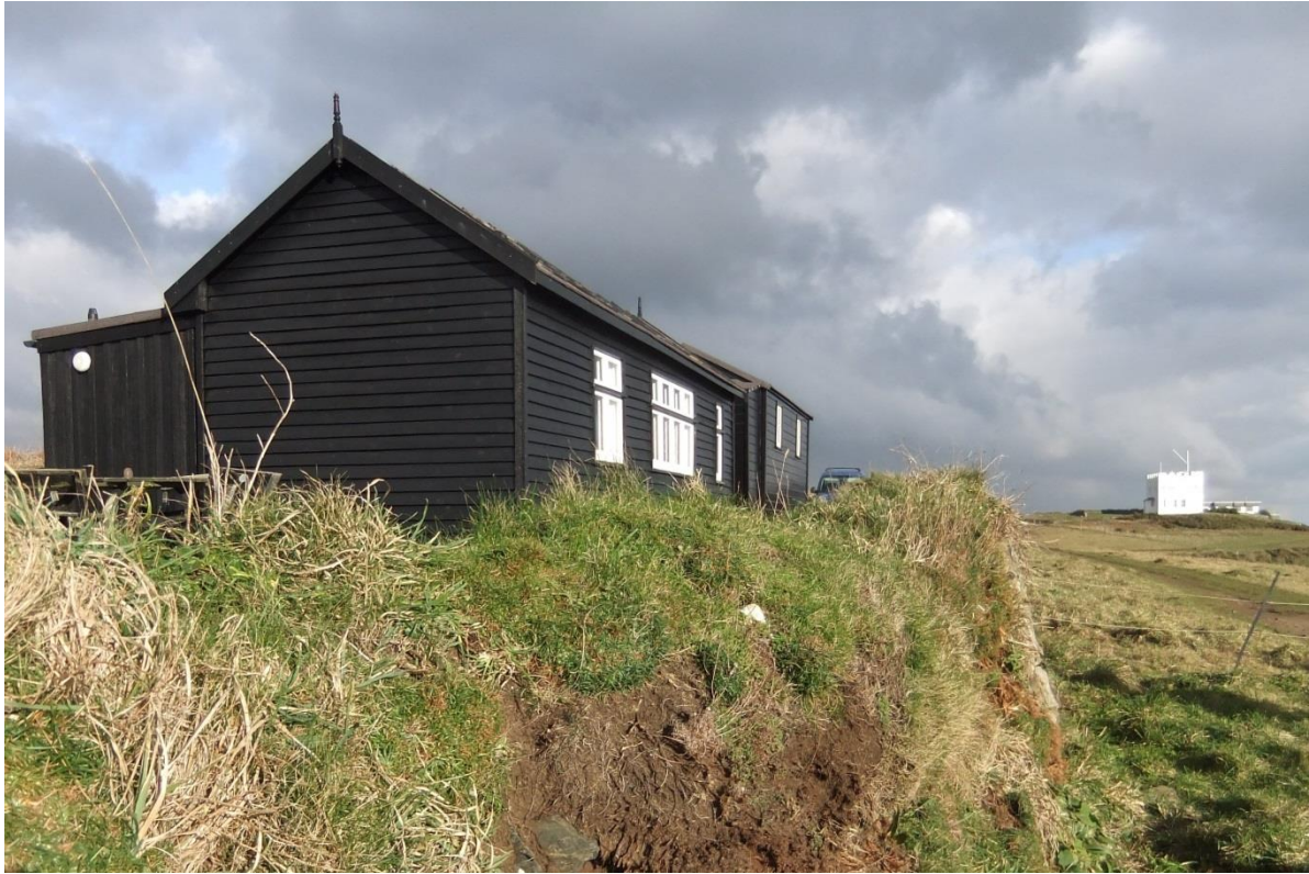
Fig 32 Marconi's Lizard Wireless Telegraphy Station of 1900 at Pen Olver (Sites 90, 91), with the Lloyd's (originally Fox's) Signal Station of 1872 beyond (Site 100).
