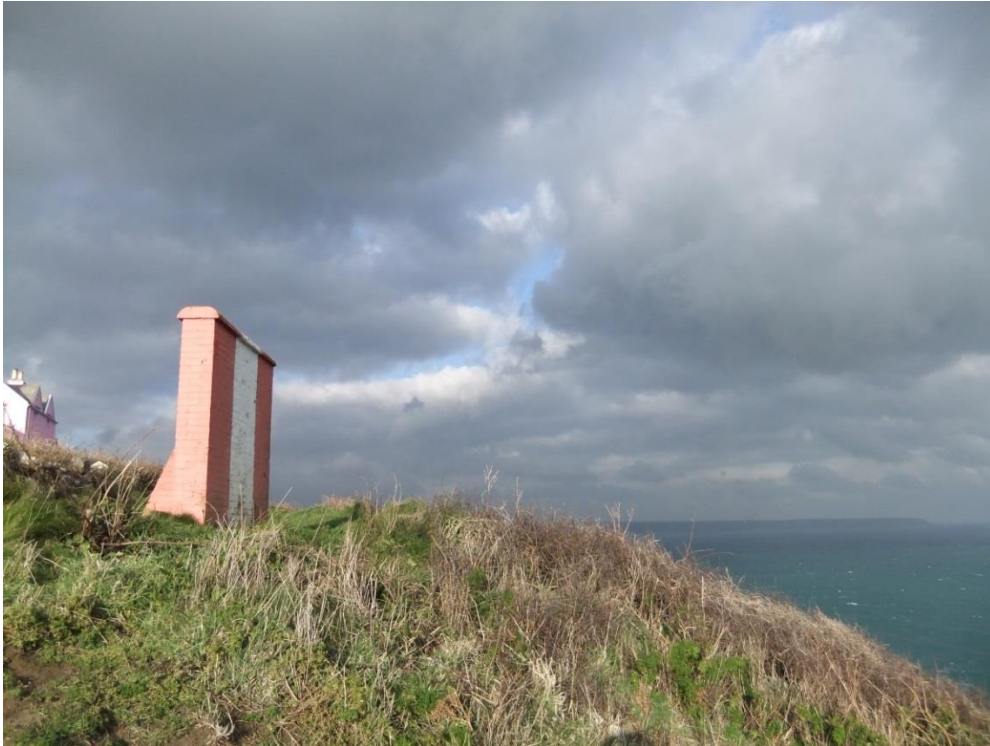
Fig 26 Daymark at Site 99, Bass Point, part of the infrastructure warning mariners of the submerged rock, the Vroque, where the Czar steamer was lost in 1859.
