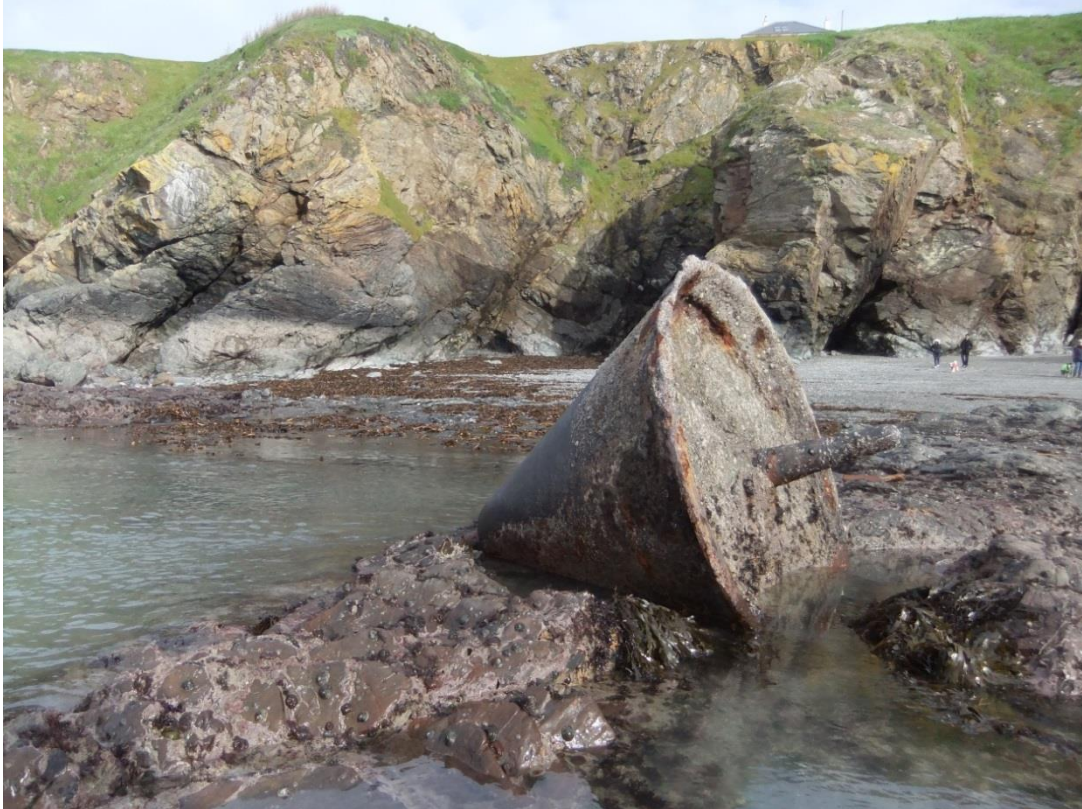
Fig 39 Fallen buoy at Polpeor Cove marking a passage over the shore, part cut into the tidal rocks, probably used to launch and recover the lifeboat in Phase 2, and as an outhaul only in Phase 3 when the lifeboat house had its own launching slip (Site P5 ).
