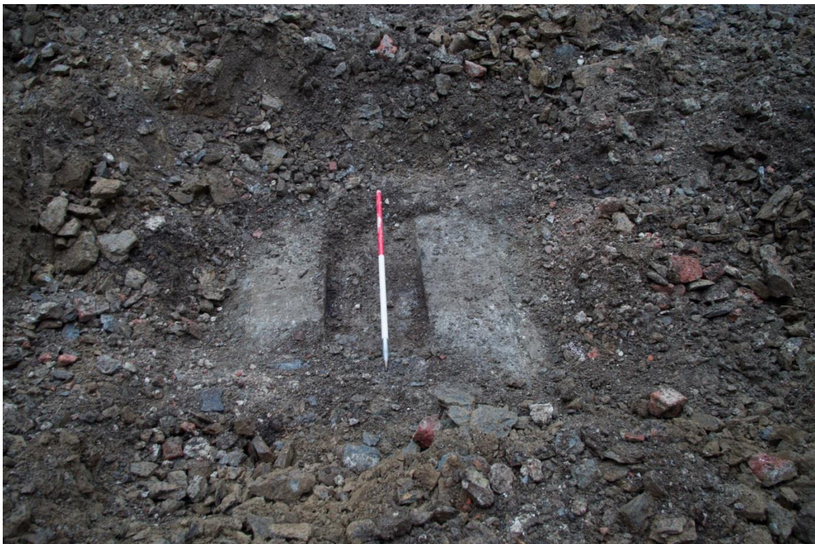
Figure 14 Block D, Horse engine house (Room 32) – Looking north west to the footings beneath the removed mellior stone.
