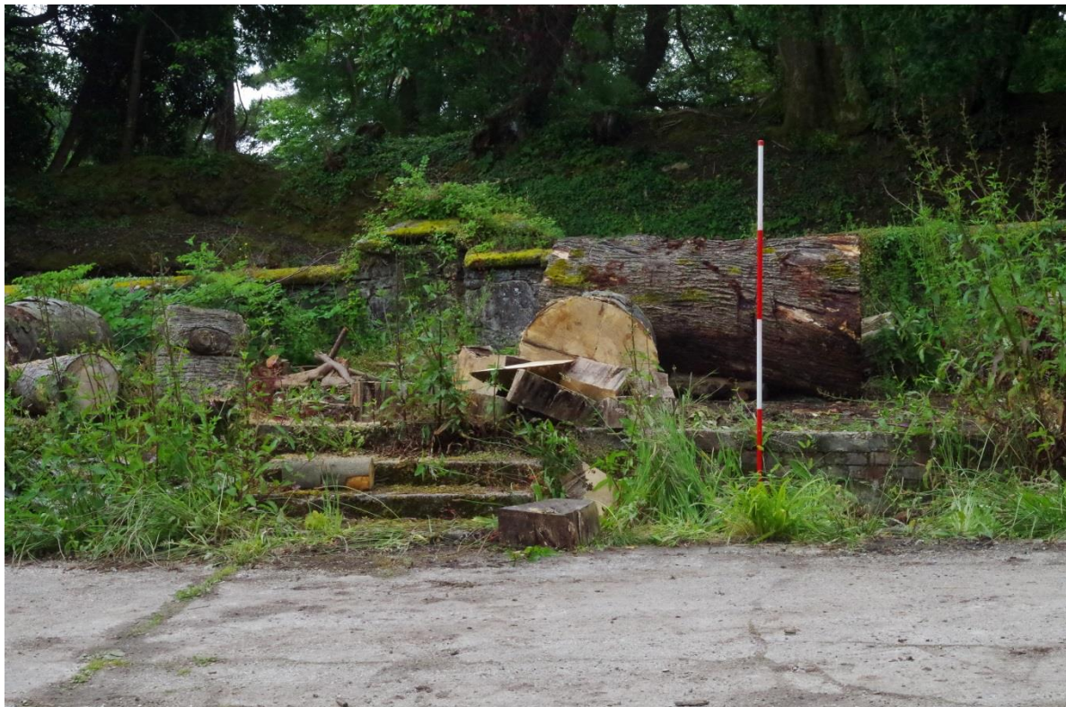
Figure 10 Rickyard – Building platform 9 showing the steps on the north wall.
