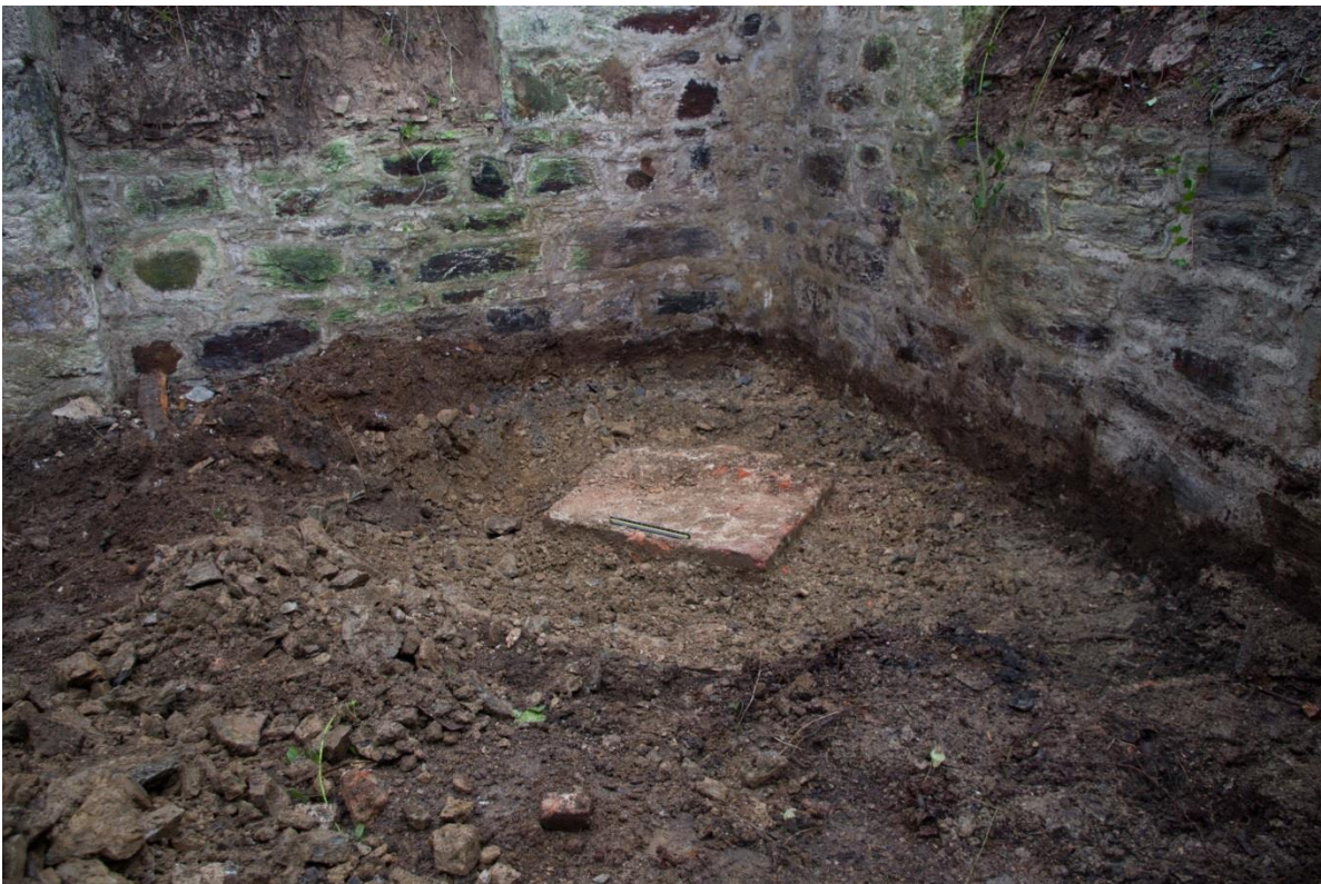
Figure 12 Block D, Horse engine house (Room 32) – Looking north to the surviving footings of the brick-built pillar for the earlier horse-engine house.
