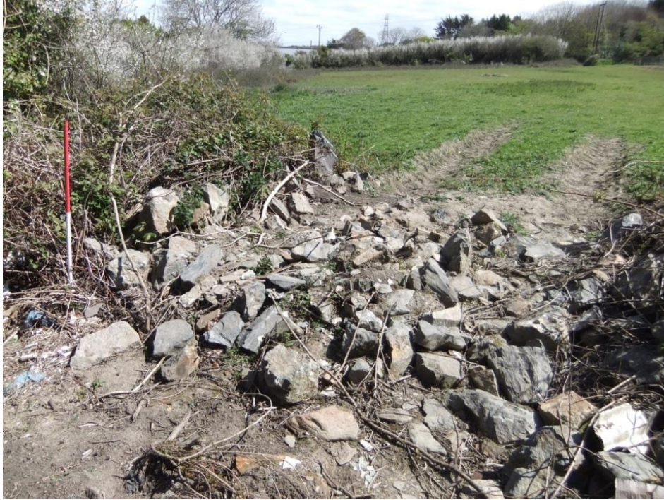
Fig 9 Recent damage on east of yard Site 6, with tracks aligned towards dump Site 10.
