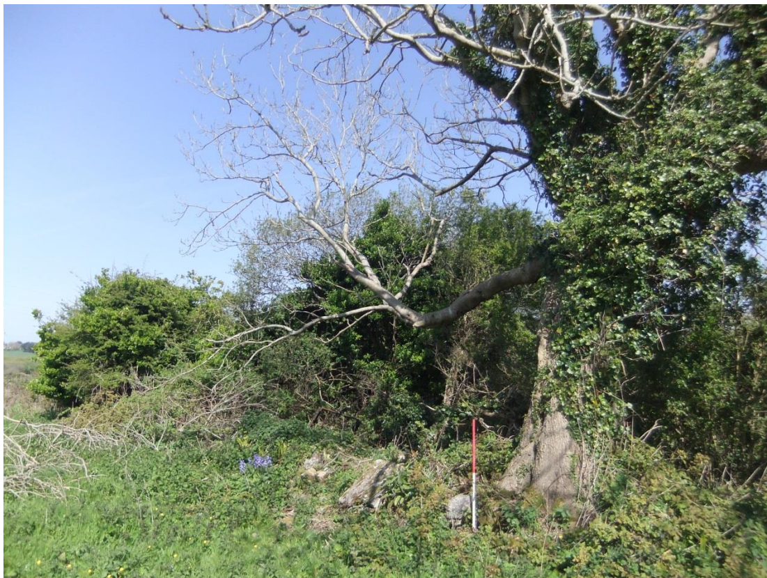
Fig 5 Bank west of cottage Site 3, with old ash tree, and possible well cover left of this.
