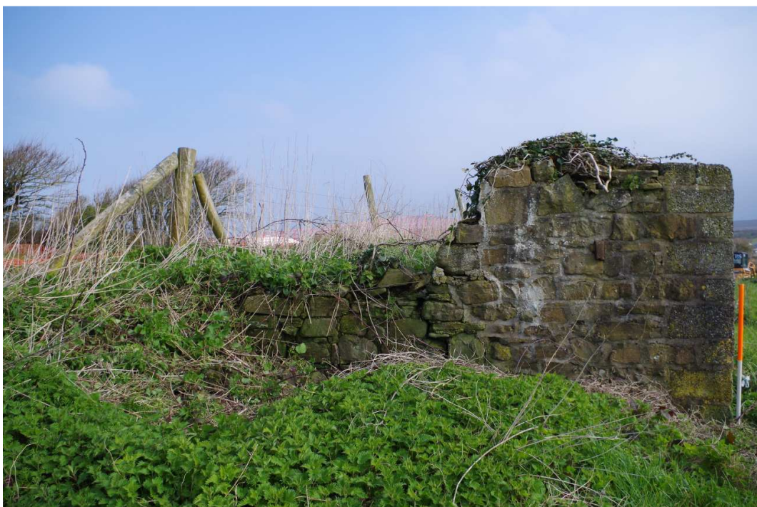
Figure 18 West facing elevation of Structure 1, Field 2, looking east.
