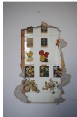
Fig 38 Quadrangle: example of tiles in science lab (room 51).
