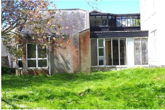
Fig 55 Link Building: East elevation.
