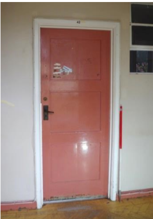
Fig 41 Quadrangle: example of three panel door (room 43).
