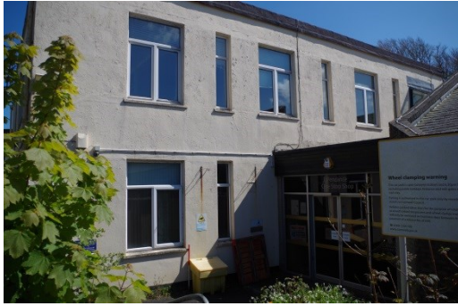
Fig 16 Quadrangle: South-west range, west elevation.
