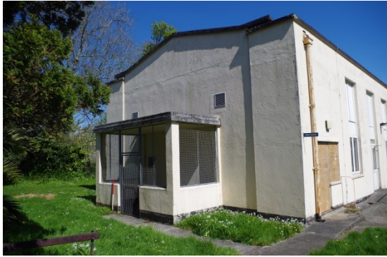
Fig 8 Quadrangle: North range, west elevation.
