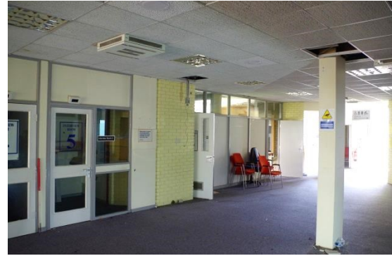
Fig 59 Link Building: Reception (room 61) looking south-east.
