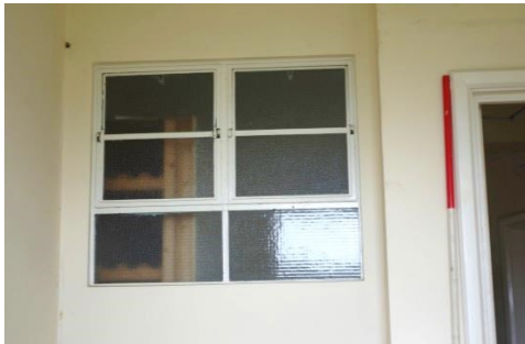
Fig 48 Quadrangle: example steel frame borrowed light to stairs (room 19).
