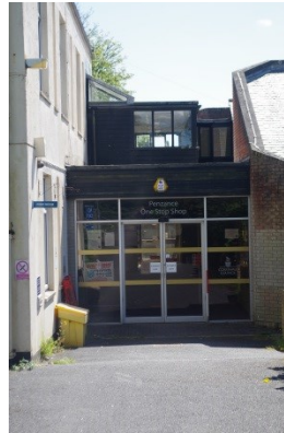
Fig 52 Link Building: North elevation main entrance.
