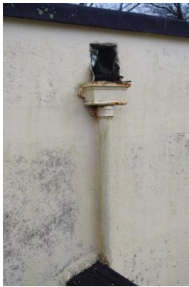
Fig 17 Quadrangle: cast iron down pipe.
