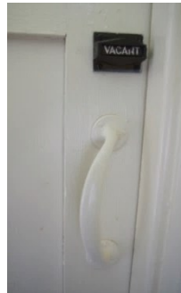
Fig 45 Quadrangle: example of cubicle door handle and lock (room 39).
