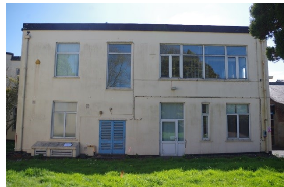
Fig 13 Quadrangle: South-west range, north elevation.
