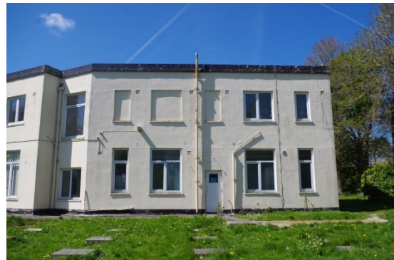
Fig 6 Quadrangle: North range, east elevation.
