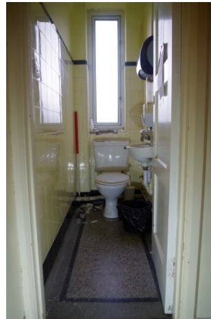
Fig 21 Quadrangle: example of toilet (room 37).
