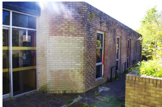
Fig 53 Link Building: North elevation.
