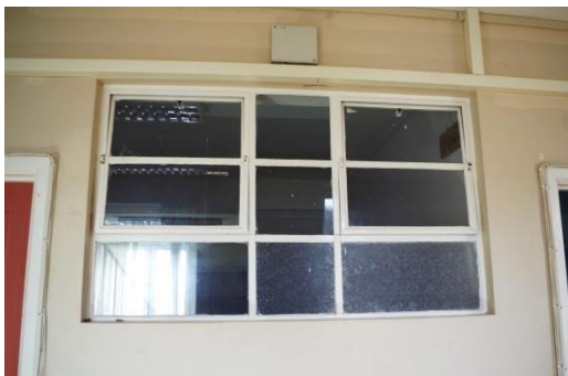
Fig 49 Quadrangle: example steel frame borrowed light (room 43).
