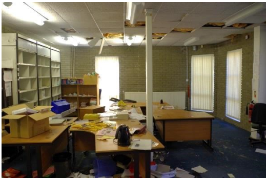
Fig 64 Link Building: Office (room 71) looking west.
