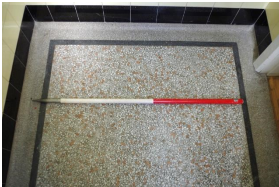
Fig 24 Quadrangle: example of terrazzo floor in toilets and bathrooms.
