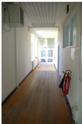
Fig 25 Quadrangle: narrow board floor in first floor corridor (room 54).
