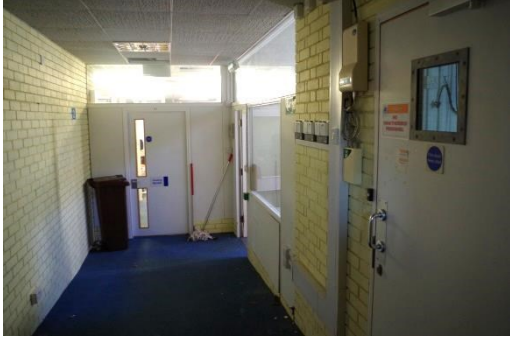
Fig 63 Link Building: Corridor (room 70) looking north.
