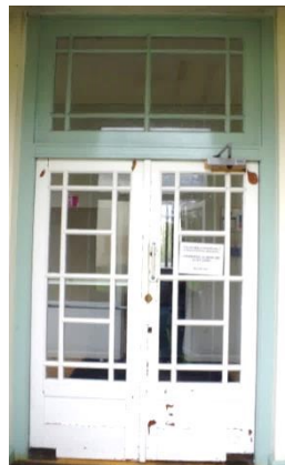
Fig 46 Quadrangle: internal porch doors (room 14).
