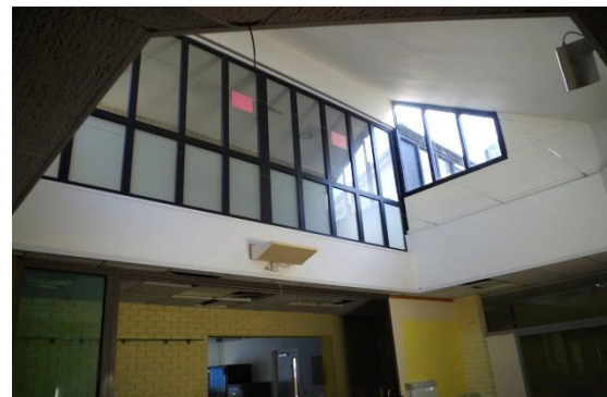
Fig 61 Link Building: Reception (room 61) looking up to link corridor.
