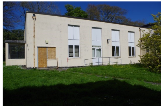
Fig 7 Quadrangle: North range, south elevation.
