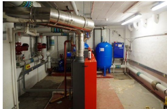
Fig 22 Quadrangle: Boiler room (60) looking north.
