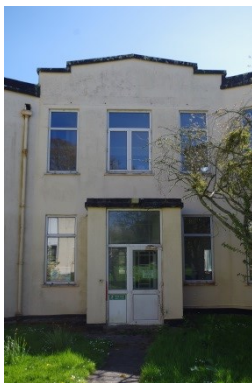
Fig 11 Quadrangle: South-east range, north-west elevation and porch.
