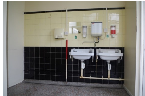
Fig 36 Quadrangle: example of tiling and sinks in toilets (room 5).
