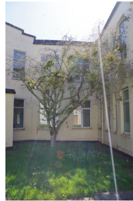
Fig 12 Quadrangle: South-west range, north elevation.
