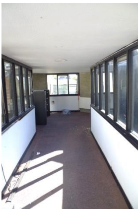
Fig 66 Link Building: Link passage (room 72) looking south.
