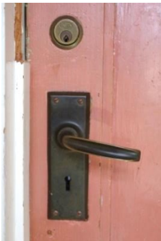
Fig 42 Quadrangle: example of brass door handle (room 43).
