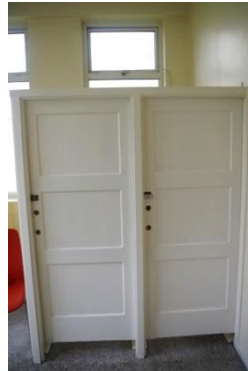
Fig 44 Quadrangle: example of cubicle doors (room 5).
