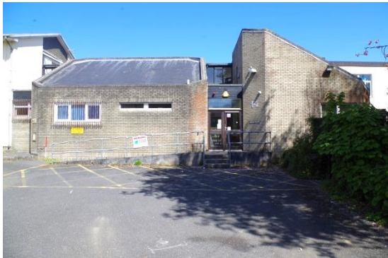
Fig 56 Link Building: South elevation.
