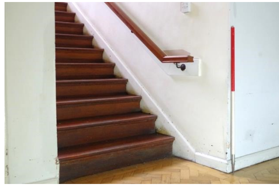
Fig 27 Quadrangle: stair detail.
