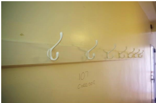
Fig 33 Quadrangle: peg rail in room 34.
