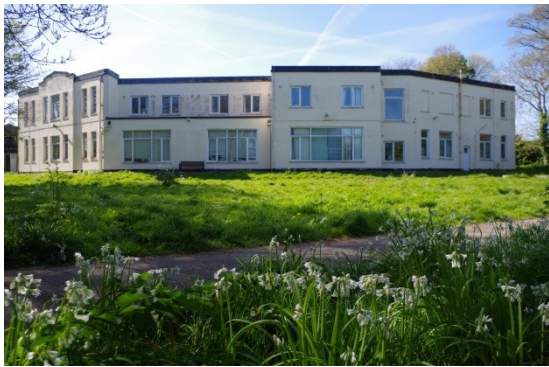
Fig 9 Quadrangle: South-east range, south-east elevation.
