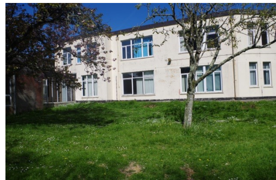
Fig 15 Quadrangle: South-west range, south elevation.
