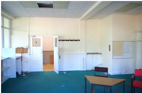
Fig 18 Quadrangle: example of classroom (room 58).
