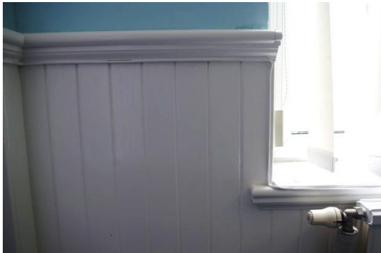
Fig 32 Quadrangle: detail of wall panelling and dado rail (room 9a).
