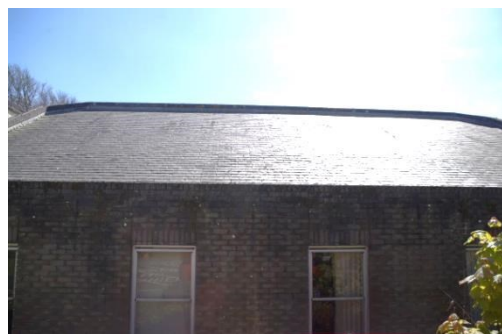
Fig 54 Link Building: North elevation roof.
