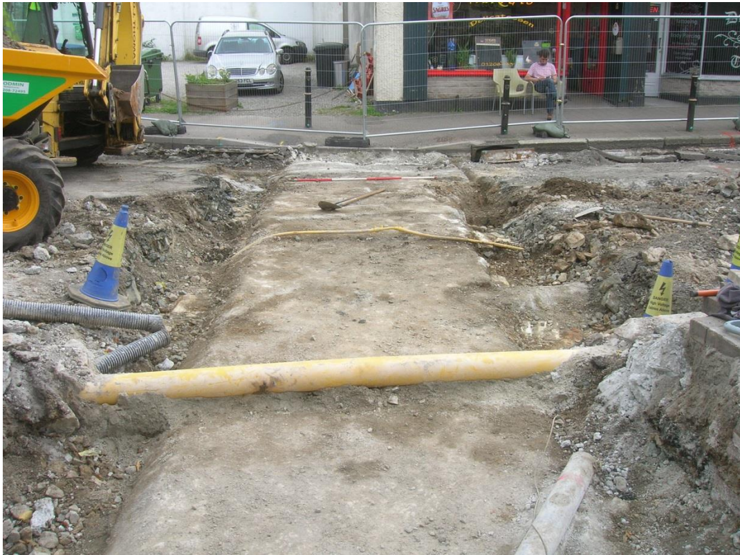
Figure 14. Scheme 5. Church Square. Bodmin Town Leat looking south east showing concrete capping.
