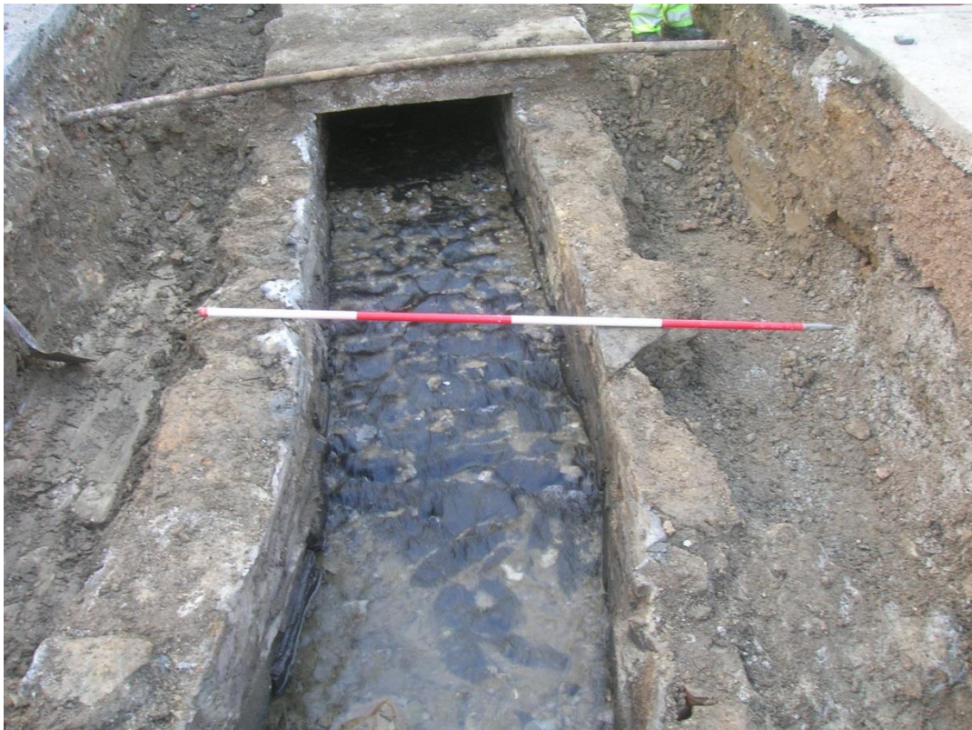
Figure 19. Scheme 5. Bodmin Town leat in Dennison Road, looking south east showing cobbled floor.
