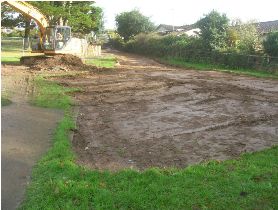
Figure 20. Scheme 9. Priory Park. The area topsoil stripped for cycle path looking north east.
