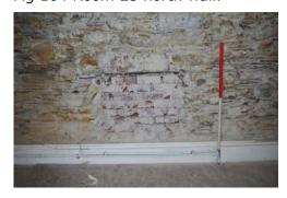
Fig 105 Room 25 blocked fireplace in north wall.
