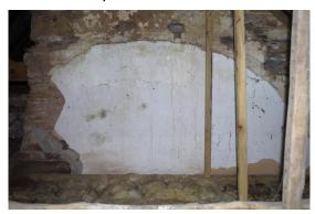
Fig 97 Room 22 roof space showing evidence for removed barrel ceiling on west wall.
