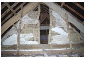
Fig 102 Room 23 partition in roof space between landing and room 23 (west wall) with later cornice for a barrel ceiling.
