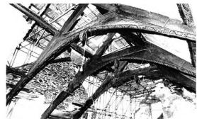
Fig 22 Room 3 roof taken after the 1990s fire looking south-east.
