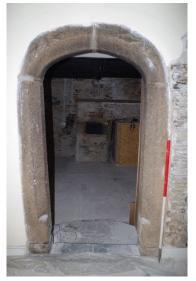
Fig 18 Room 2 Granite door opening in south wall.
