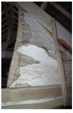
Fig 103 Room 23 showing remains of moulded cornice for barrel ceiling on west wall.
