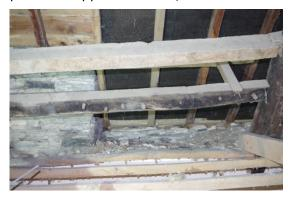
Fig 98 Room 23 roof space showing original multi-pegged purlin to north.
