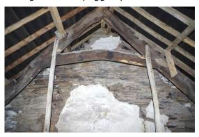
Fig 99 Room 23 roof space showing original cranked collar truss.
