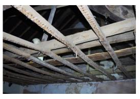
Fig 101 Room 23 showing battens for removed lath and plaster ceiling.
