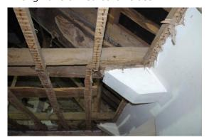
Fig 100 Room 23 roof space showing foot of principal rafter to south indicating location of original south wall.
