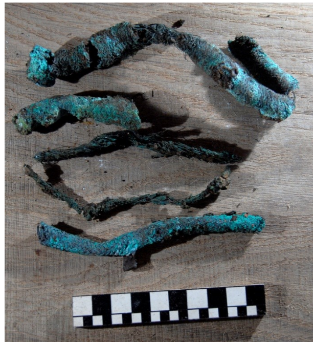
Fig 16. Smaller diameter sections of woven armoured cable sheathing.
