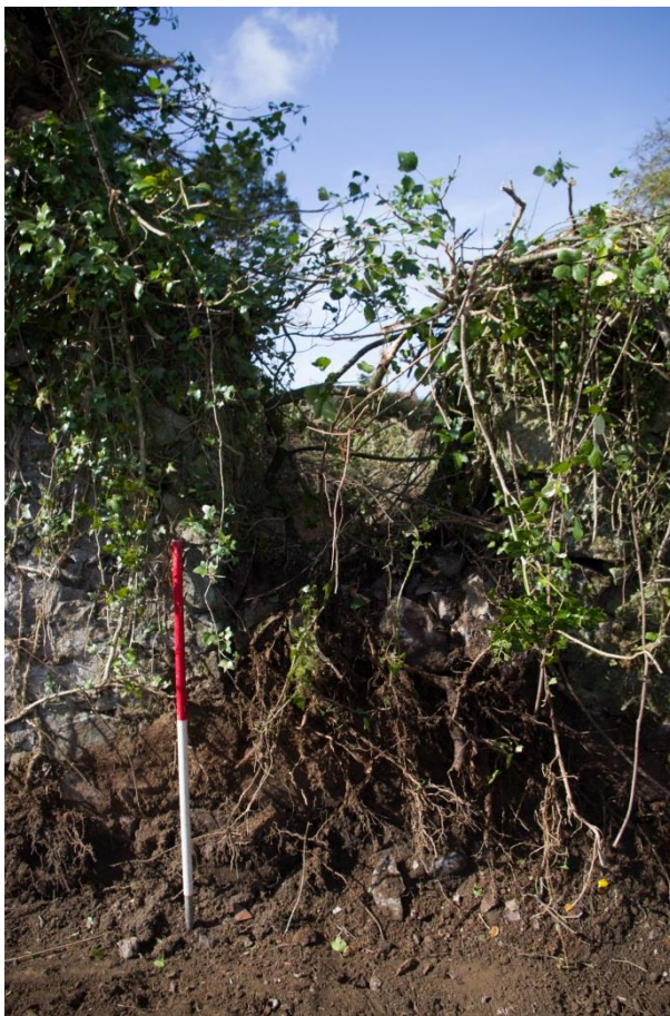
Figure 20. Window opening in east wall Structure 2, room 1.
