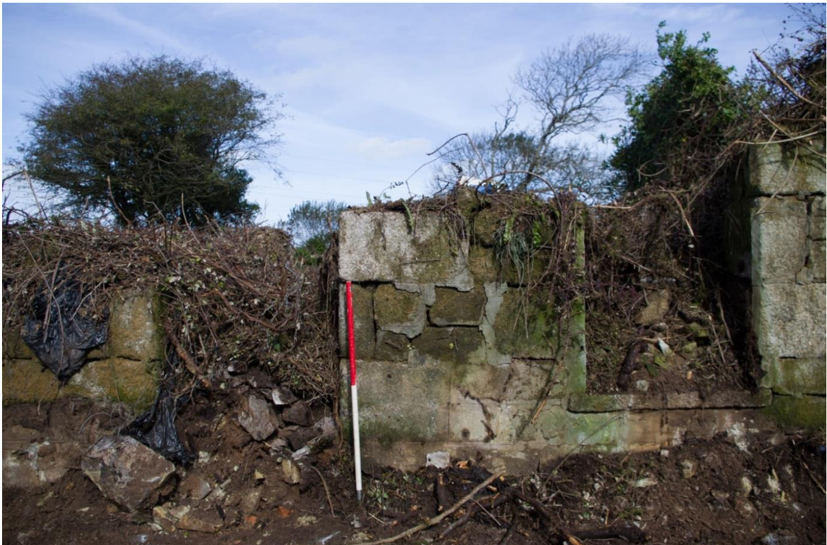
Figure 23. Southern external elevation of Structure 2, room 2 showing window opening with surviving cill and nearby doorway.
