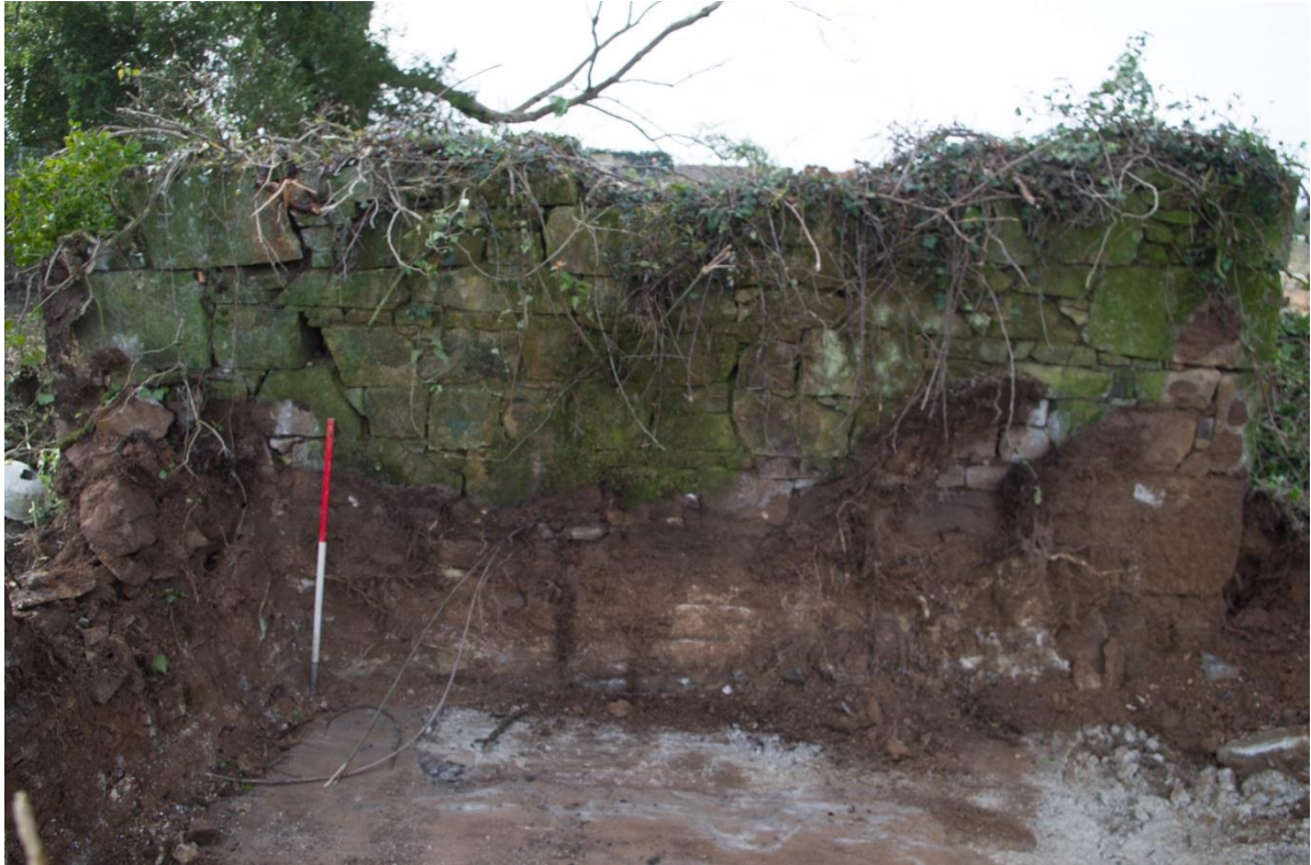
Figure 26. Eastern internal wall face of Structure 2, room 3.
