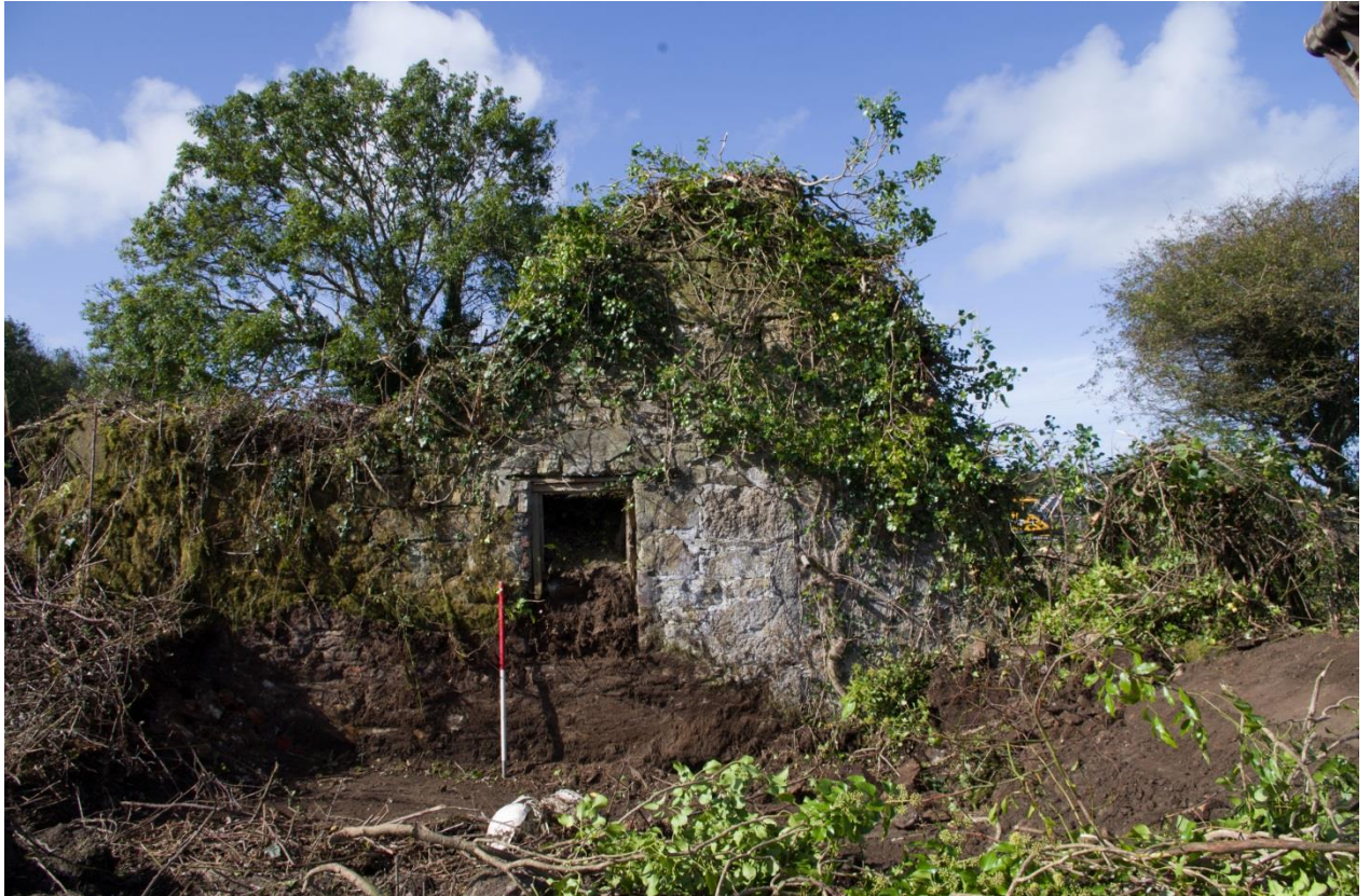
Figure 19. East-facing gable, Structure 2.
