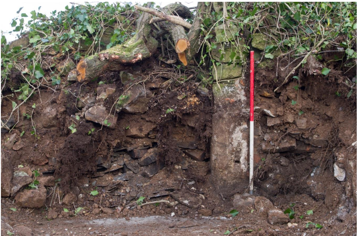
Figure 37. East wall of Structure 2, room 7 showing extensive collapse.
