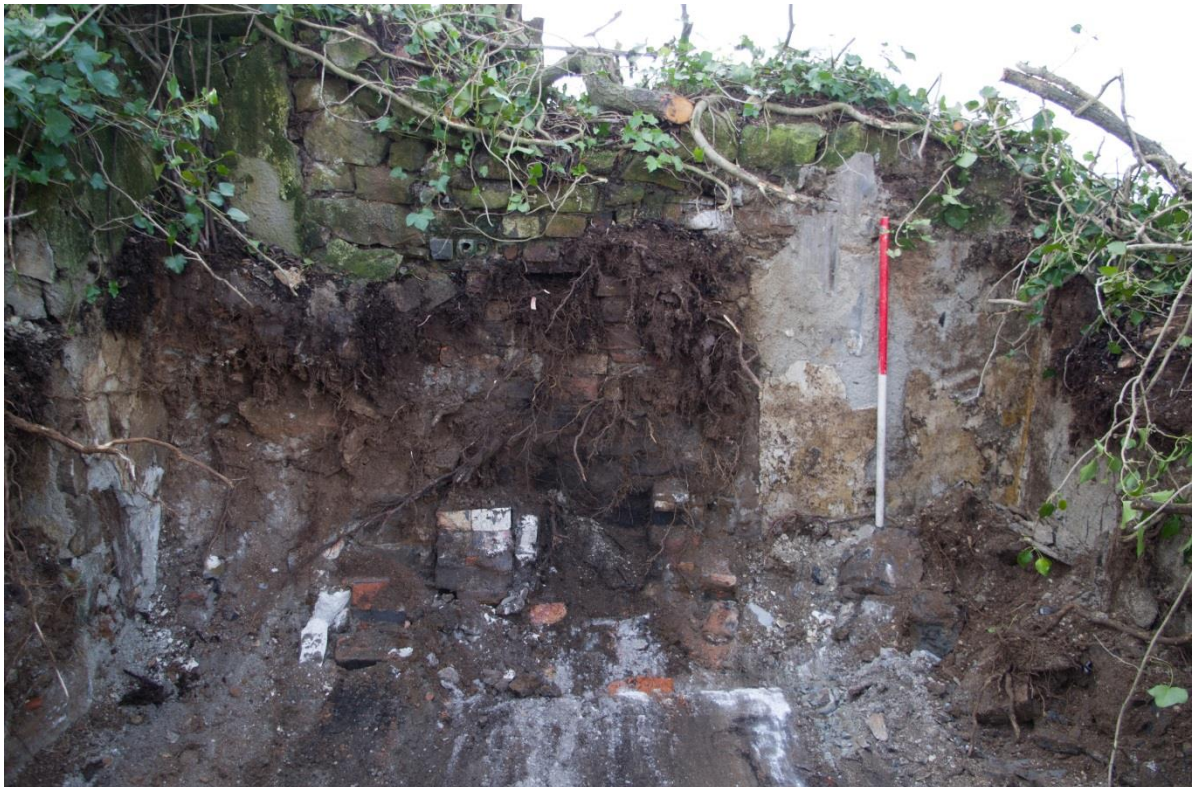
Figure 27. Eastern internal wall face of Structure 2, room 4 showing removed fireplace or range and surviving plaster.
