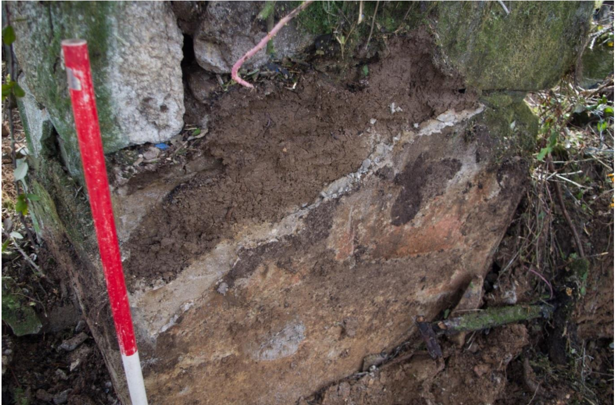
Figure 22. Plaster detail in south wall Structure 2, room 3.
