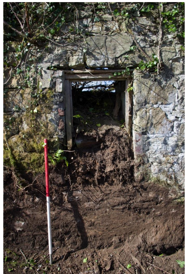
Figure 21. Window opening in east wall Structure 2, room 2.
