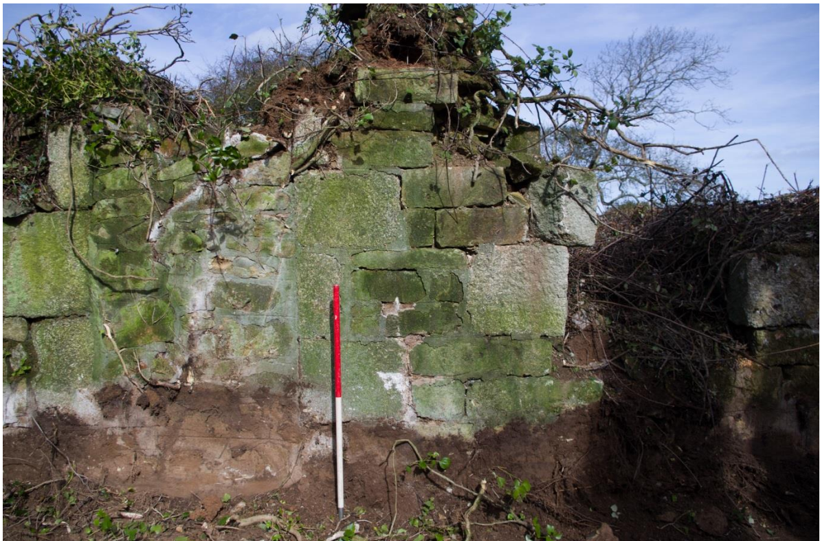
Figure 25. External southern elevation of Structure 2, room 3 showing blocked doorway and window opening.
