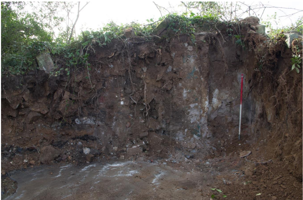
Figure 34 West wall of Structure 2, room 6 showing surviving plaster and fireplace side pillar.
