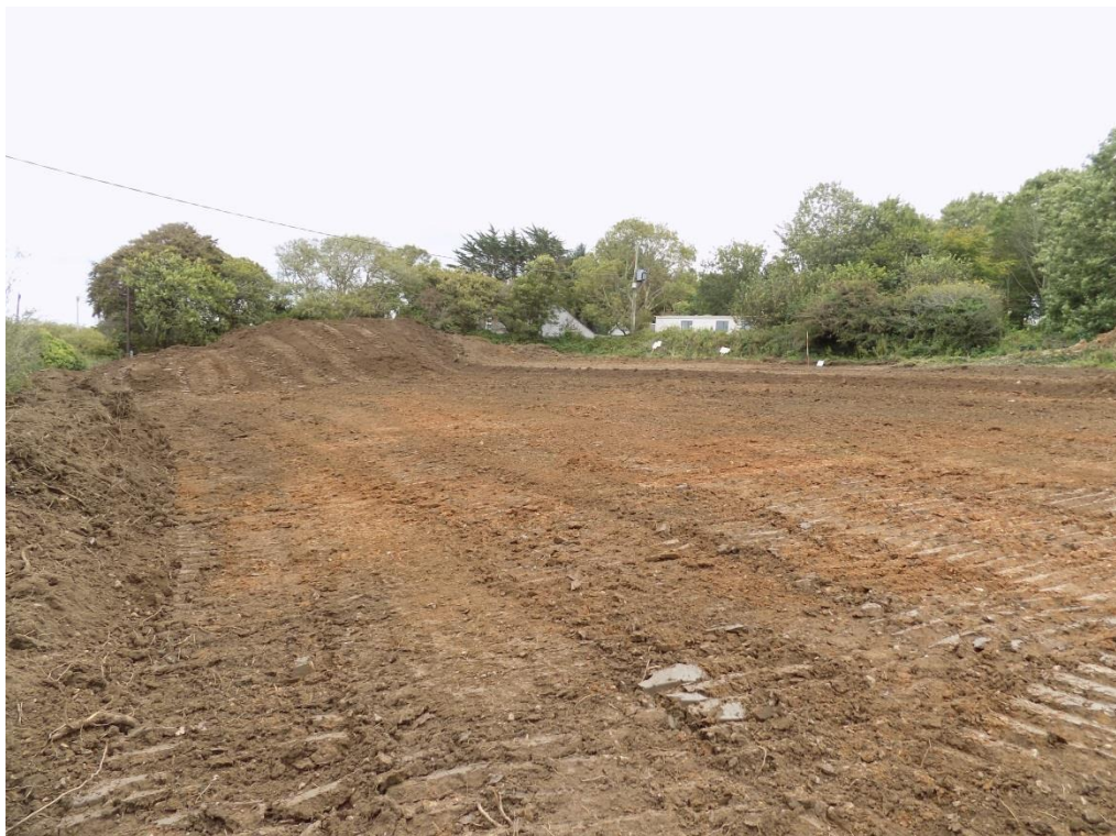
Figure 10. Field 1. A general overview after the topsoil strip looking southeast.
