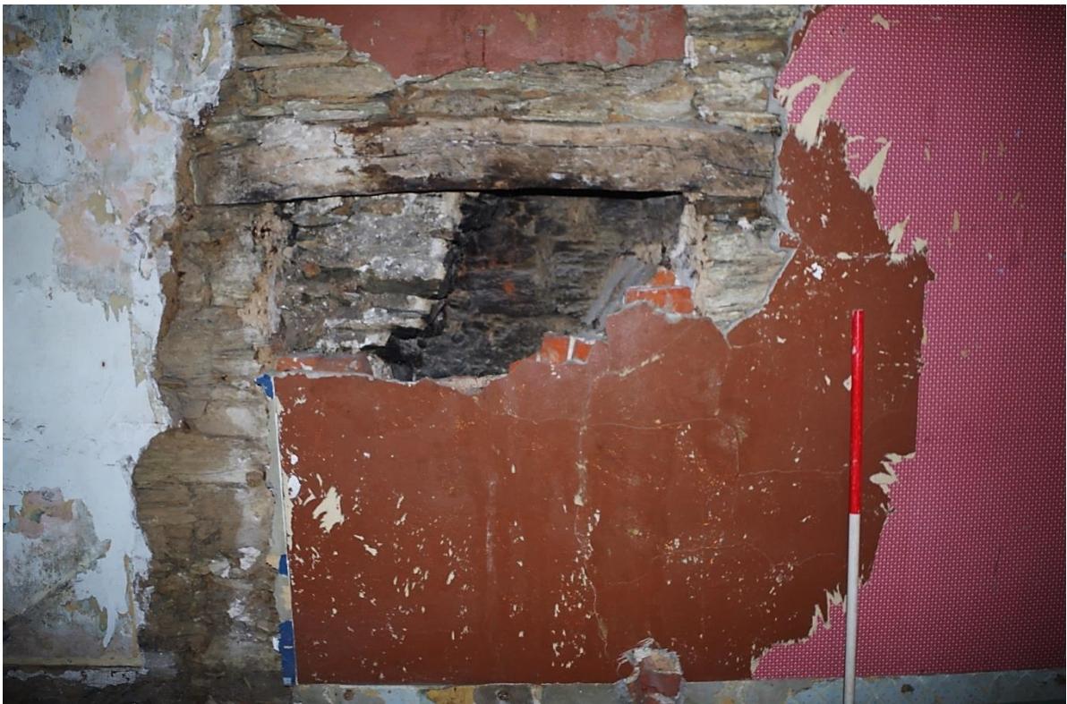
Fig 29 Second floor north-east wall in the Front Range showing original blocked fireplace with timber lintel.
