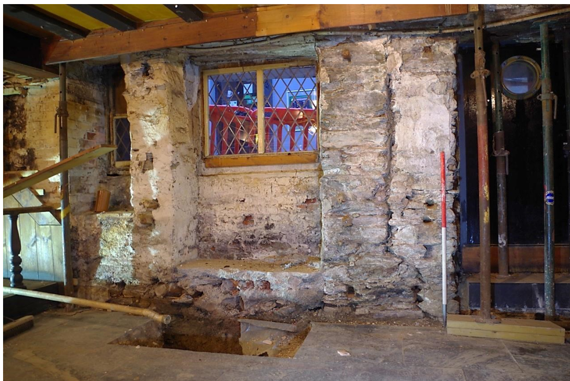
Fig 20 Ground floor north-west wall showing original, blocked front door opening.
