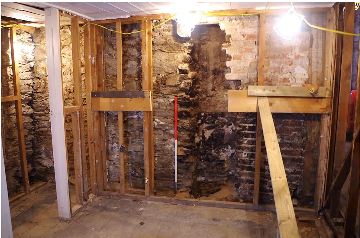
Fig 27 First floor phase 1 north-east wall in the Front Range showing original fireplace blocked with brickwork to the south-east.
