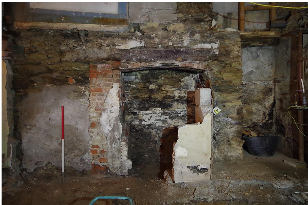
Fig 30 Ground floor south-west wall in the Front Range showing large fireplace blocked with brickwork to the south-east.
