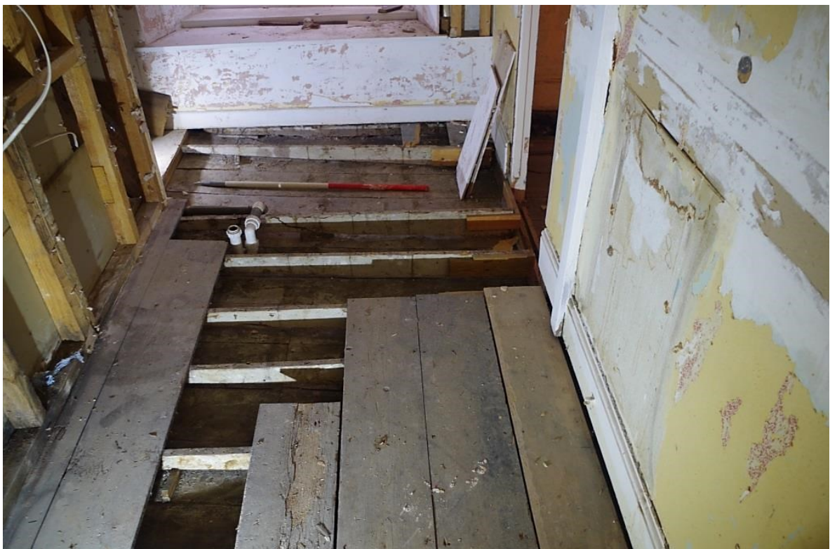
Fig 45 Room 10 (Bathroom): floorboards (2) overlying earlier floor (1).
