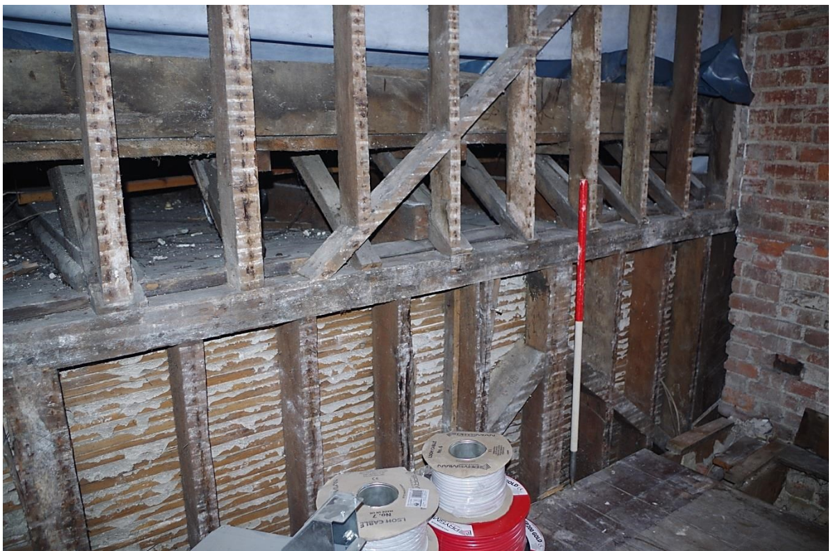
Fig 49 Late 17th or 18th century second floor wall and roof of the narrow range which runs along the rear north-east side of the building. The upper studwork was added in the 19th century to raise the height of the rest of the rear range (looking east).
