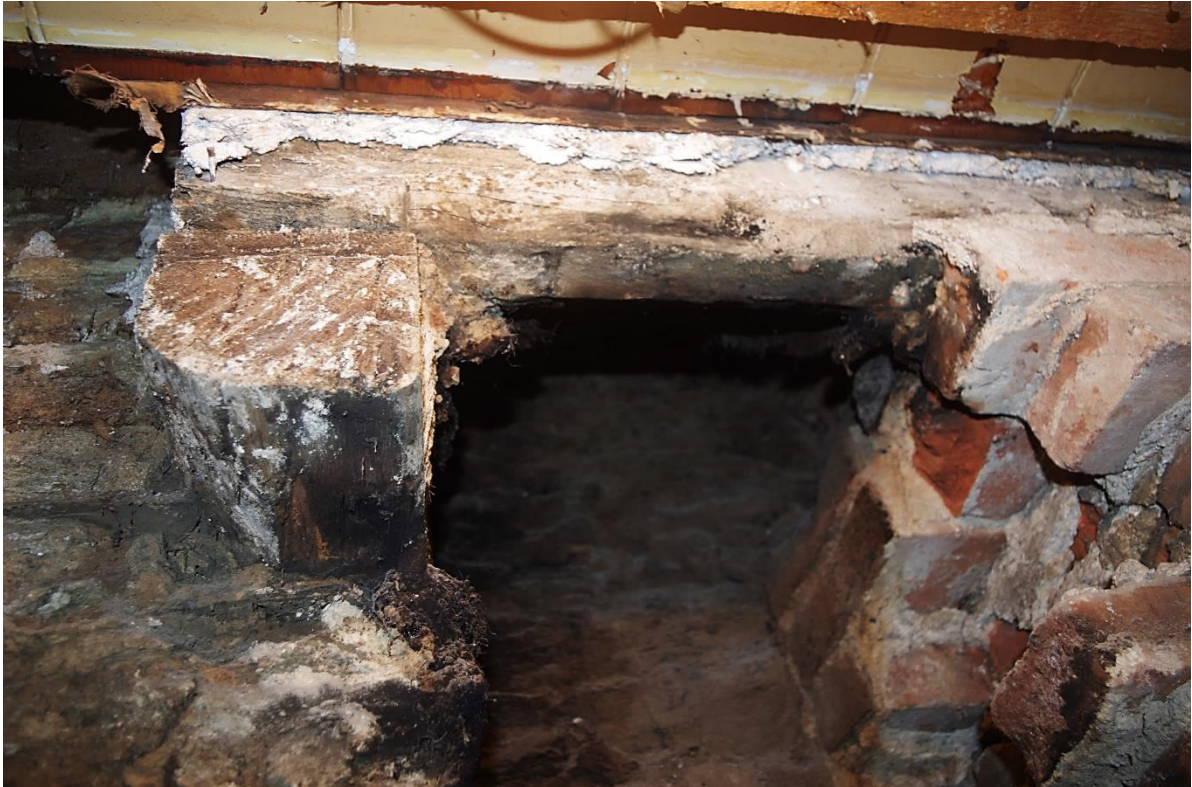
Fig 28 First floor north-east wall in the Front Range showing chamfered lintel with ogee stops over original fireplace blocked with brickwork to the south-east.
