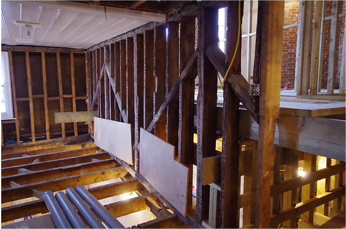
Fig 50 Late 17th or 18th century studwork of second floor wall in room 13. (looking south).
