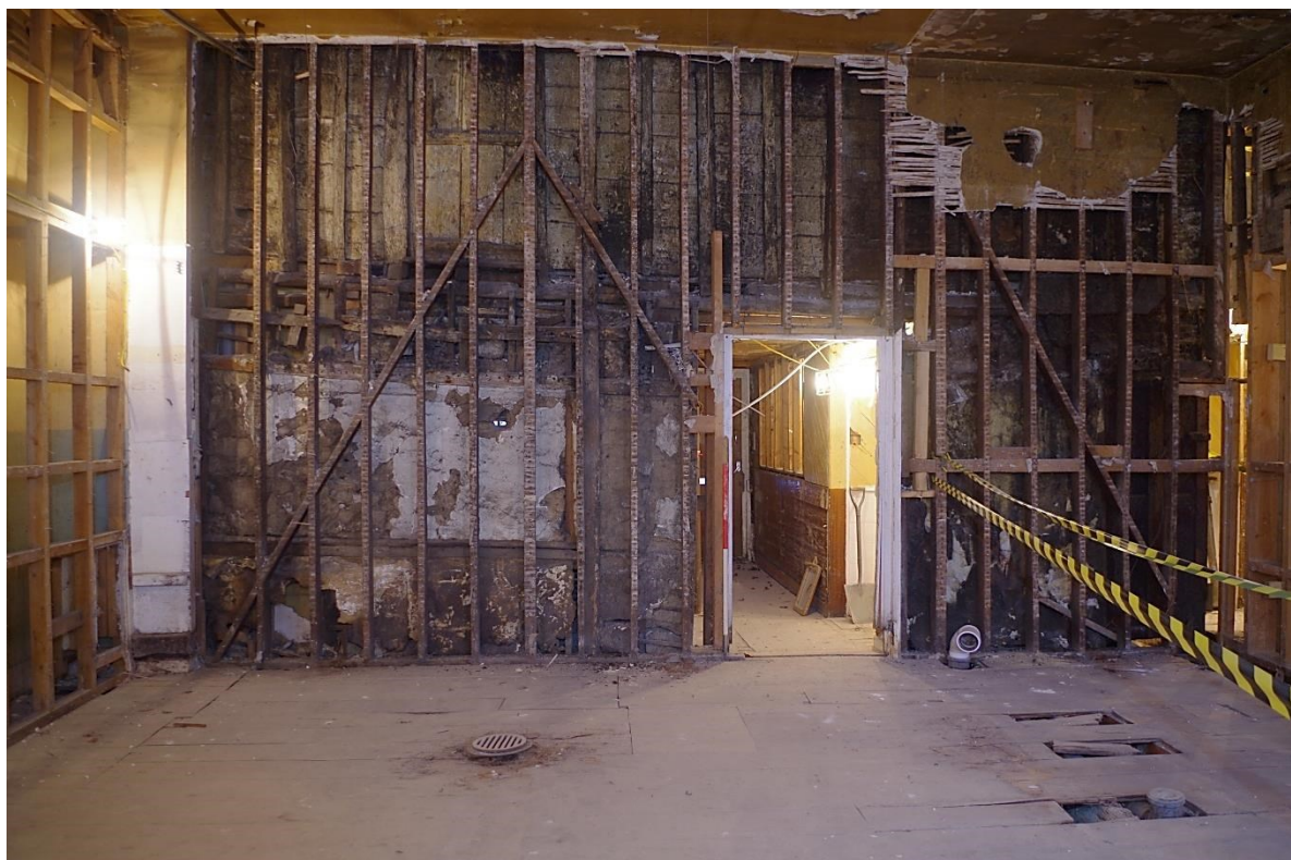
Fig 33 South-east elevation of partition wall showing original first and second floor levels.
