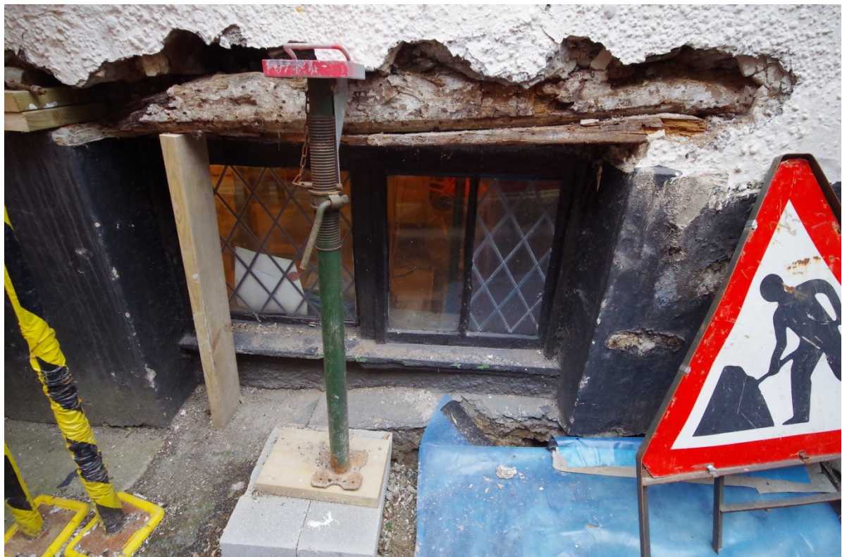
Fig 18 Exposed, moulded lintel with later lintel inserted below it for support above ground floor window in north-west (front) elevation of the Chain Locker.
