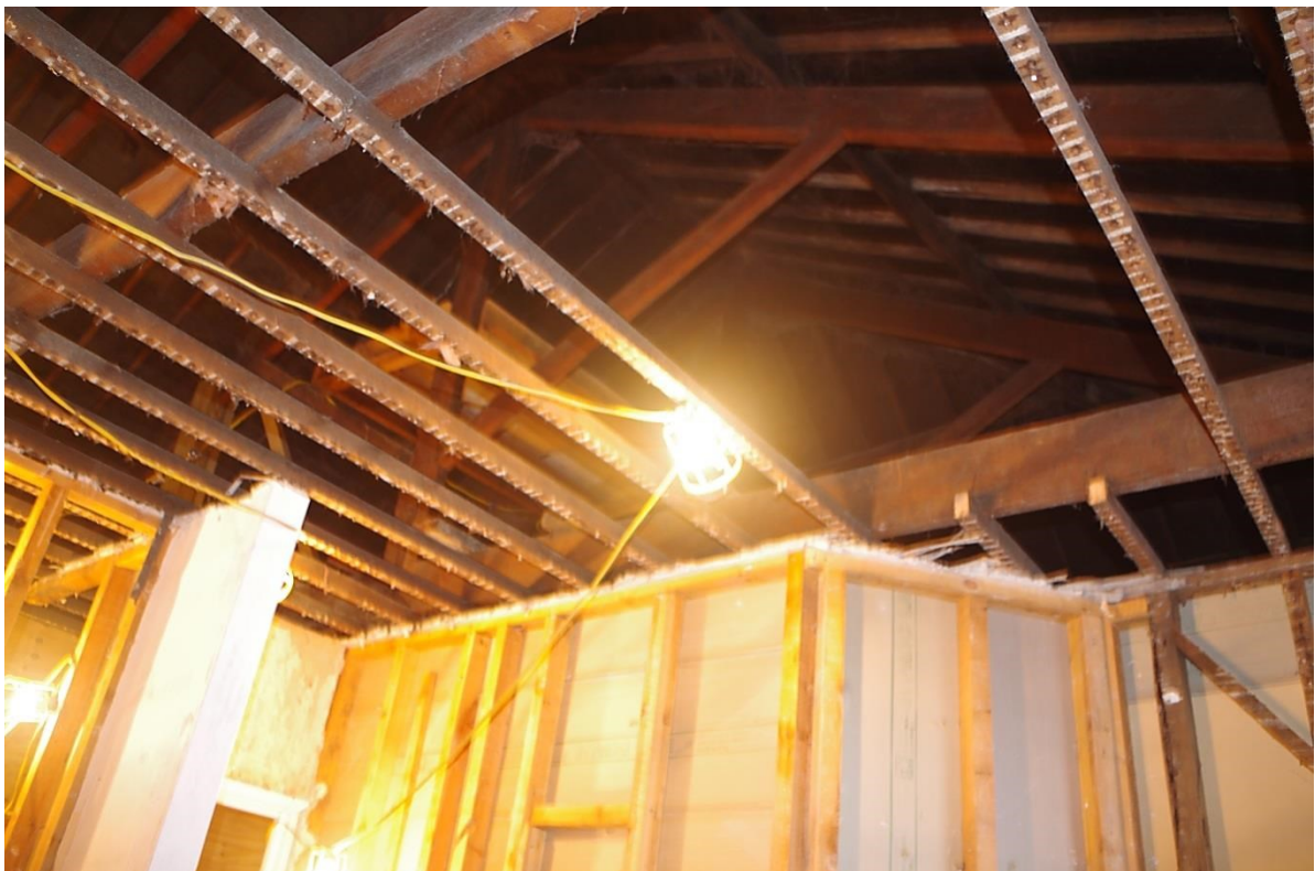
Fig 47 19th century replacement king post roof structure over the higher Rear Range looking north-east.
