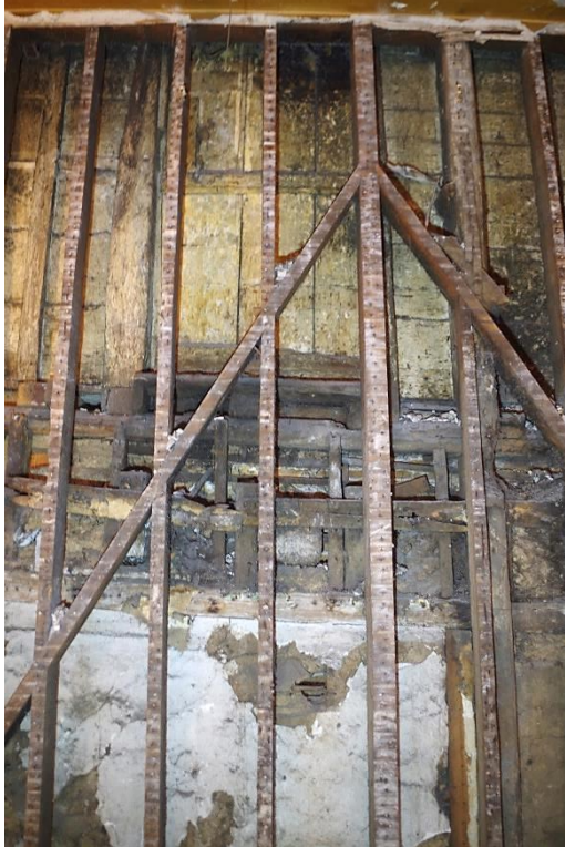
Fig 35 Partition wall, showing ledgered door and plank walling at second floor level and lath and earth plaster walling below at first floor level- both behind later studwork.
