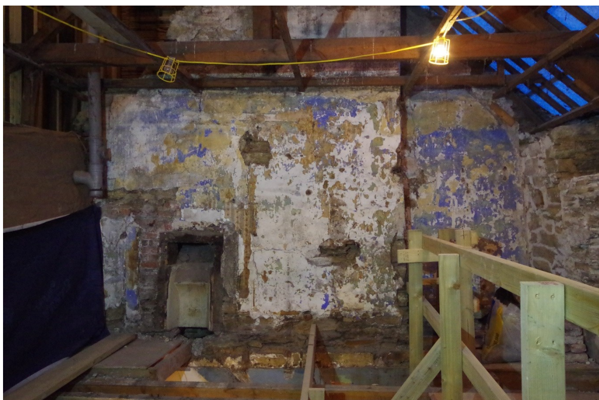
Fig 31 Second floor south-west wall in the Front Range showing fireplace blocked with brickwork to the south-east.
