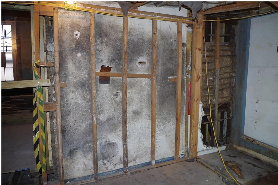
Fig 36 North-west elevation of partition wall at first floor level showing lath and earth plaster to right.
