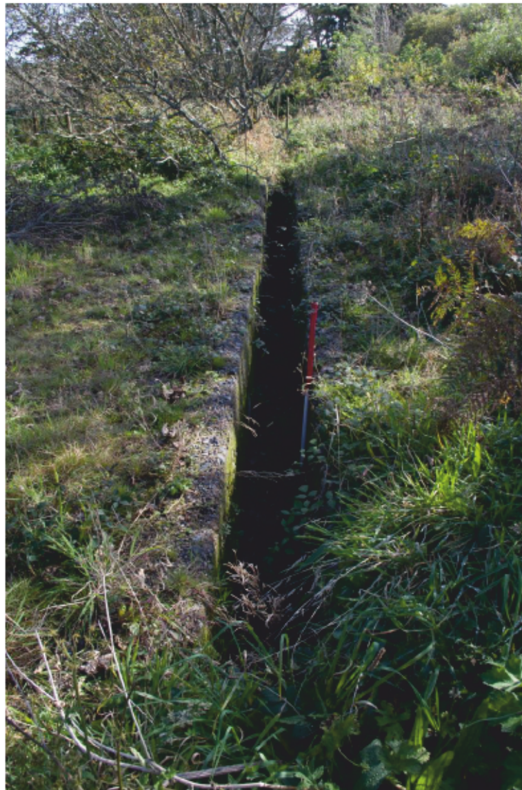
Fig 10 The water channel, or flue (facing SSE).
