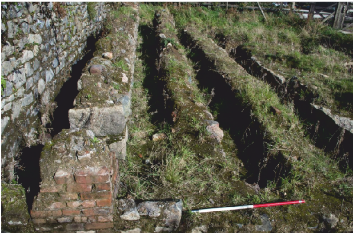
Fig 9 The retaining wall, left, and labyrinth (facing northeast).
