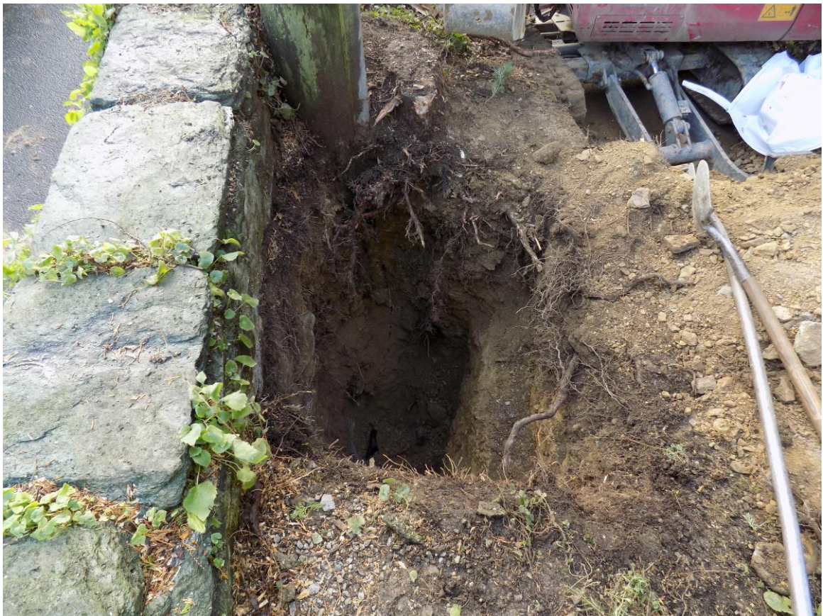
Figure 3. Pit 1 showing excavated section.
