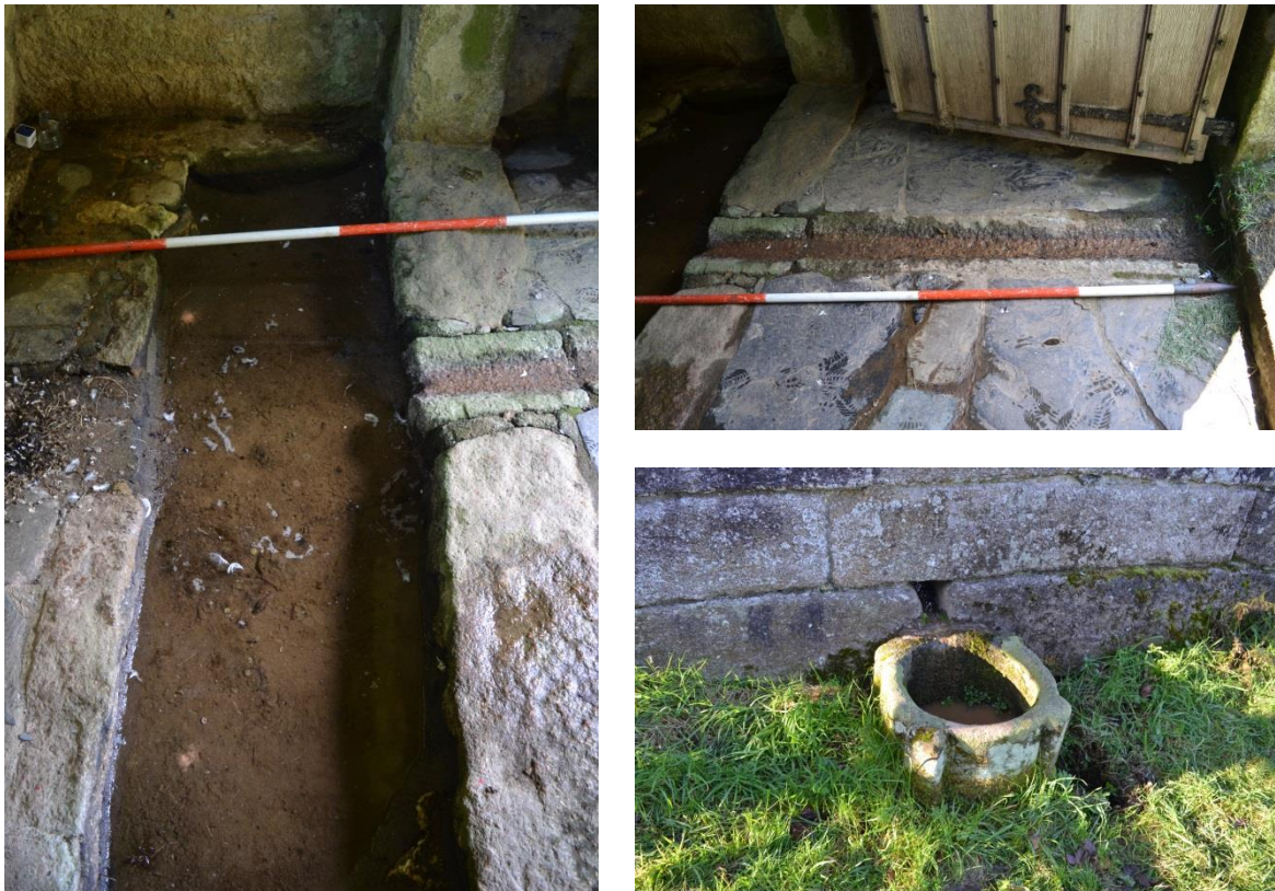
Fig 7. Visible features of the passage of spring water through the well-house. Left, the main trough or pool (before recent repointing). Top right, the granite launder conducting water across the well-house floor to the trough. Below right, the stone basin or mortar into which the water falls after exiting the well-house.
