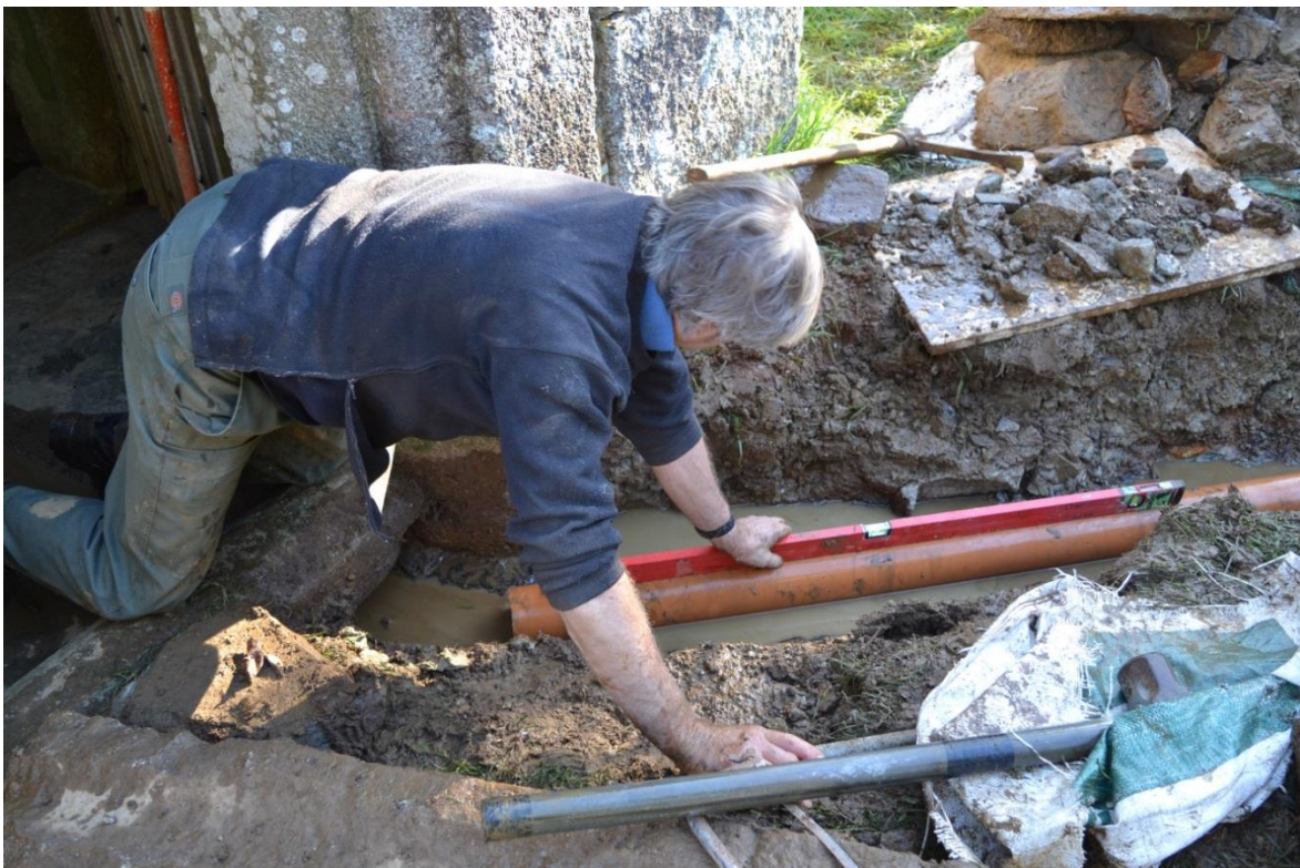
Fig 24. Peter Coombe, laying and levelling the new pipe.
