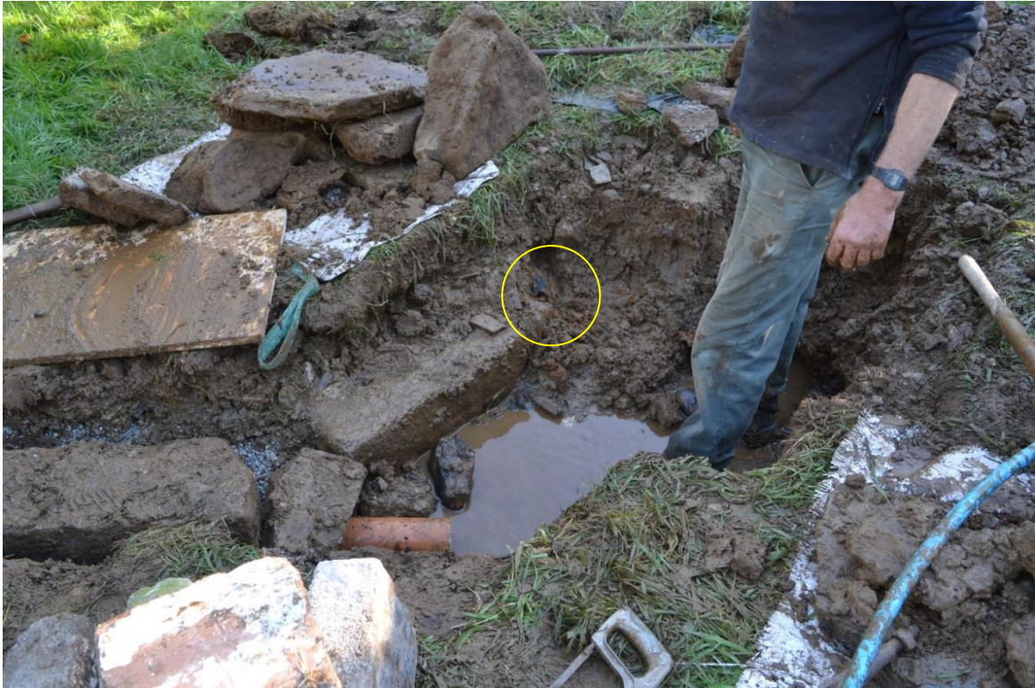
Fig 23. Iron pipe seen at a late stage, in the excavation on the east side of the 'chamber'. The pipe was black as a result of corrosion which had stained the surrounding ground red. The pipe had been previously cut through, presumably by earlier work on the chamber – it was not damaged during this project. The fall of the pipe (as far as we could ascertain) appeared to be from east to west and its purpose was uncertain.
