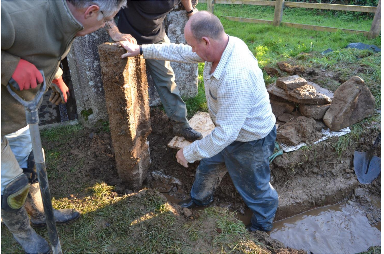
Fig 19. Lifting the granite launder.
