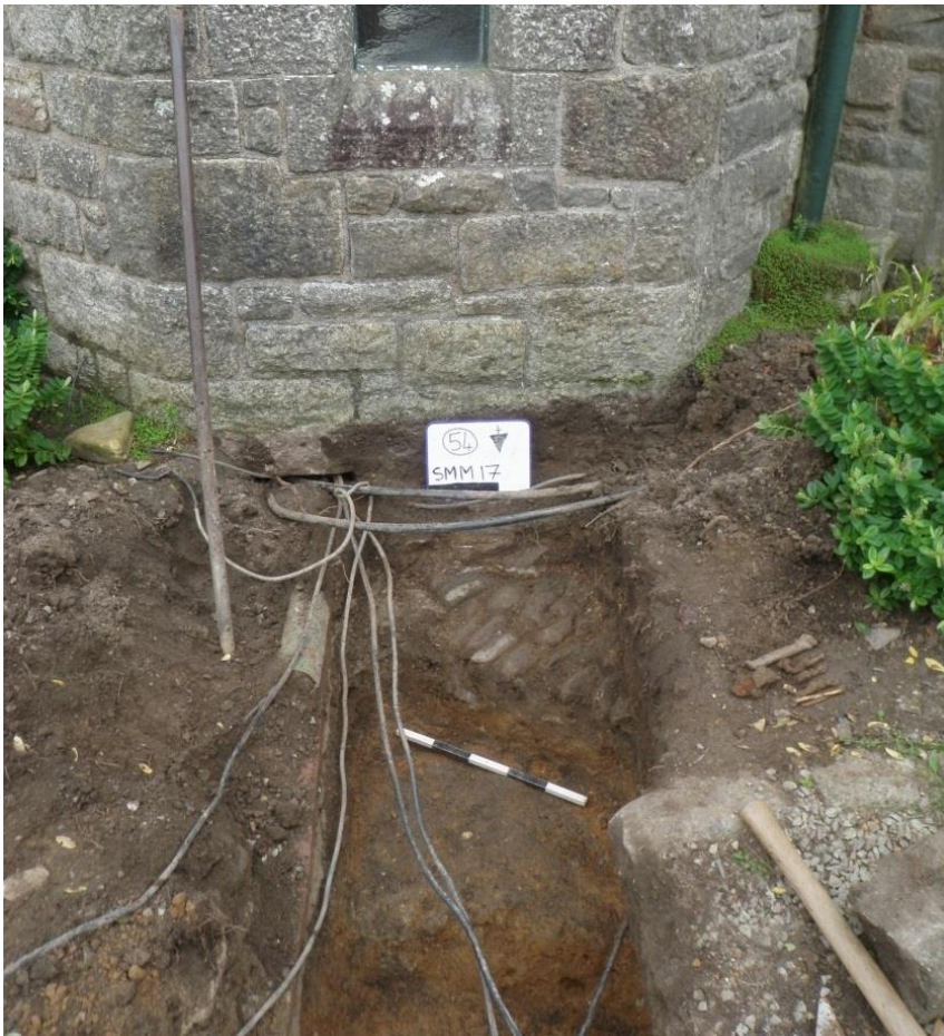
Fig 26 Looking south at the southern end of trench F/S showing cobbling (54).
