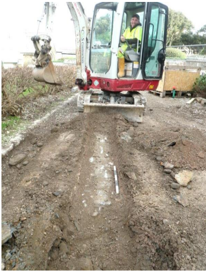
Fig 49 Looking east across the stone slab roof of culvert 155 (left) and along the emptied culvert (note fill (163) at the far end of the 0.5m scale).
