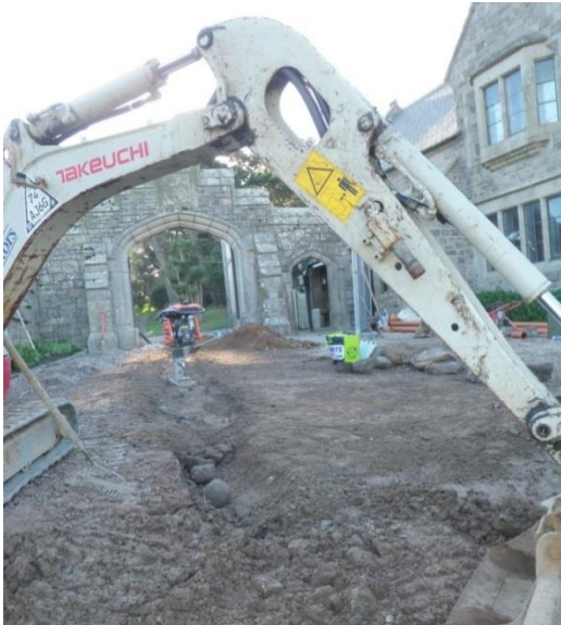
Fig 50 Looking south up largely backfilled trench J as it runs through the main gateway in to the gardens. Note the occasional cobbles in the back fill and the line of larger boulders beneath the arm of the digger, which come from wall 161.
