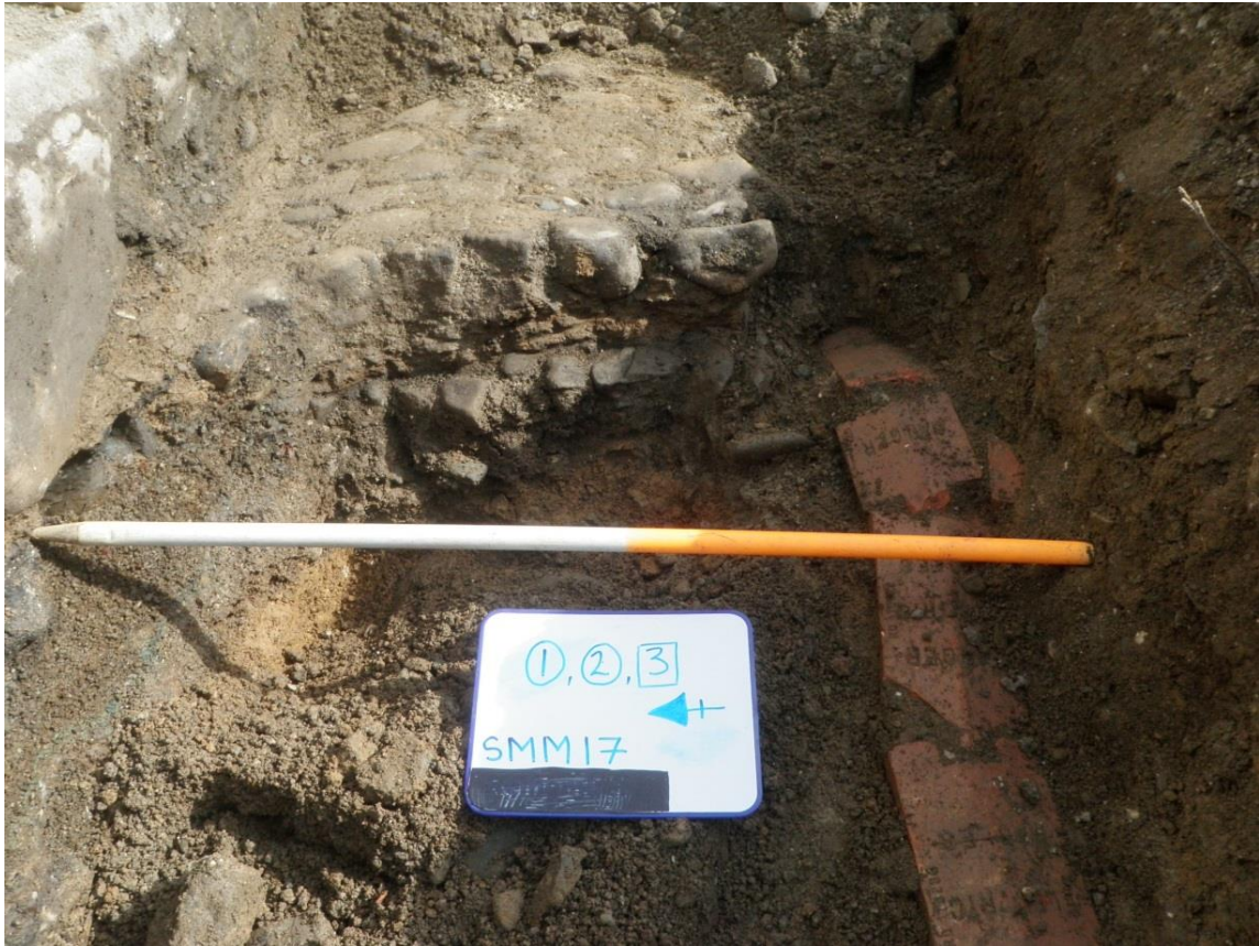
Fig 12 Looking east at upper cobbling (1), lower cobbling (2) and electrical cable tiles [3], with granite path sets (14) on upper left of photograph.
