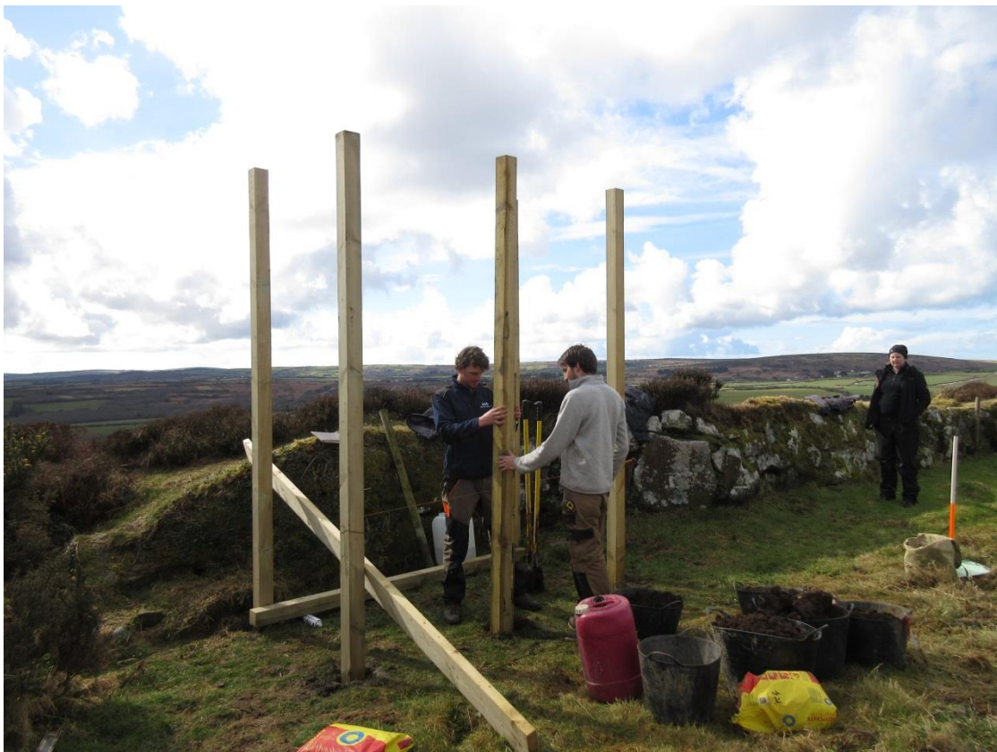
Fig 4. Construction of the framework for the viewing platform under way. The upright timbers had not, at this stage, been cut down to their final heights.
