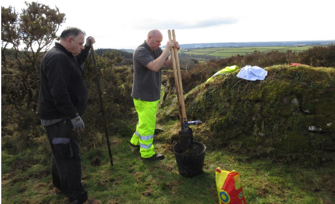
Fig 3. Contractors excavating the postholes and disposing of the arisings into buckets for subsequent inspection.
