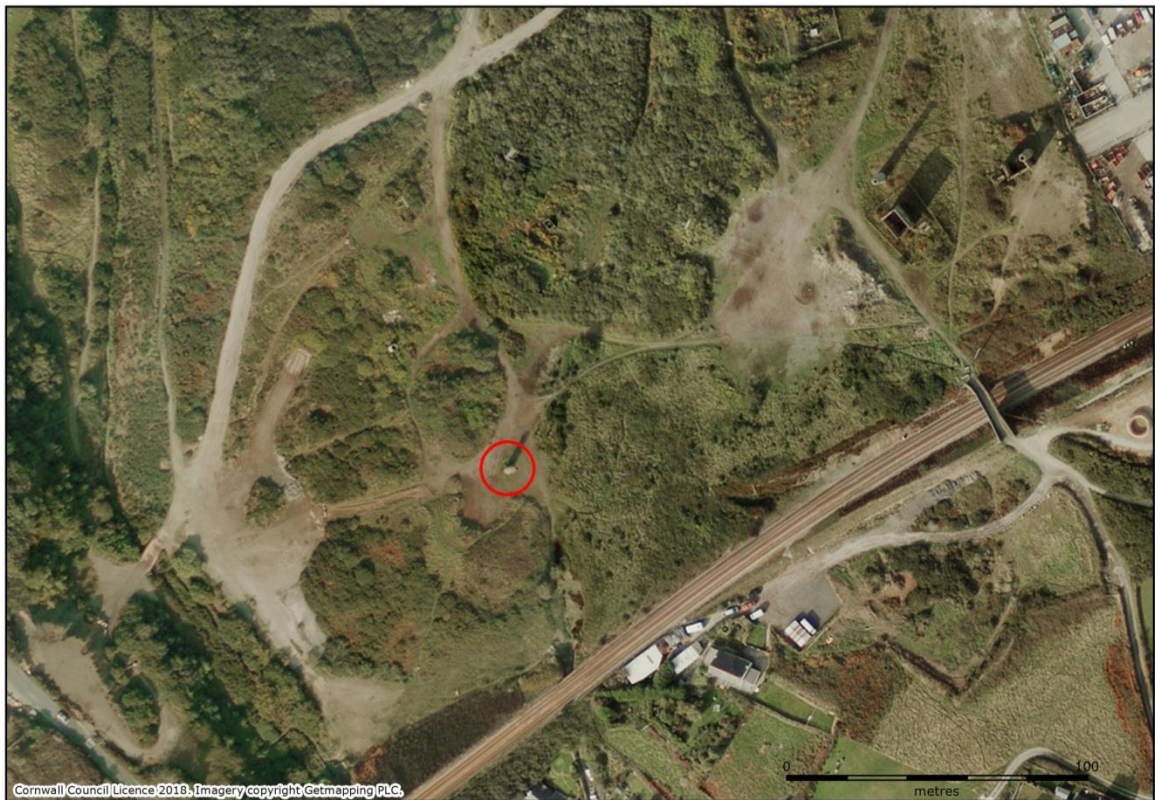
Fig 8. The situation of the Cook's Kitchen chimney in 2005.
