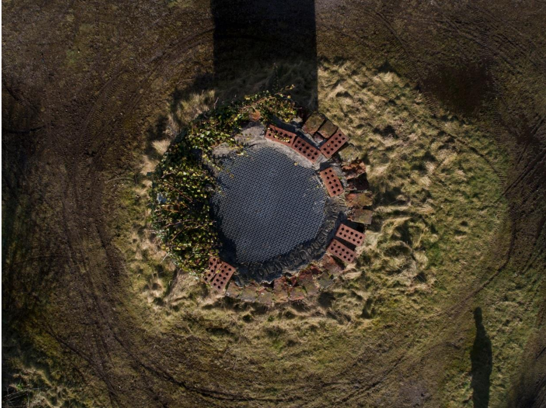
Fig 15. A vertical view of the chimney, showing the layers of galvanised mesh closing off its opening.
