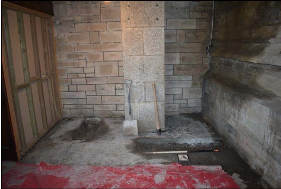
Figure 22: Trenches 2 and 1 prior to excavation. Looking north.
