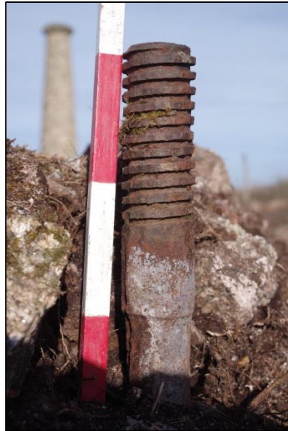
Figure 20: Threaded top of hold down bolt.
