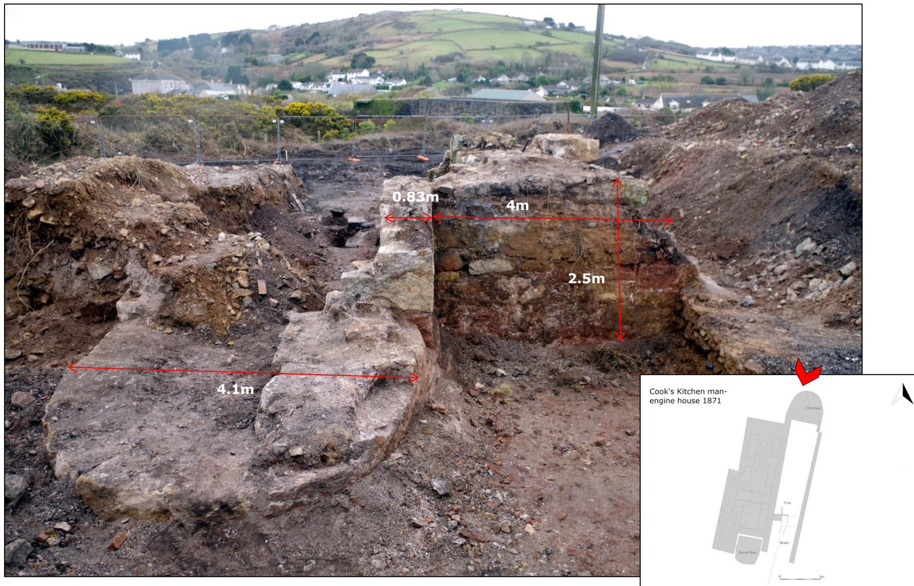
Figure 13: North elevation of man-engine house showing measurements. 30
