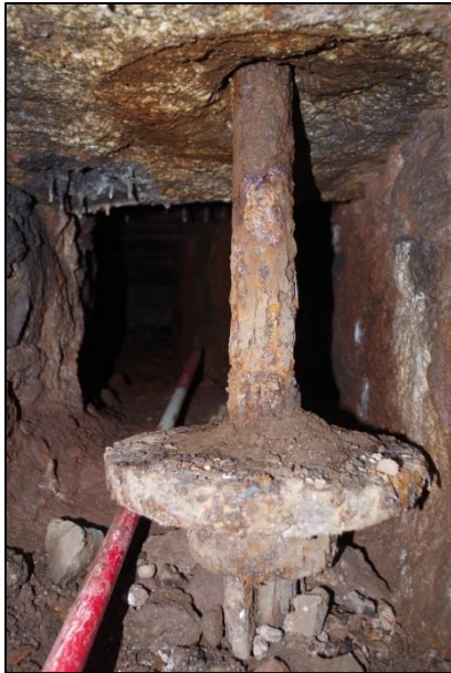
Figure 19: Bottom end of hold down bolt within crow hole.
