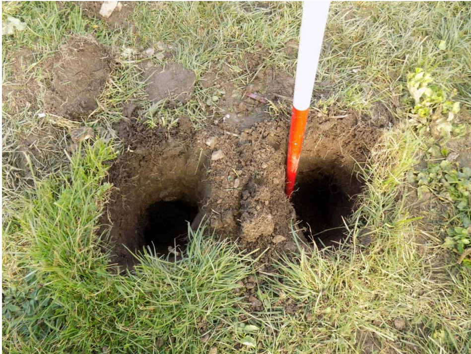
Figure 10. Panel 5, the postholes dug for the new panel.
