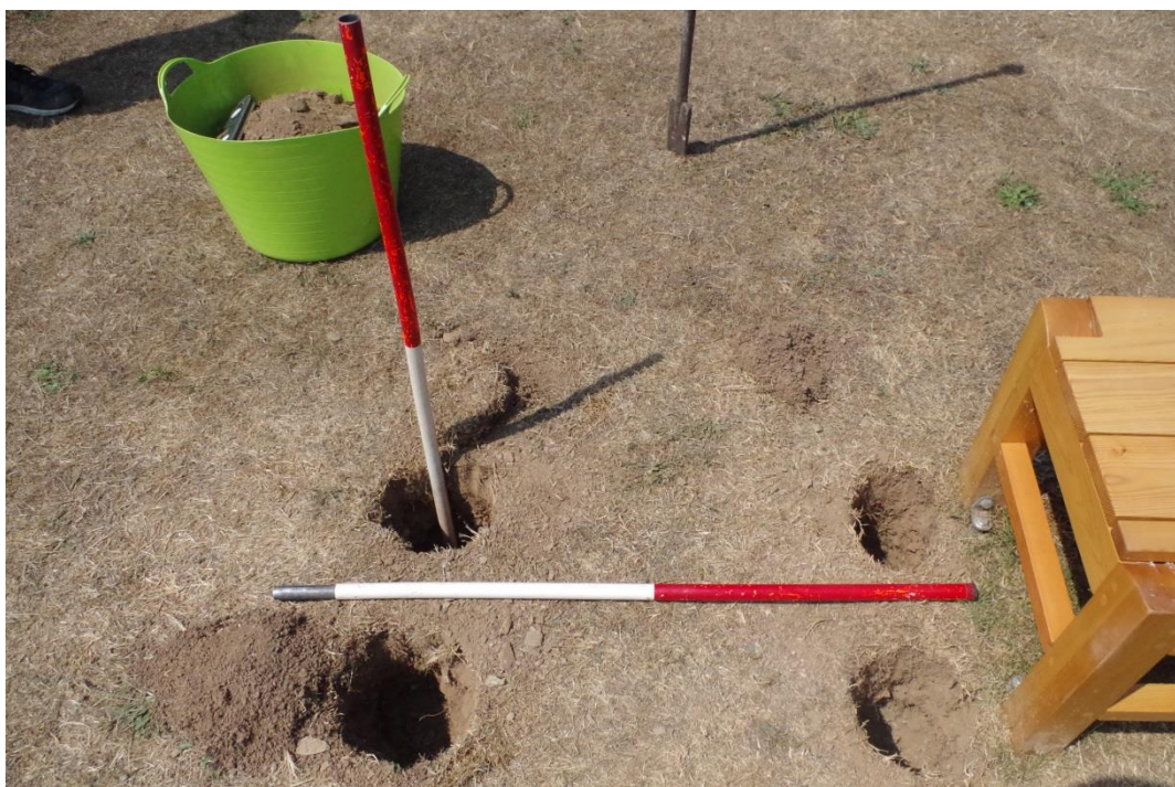
Figure 10. Panel 6. Postholes for the new panel.
