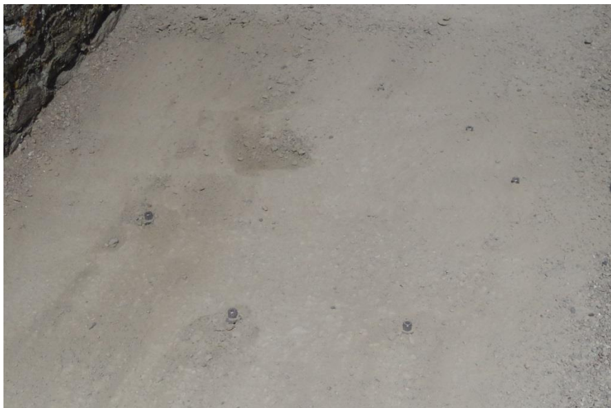
Figure 3. Panel 1. Corkscrew fixture bolts in position to hold support plate for panel showing minimal ground disturbance.
