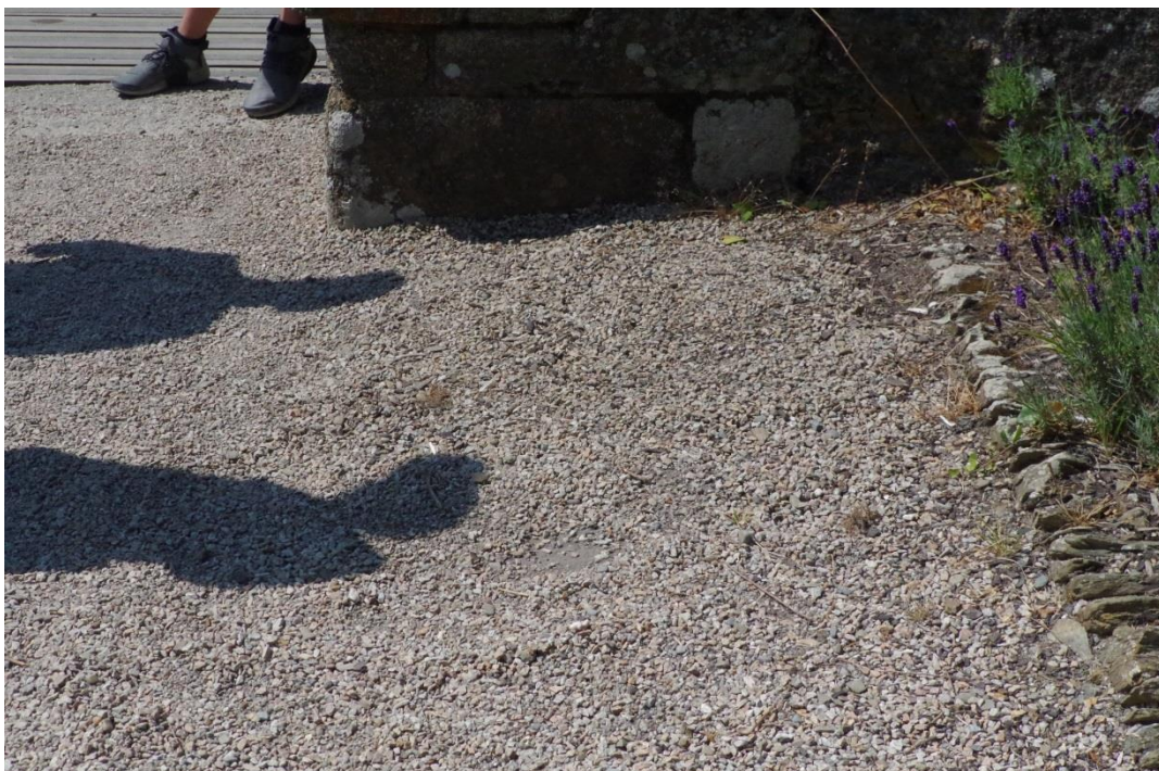
Figure 6. Panel 2. Location after the removal of the post.
