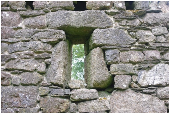
Fig 19 Interior of shippon, slit ventilator in north-west (rear) wall.
