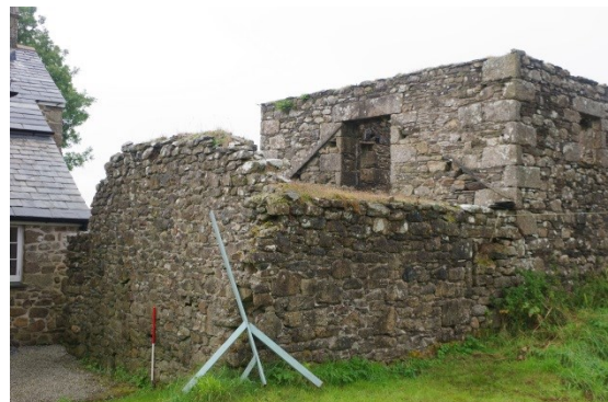
Fig 15 North-west and north-east elevations of threshing barn and shed/calf house.
