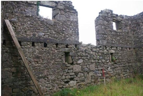
Fig 18 Interior of shippon and threshing barn, north-west (rear) wall.
