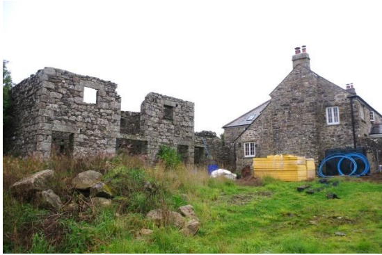
Fig 9 South-east (front) elevation of barn range.
