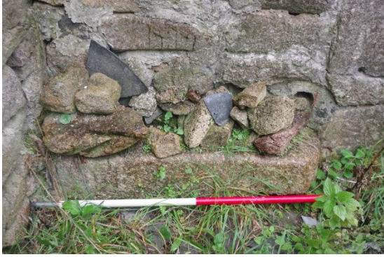
Fig 23 Interior of shed/calf house, step in blocked door opening in north-west (rear) wall.
