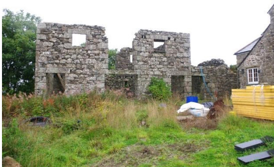
Fig 10 South-east (front) elevation of barn range.
