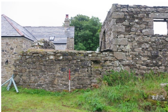
Fig 12 North-west (rear) elevation of shed/calf house.
