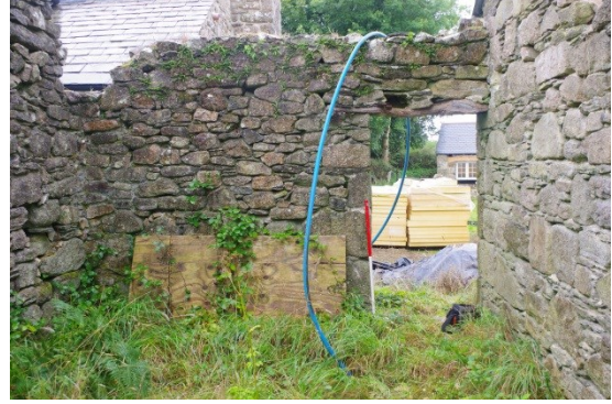
Fig 25 Interior of shed/calf house, south-east (front) wall.
