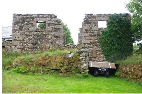
Fig 13 North-west (rear) elevation of shippon and threshing barn.
