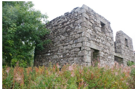
Fig 14 South-west elevation of shippon and threshing barn.
