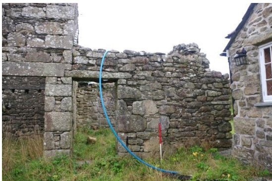
Fig 11 South-east (front) elevation of shed/calf house.
