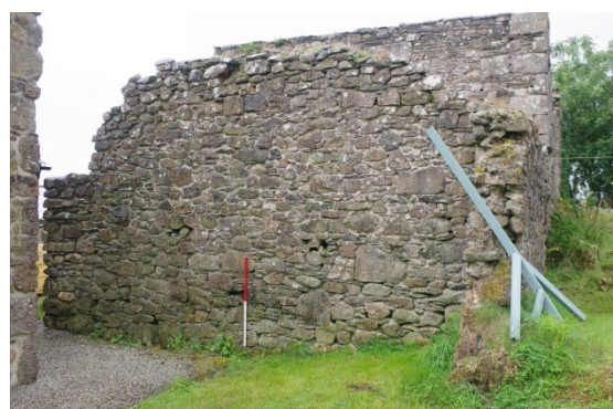
Fig 16 North-east elevation of shed/calf house.
