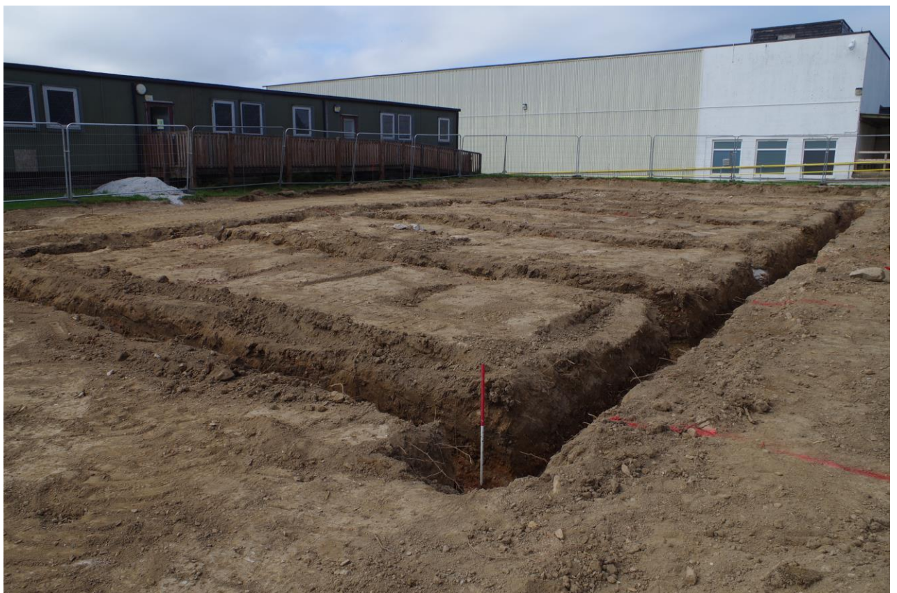
Fig 8 Site with foundation trenches excavated, seen from the southernmost corner.
