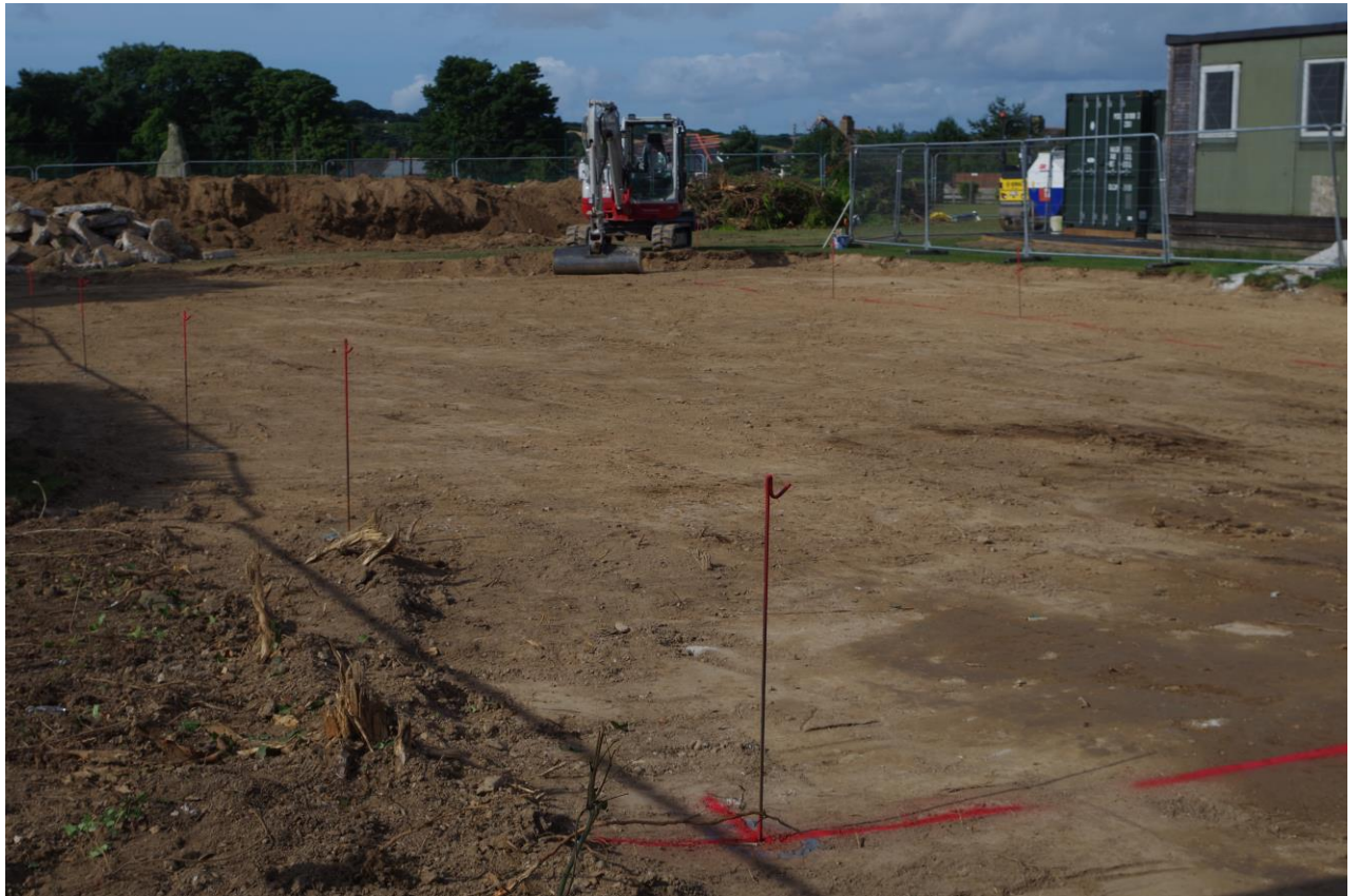
Fig 5 Site following topsoil strip, looking SSW. The Longstone is visible in the rear ground on the left, beyond the site fence.
