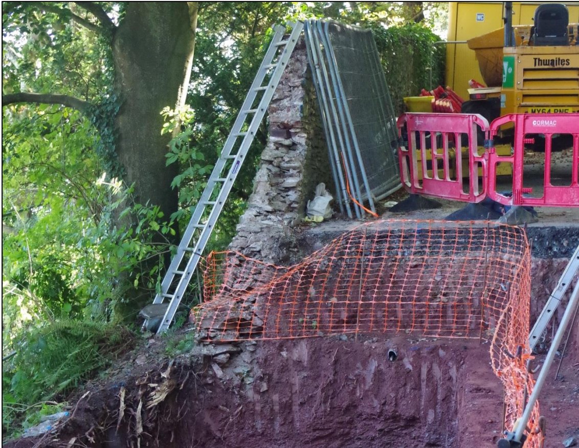
Figure 15. Detailed view of section A - B looking south east.
