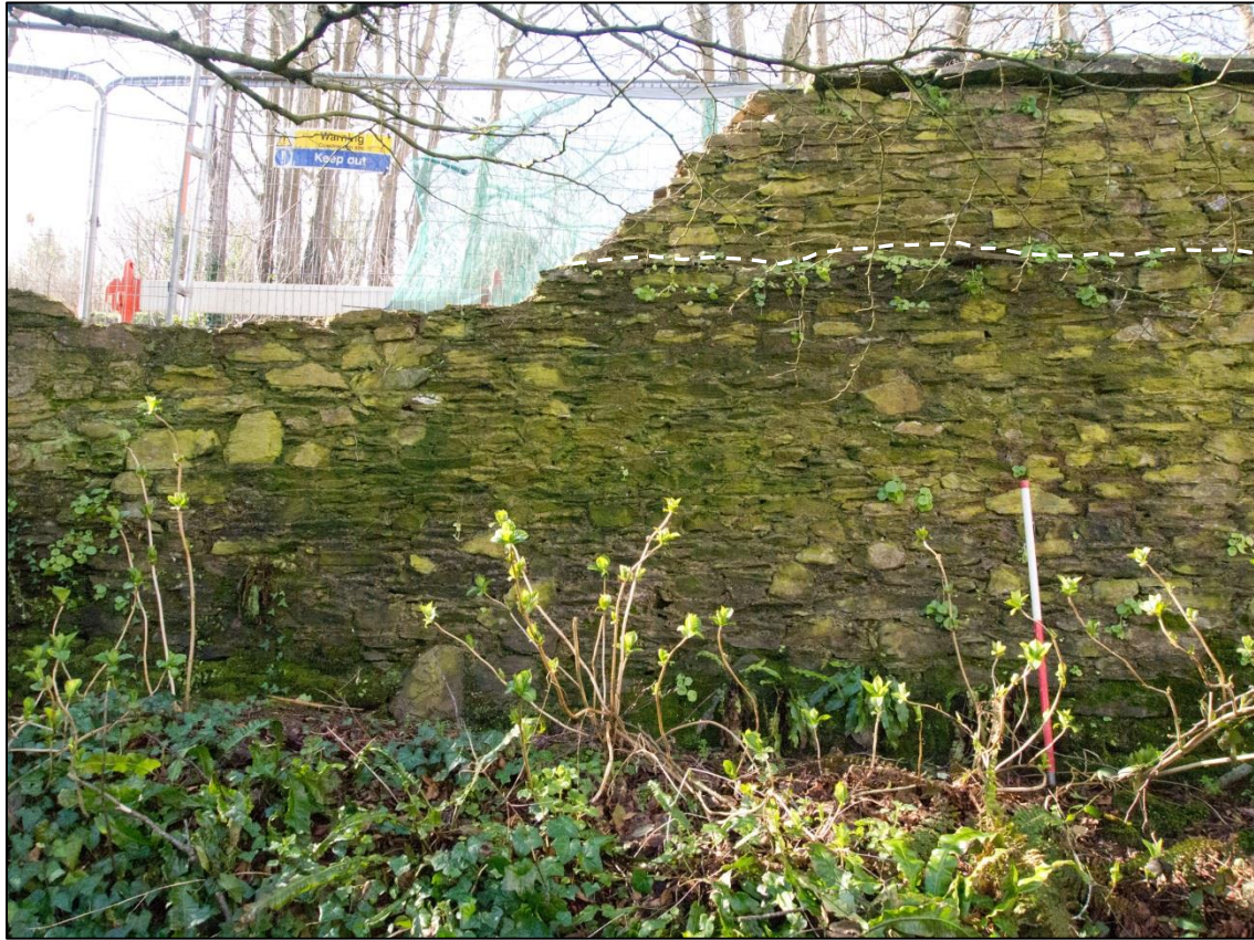
Figure 13. Eastern (The Woodlands) side. Detail close to damaged section of the boundary wall showing 'embankment' in foreground, and two construction phases to the wall.
